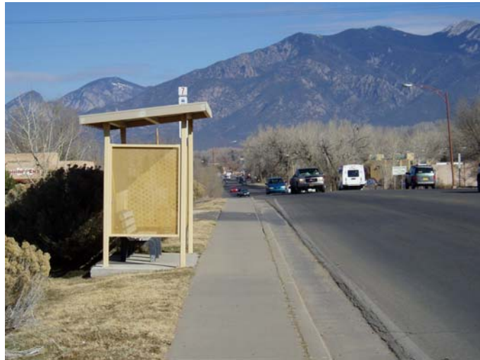
Figure 25: A Chili Line bus shelter
