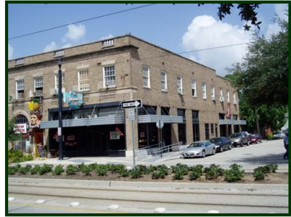
Figure C-12. Example of Missing Crosswalk
