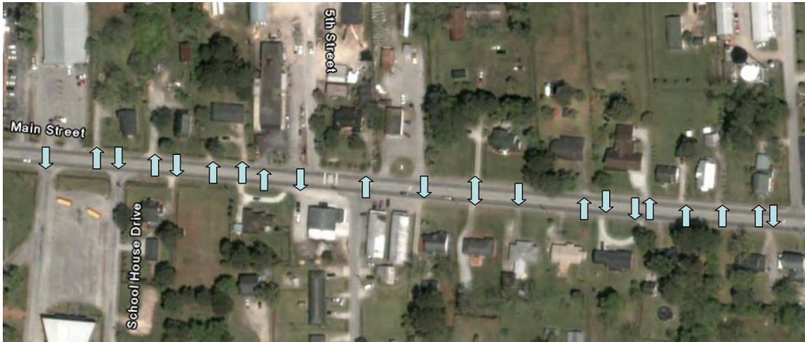
Figure 7. Aerial photo of Hwy 55 extending from Pamlico County High School to Fourth Street in the town of Bayboro. The arrows in this photo show twenty-two access points to Hwy 55 from commercial and residential properties for a 0.3-mile span. 12
