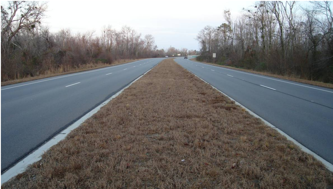
Figure 19. West of Columbia, NC, U.S. Highway 64 is designed as a “rural boulevard” and provides limited controlled access. 29
