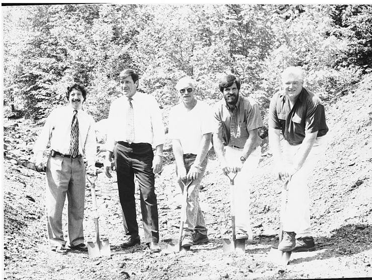
Ground breaking ceremony for the Green Run Reclamation Project in the Cheat River Watershed. Credit: Dave Bassage, Friends of the Cheat
