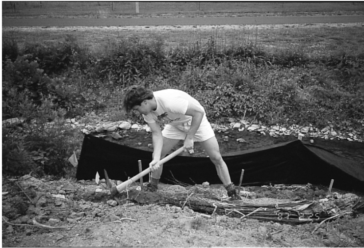
Save Our Streams volunteer digging a trench for a facine. Credit: Jay West.
