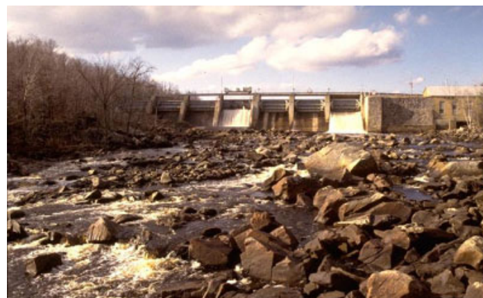
Grandfather Falls Dam, Wisconsin has had a visible effect on reducing flow volume and changing sediment characteristics downstream, with resultant changes in aquatic habitat quality.
