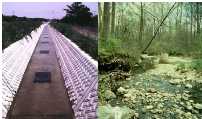
Urban channelized and "hardened" streams (left) are poor habitat but route stormflows quickly. Natural streams below urban areas (right) retain some habitat features but become heavily eroded by flows from increased urban runoff.
