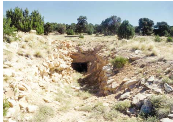
Figure 2. A typical trench portal leading to a uranium mine in western Colorado.
