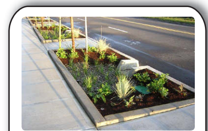
Portland's new stormwater marketplace should encourage more onsite stormwater features such as this planter. See article on page 6.
