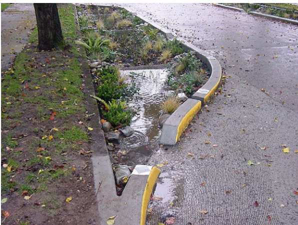
A landscaped curb extension on a Portland street improves aesthetics, calms traffic, and captures and infiltrates runoff from the street.
