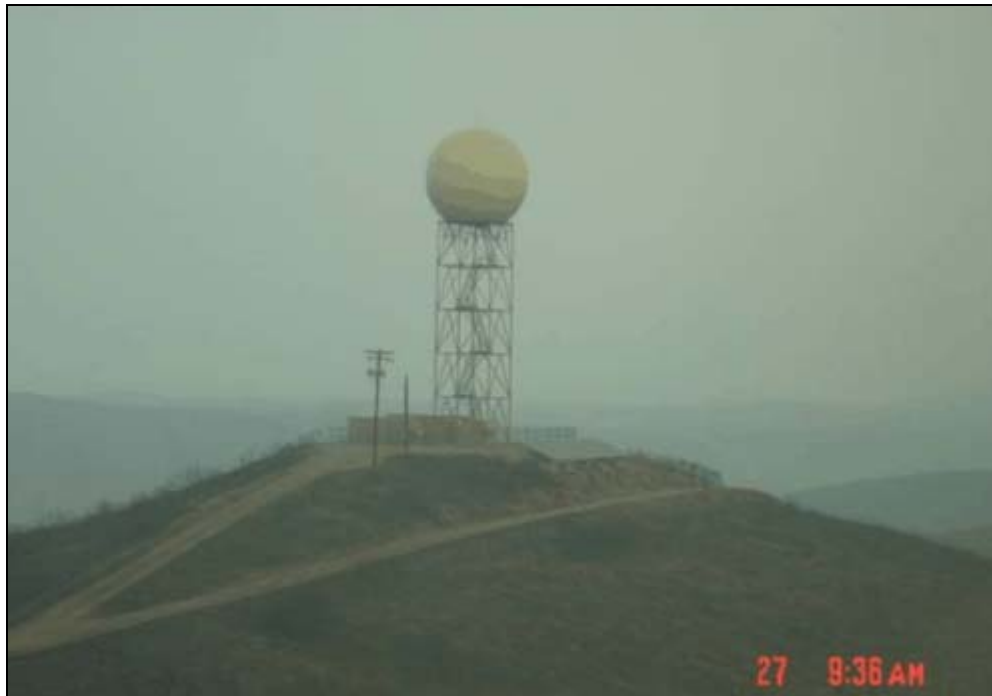
Picture 4. WFO San Diego's WSR-88D facility after the firestorm. Courtesy of WFO San Diego.
