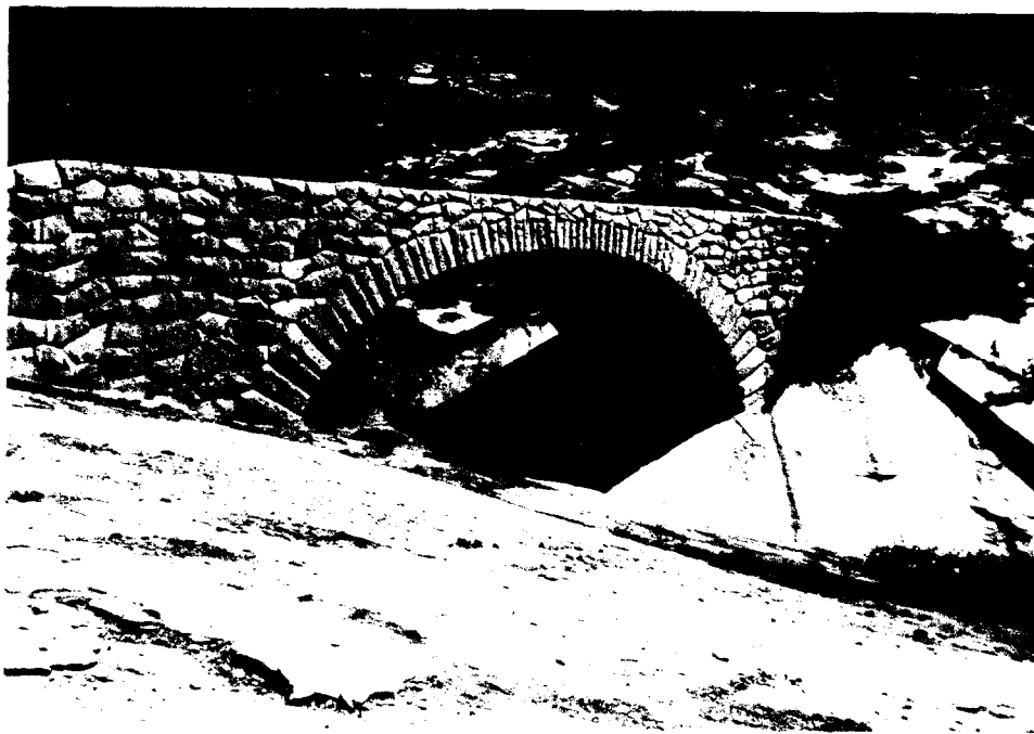
Photograph No. 79 -- Clover Creek Bridge; downstream side
