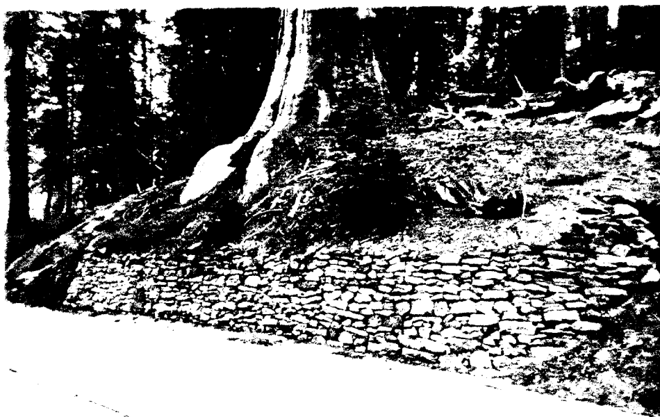
Photograph No. 70 -- Loose rock retaining wall along upslope side of highway to protect Sequoia tree (1.9 miles above Giant Forest Market)
