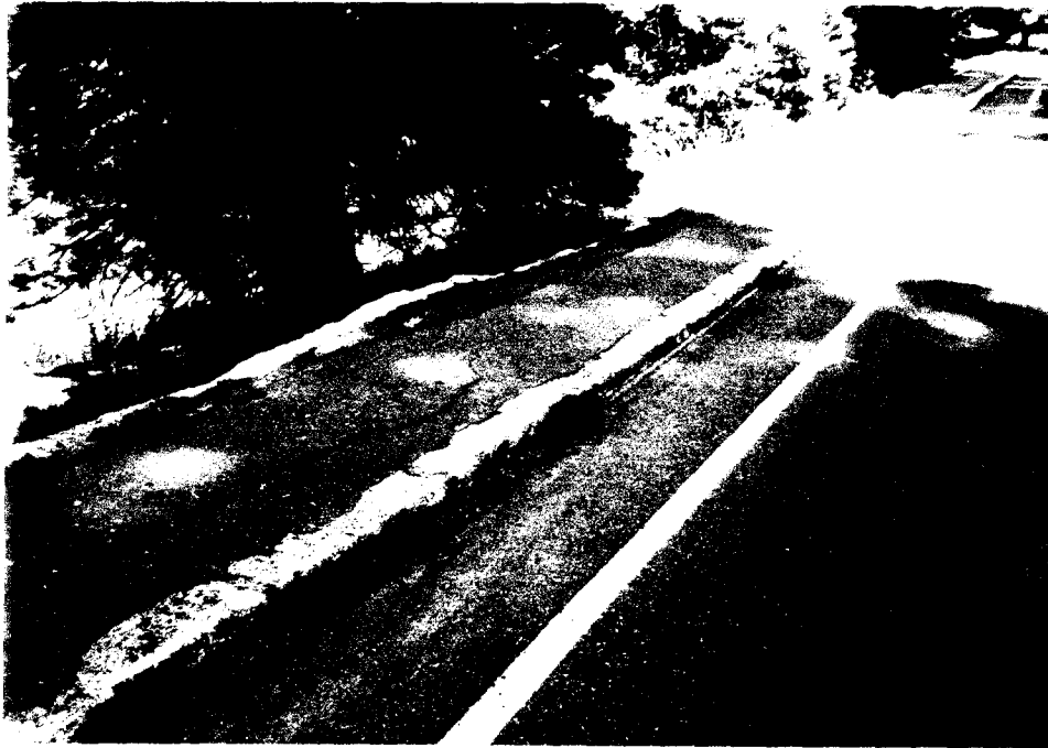
Photograph No. 5 -- Blacktop walk between cut stone curbing along highway just above Giant Forest Market Plaza
