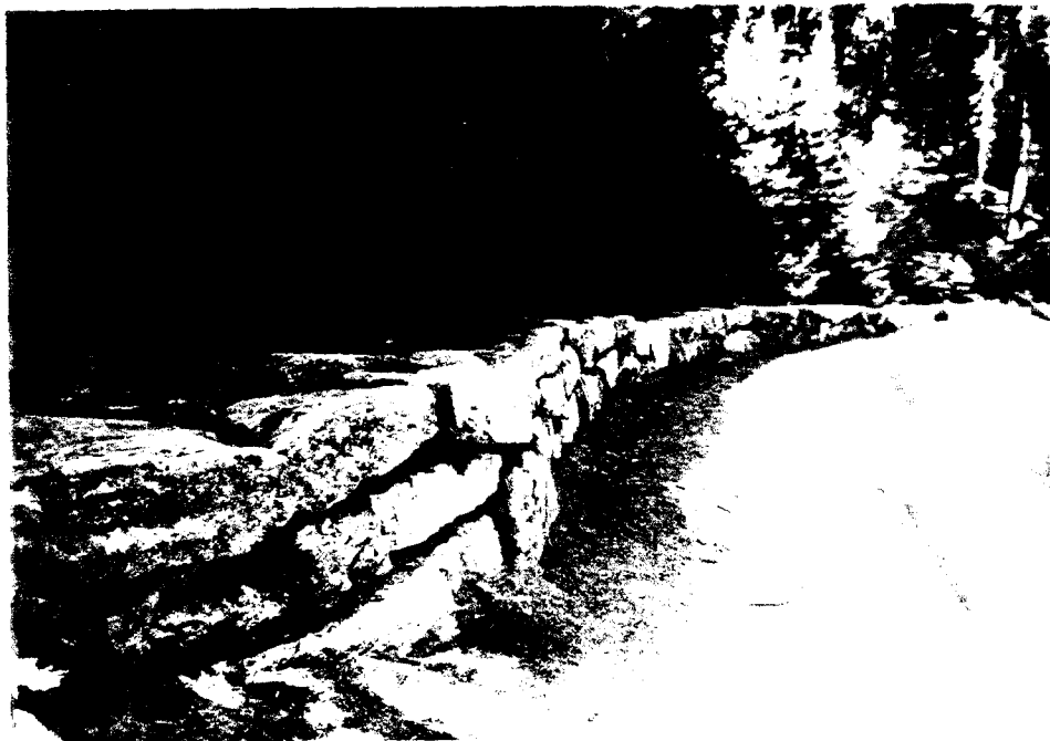
Photograph No. 10 -- Longest example of low granite retaining wall along highway; on upslope side just below Wall Spring (0.9 mile below Giant Forest Market)
