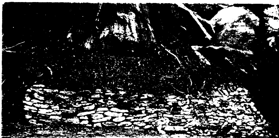
Photograph No. 58 -- Stone retaining wall along upslope side of highway to protect Sequoia tree (1.8 miles above Giant Forest Market)
