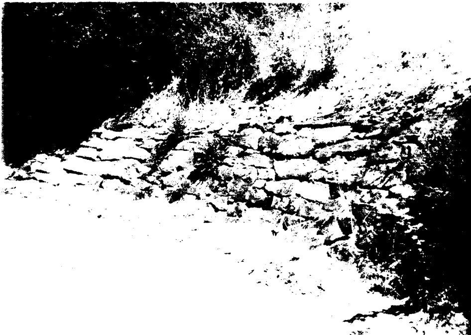
Photograph No. 27 -- Sloping retaining wall along upslope side of highway just above Black Oak Corner (6.5 miles below Giant Forest Market)
