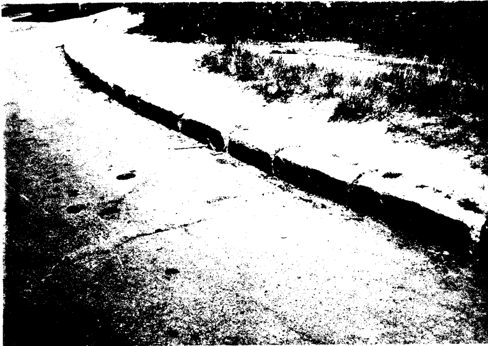
Photograph No. 1 -- Cut stone curbing around parking lot at Grant Forest Market Plaza
