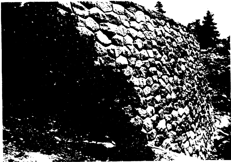
Photograph No. 94 -- Masonry retaining wall which is topped by Photograph No. 93
