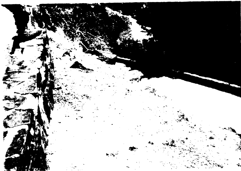
Photograph No. 26 -- Amphitheater Point overlook parapet wall at left; parapet forms top of stone retaining wall on upslope side of highway below; parapet wall along downslope side of highway below at right (5.55 miles below Giant Forest Market)
