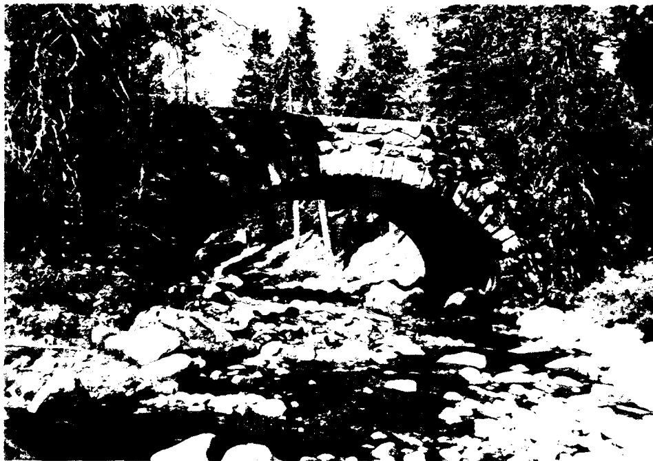
Photograph No. 75 -- Stone bridge over Marble Fork of Kaweah River looking upstream
