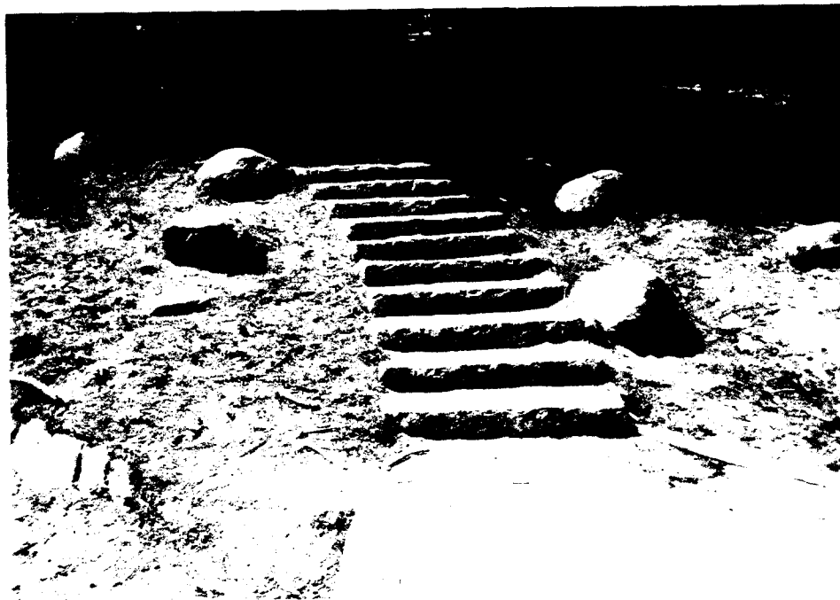
Photograph No. 4 -- Cut stone steps leading from highway toward Camp Kaweah Motel area
