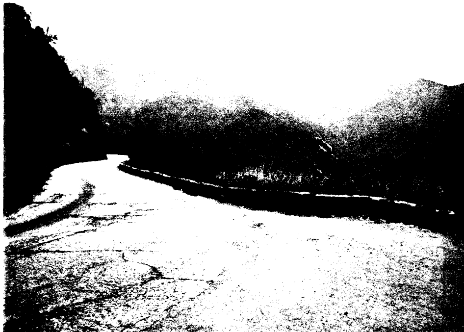
Photograph No. 15 -- Parapet rock wall at Deer Ridge overlook and along downslope side of highway below turnout (4.0 miles below Giant Forest Market)
