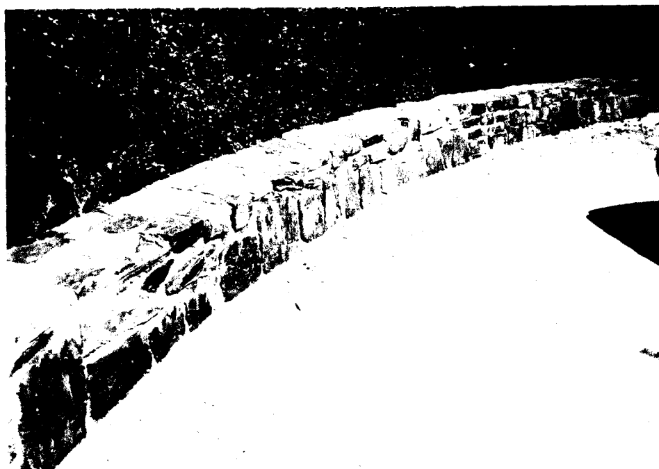
Photograph No. 16 -- Parapet rock wall at Deer Ridge overlook on downslope side of highway (4.0 miles below Giant Forest Market)
