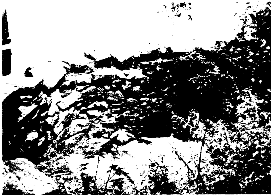
Photograph No. 31 -- Big Fern Spring rock work on upslope side of highway with culvert to carry spring water under road (6.95 miles below Giant Forest Market)
