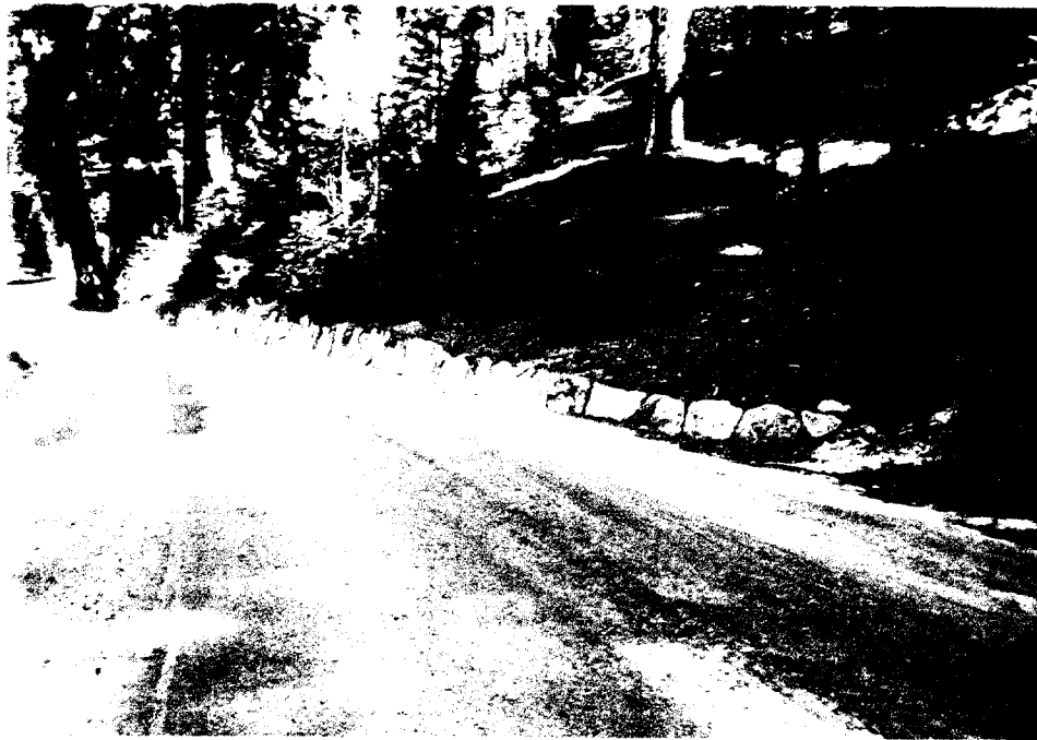
Photograph No. 7 -- Stone retaining wall along highway just above Giant Forest Market Plaza
