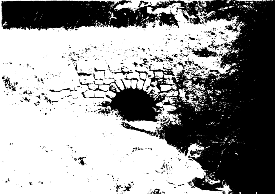
Photograph No. 33 -- Double stone culvert headwalls on S-curve along highway (7.95 miles below Giant Forest Market)
