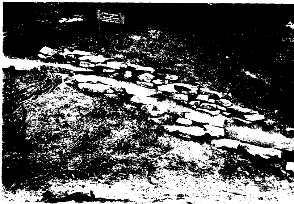
Photograph No. 86 -- Rock-lined Little Baldy trail head along upslope side of highway
