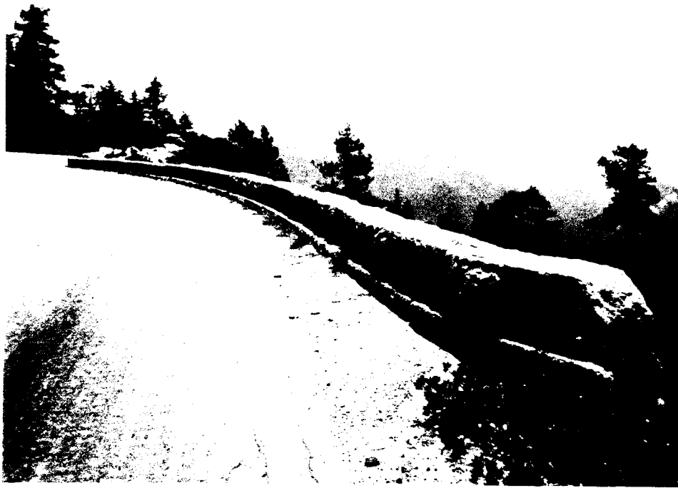
Photograph No. 93 -- Masonry parapet wall along downslope side of highway just above Redwood Mountain Grove turnout
