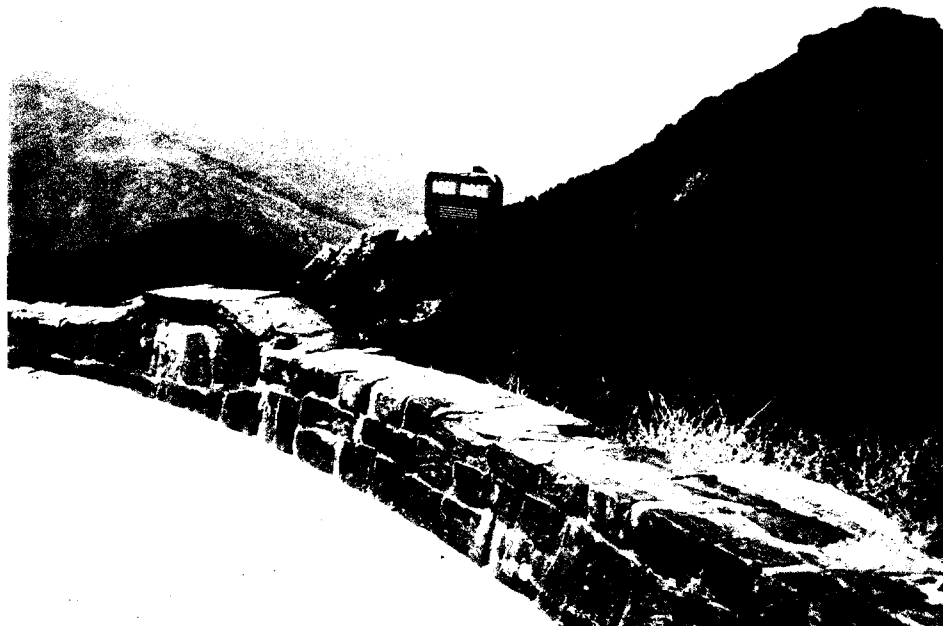
Photograph No. 14 -- Deer Ridge overlook parapet rock wall on downslope side of highway; uppermost turnout of rustic design (4.0 miles below Giant Forest Market)
