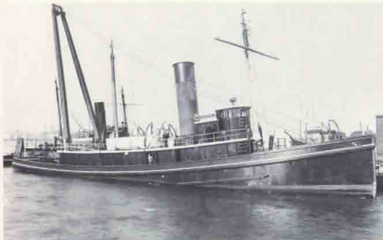
Fig. 3. HERCULES and her sister vessel GOLIAH (obscured by large sheerlegs behind aft end of HERCULES' deckhouse) at their builder's yard in 1907. Square yards and staymasts are rigged for the long voyage to the West Coast.
