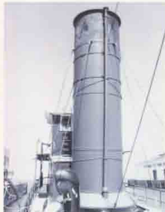
Fig. 25. The smoke stack as viewed from aft. The stack has been rebuilt at least once during HERCULES' working life, as evidenced by a combination of welded and riveted construction, but retains its original form. The tall stack is a significant feature of steam tugs.
