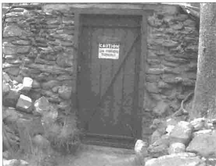
Contemporary view of the food locker (HS-3). Built into the slope, this structure is believed to have been constructed in 1900 as a cold food storage facility. View looking southwest. Photo, 2003. (National Park Service)
