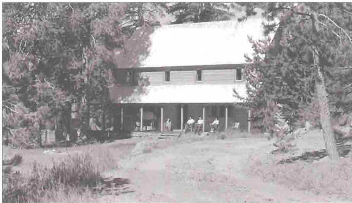
The early path of the Warner Valley Road routed it just east of the lodge. Photo, 1939. (LAVO Collection, B-1028-1)
