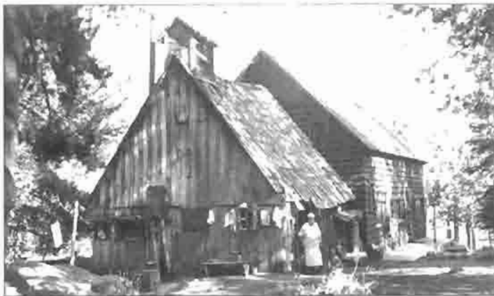
View looking south toward the kitchen and dining room. Photo, circa 1941. (LAVO Collection, DB79)
