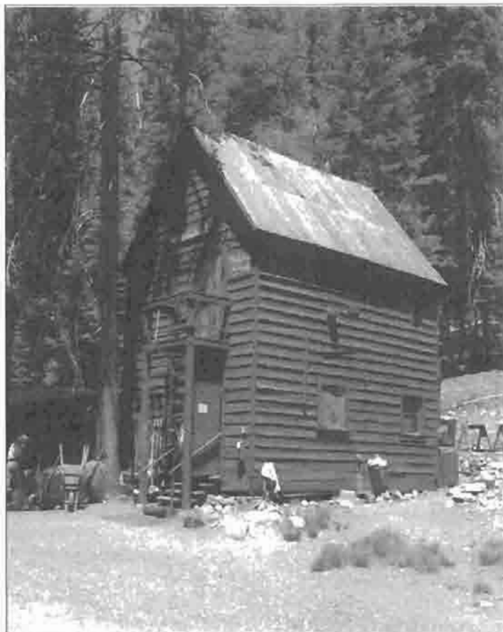
Contemporary view looking northwest at the storage building, more commonly known as the Hilton. The upstairs is used as housing for concession staff, and the main floor is used as a laundry room and storage area. Photo, 2003. (National Park Service)
