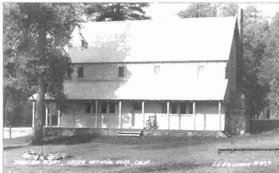
Photograph showing the porch along the east façade of the new lodge building, rebuilt by the Sifford's in 1938 after a winter snow storm that demolished the original lodge. Photo, 1938. (LAVO Collection, DB26)
