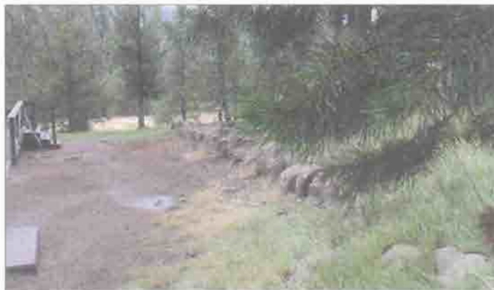
West of the lodge a single-course, dry-laid retaining wall separates the parking lot from the lawn area. Photo, 2003. (National Park Service)
