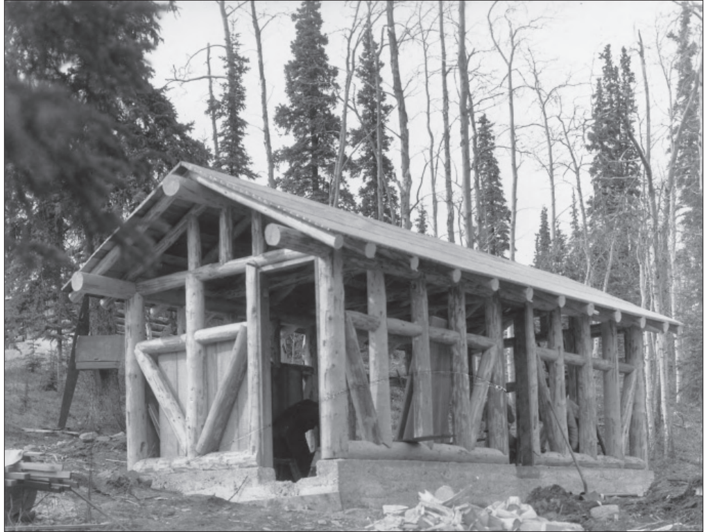
Figure 1.28. View northwest of the comfort station (Building 112) during construction. Photographed by Joseph S. Dixon, Field Naturalist for the NPS, May 29, 1932 (DENA-69-3-43, Harpers Ferry Center).
