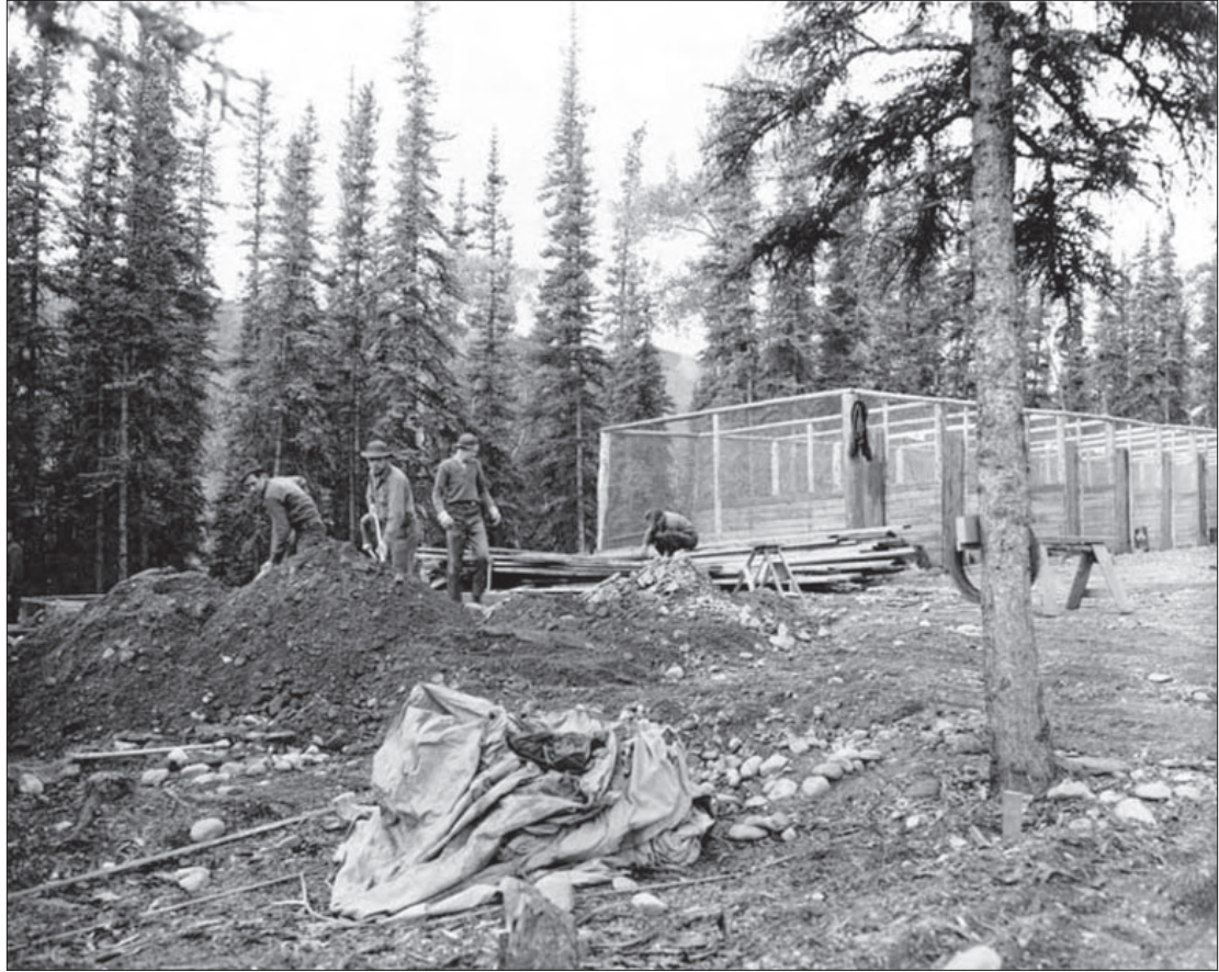
Figure 1.36. View southwest of CCC crew reconstructing the dog feed cache and cookhouse (Building 105), August 1938 (Ickes Collection, B75-175-295, Anchorage Museum of History & Art).
