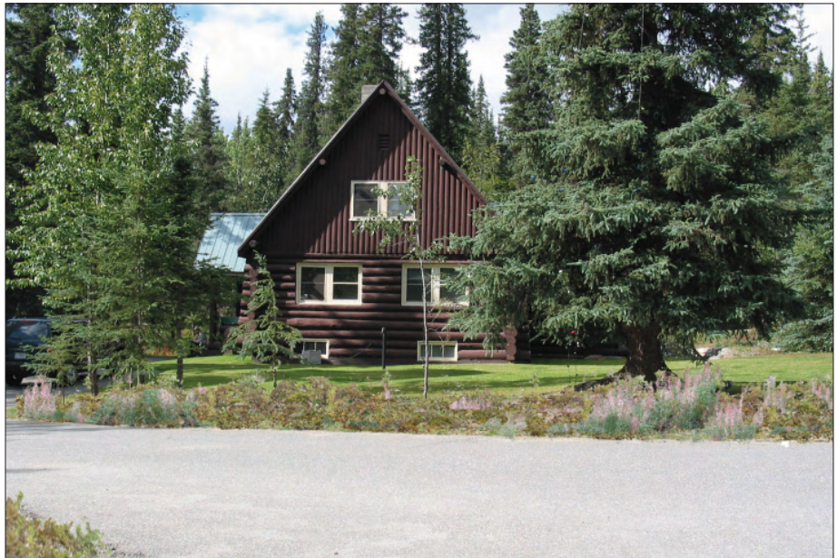
Figure 4.25. Circulation and Parking - Enhance Roadside Character and Vegetation - Treatment Task 2.F - Establish an eight-foot-wide buffer of native vegetation between the edges of headquarters roads and areas of managed turf. By establishing an eight foot wide buffer of native annual and herbaceous plants where areas of lawn meet the Headquarters roadways, popular areas of turf grass may be retained while enhancing the historic character of the property. These narrow buffers may be economically established over time by simply limiting mowing to once per year, timed to coincide with the end of each growing season (OCLP, 2007).
