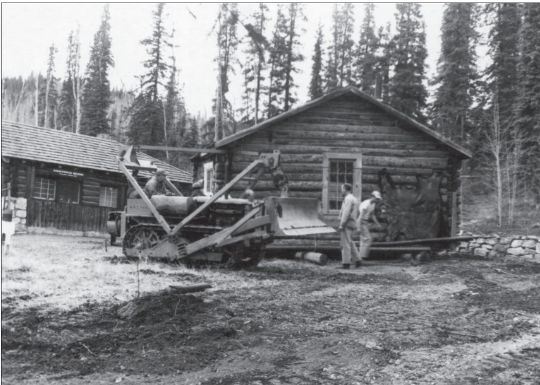
Figure 1.64. View northwest during relocation of the log naturalist's office and workshop (Building 22, original superintendent's office), June 1952. Note the animal hide attached to the side of the building, the administration building (left, Building 111, original superintendent's office) and the stone retaining wall (right, Building 111A) (National Archives and Records Administration, College Park, MD).
