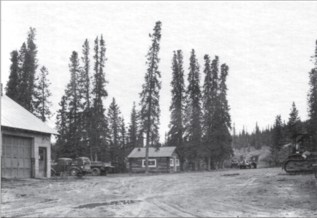
Figure 1.63. View of the former log park museum (Building 22, original superintendent's office), September 12, 1950, several months after it was relocated to the service area for use as a construction office. This building subsequently became the park naturalist's office and workshop. Also depicted is the machine shop and garage (Building 102, left) and the unpaved service road (DENA 3-18, Denali National Park and Preserve Museum Collection).
