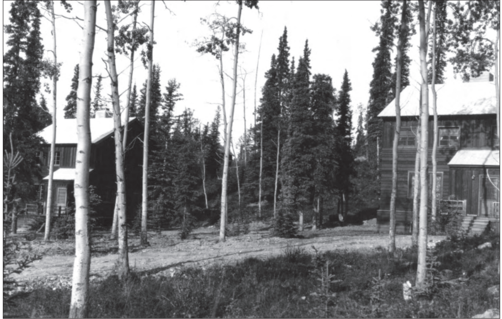
Figure 3.20. View west of vegetation surrounding Building 12 (right) and Building 13 (left), August 16, 1939. Note the mature spruce and poplars, the young spruce planted by the CCC in 1939. Also note the earthen driveway leading to Building 12 (Alaska Regional Office, Regional Cultural Resources Files).
