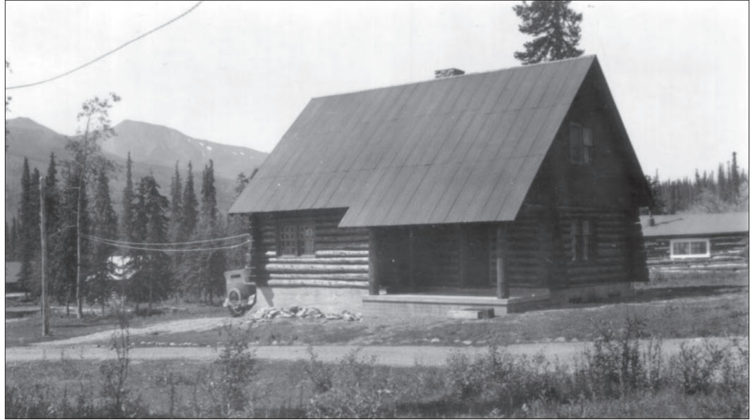
Figure 1.30. View southwest of the employee's quarters, c. 1935. The main headquarters road is in the foreground and the original clerk's cabin is to the right. Note the laborers' quarters (right, original clerk's quarters built in 1925) utility lines and the stones bordering the road. The two buildings to the left may be the garage (far left, Building 103) and the laborers' quarters (Building 6) (National Archives and Records Administration, College Park, MD).
