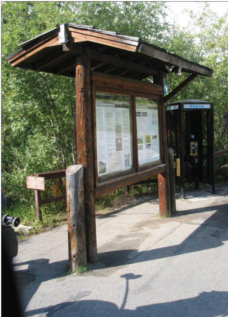
Figure 2.14. Visitor kiosk at parking lot near entrance to park headquarters with display panels capped by a small roof (August 2005, OCLP).
