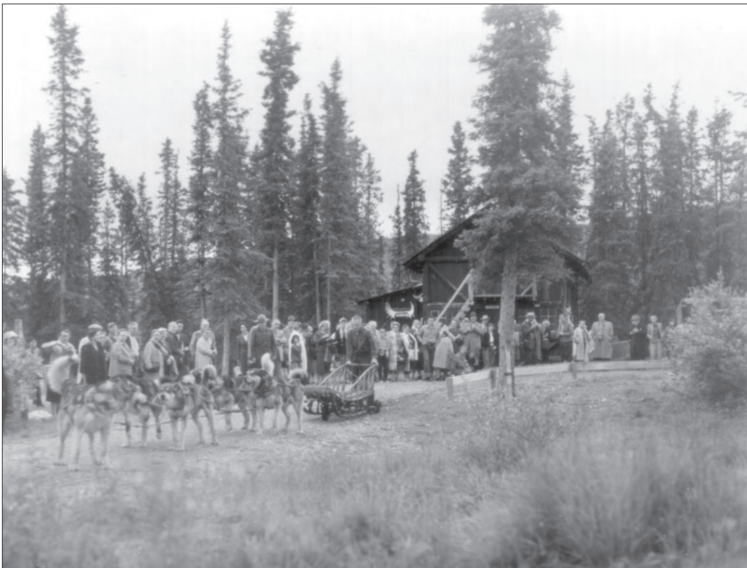
Figure 1.71. View southeast of a sled dog demonstration, July 11, 1959. The start of the sled dog demonstration trail is to the left, just outside the photograph. The dog feed cache and cookhouse (Building 105) is in the background (DENA 11-60, Denali National Park and Preserve Museum Collection).
