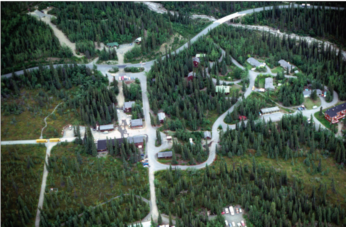
Figure 1.73. Oblique aerial photograph of Denali National Park & Preserve headquarters area on 8/24/1982 showing ground disturbance of the utility corridor leading to the water reservoir. NPS, Denali Resource Management slide file.
