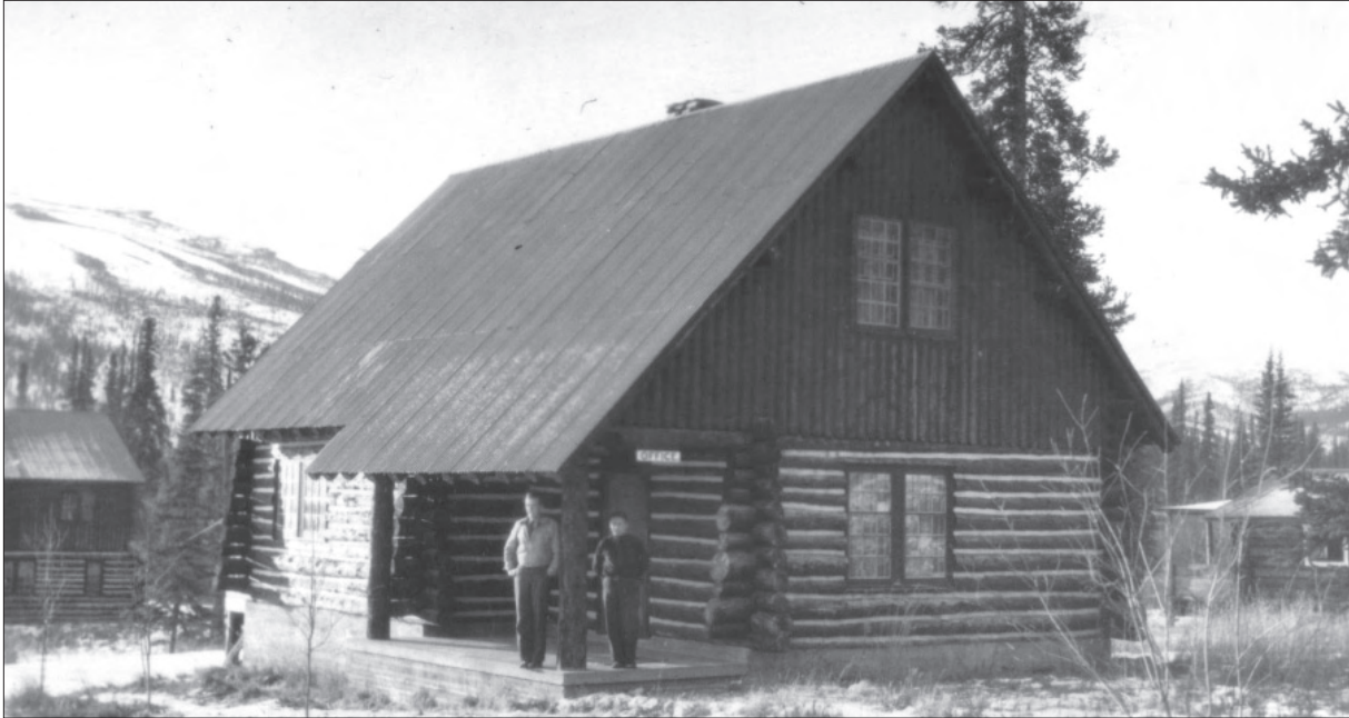
Figure 1.53. View southwest of the administration building (Building 11, original employee's quarters) from the main headquarters road. Also depicted is the rangers' dorm (Building 21, left), and employee's quarters (original clerk's cabin, Building 3, right), November 1940 (NPS, Alaska Regional Office files).
