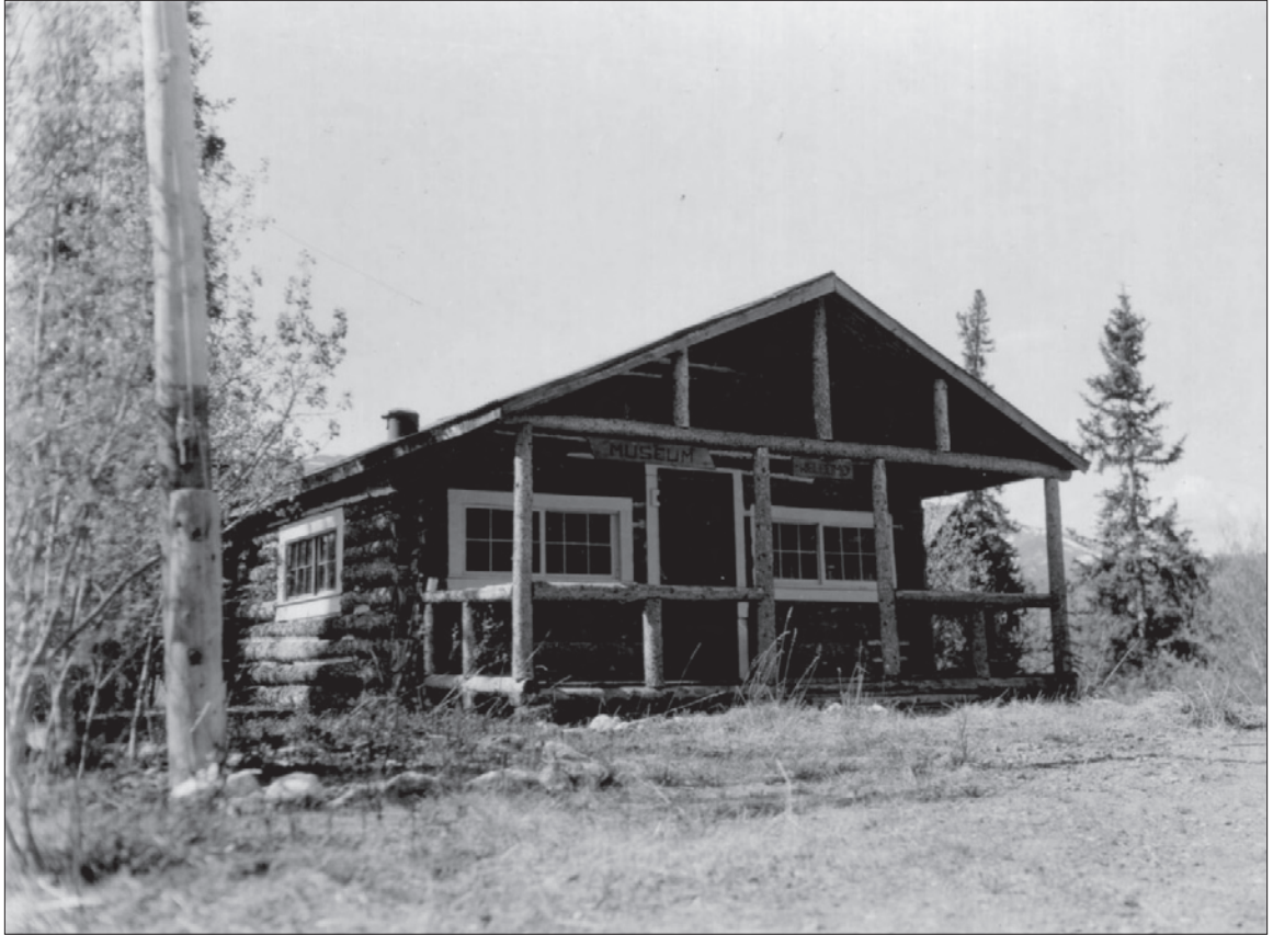
Figure 3.28. View southwest of the flag pole east of Building 22 (original superintendent's office), June 1946 (DENA 5-2, Denali National Park and Preserve Museum Collection).
