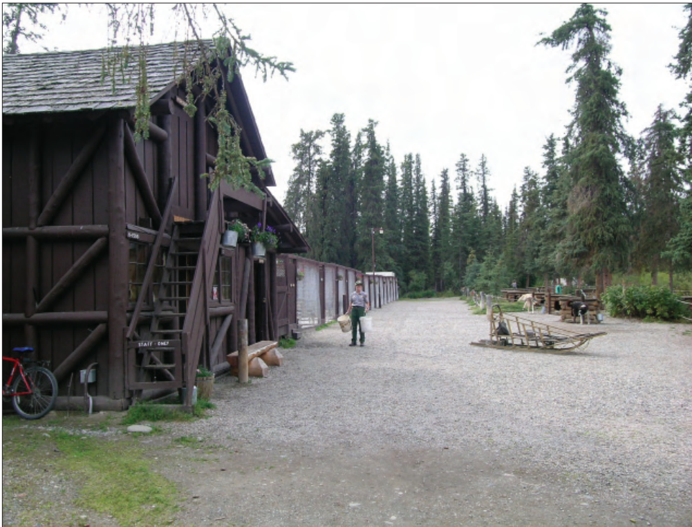
Figure 2.11. Building 105, Dog Feed Cache and Sled Storage, and the dog kennels are a popular destination for park visitors (August 2005, OCLP).
