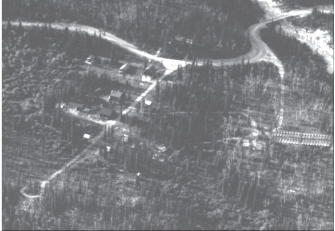
Figure 1.34. Oblique 1935 aerial photograph of park headquarters area. Note the unimproved quality of roads in the eastern half of the headquarters area. Also note the wagon-turn at the terminus of the north-south headquarters road (DENA 3906, Lincoln Washburn photograph, Denali National Park and Preserve Museum Collection).
