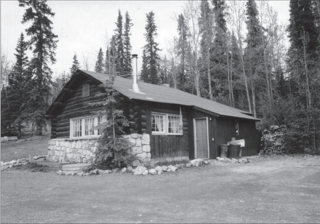
Figure 1.72. View northwest of employee's residence (Building 111) after conversion into a year-round residence, June 1984. (NPS-DSC photo 30).
