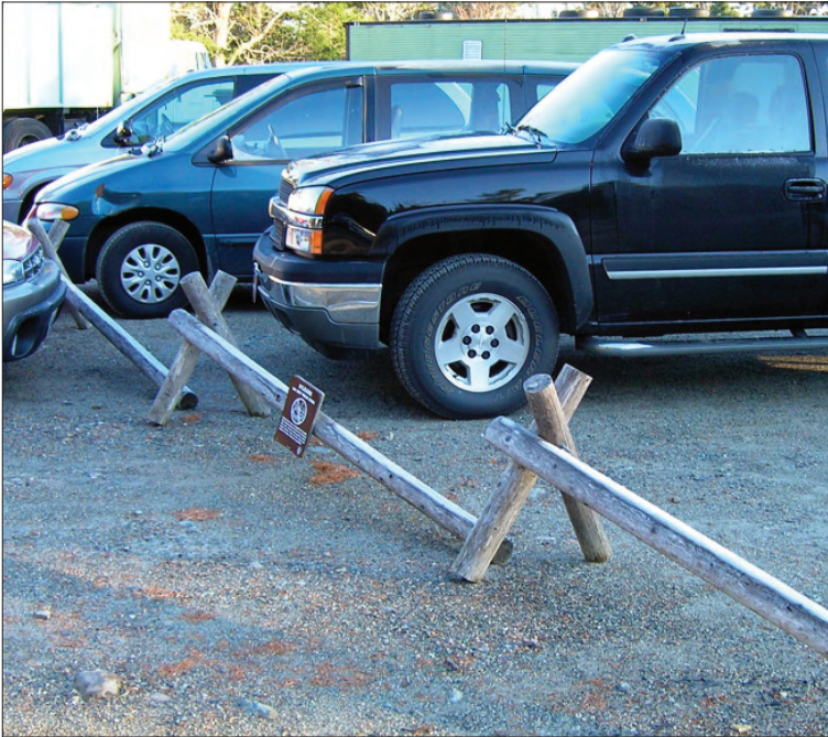
Figure 4.14. Similar barriers are found in use elsewhere in the national park system to control access and to organize otherwise informal parking on gravel lots that require winter-time snow removal. The barriers may be turned 90 degrees to the direction of travel for use as a moveable bollard (OCLP, 2006).
