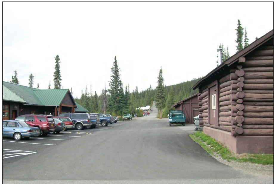
Figure 4.4. Preserving Service Area Character - Vehicular access to the historic service court will be limited by the installation of removable barriers, in order to eliminate through-traffic from the center of the historic district. This paved area will also be given a chip-seal surface treatment to better simulate the rustic gravel surface present during the pre-WWII period of significance (OCLP, 2006).
