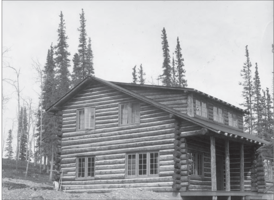
Figure 1.22. View northeast of the superintendent's residence (Building 1). Photographed by Joseph S. Dixon, Field Naturalist for the NPS, June 2, 1932 (DENA-70-4-34, Harpers Ferry Center).
