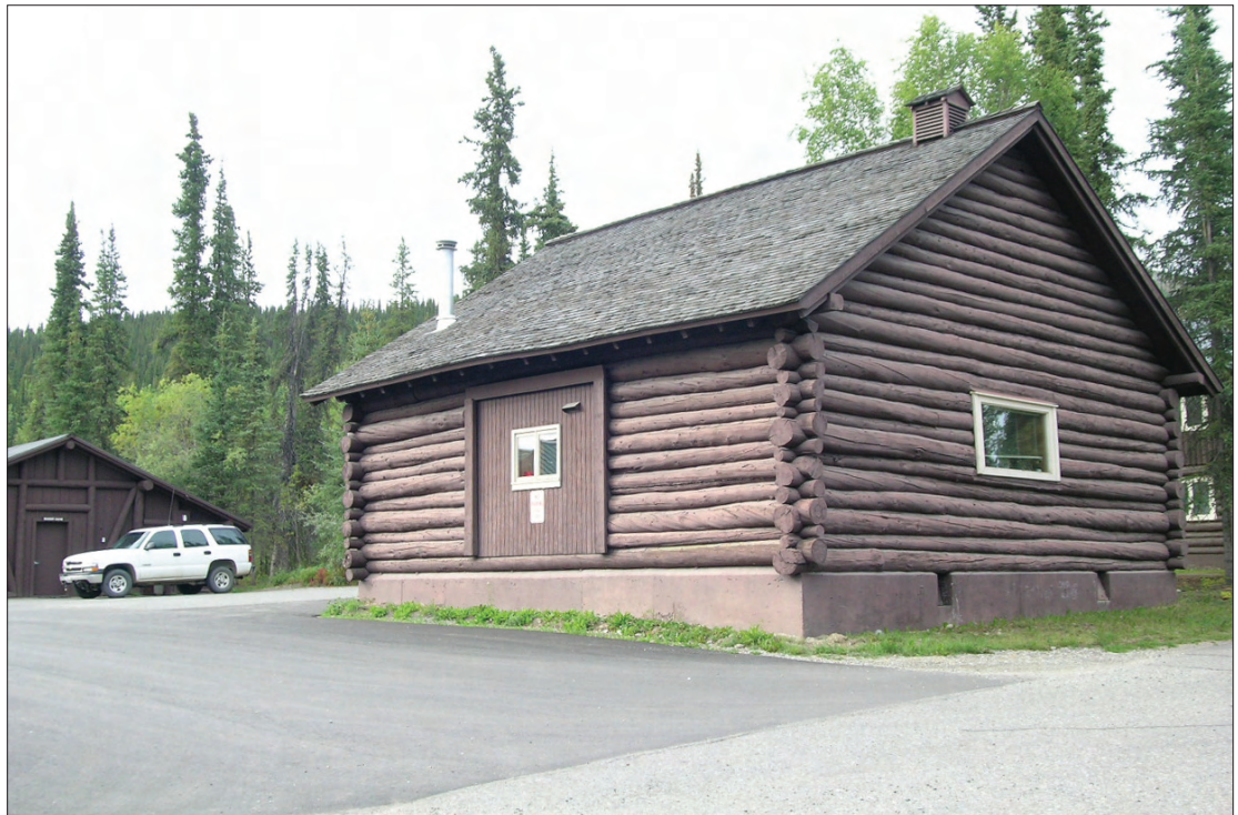
Figure 3.36. View looking northwest of Building 101 (original warehouse), August 2005. Note building changes including the in filled double doors, roof surface, concrete foundation, and absence of the loading dock. Also note the garage (Building 103) at left and the asphalt service road foreground and main headquarters road at right (OCLP).
