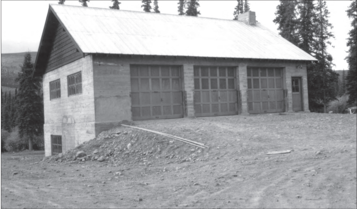
Figure 3.37. View looking southwest toward the garage and repair shop (Building 102), August 14, 1939. Also note the earthen ramp leading up to the garage doors, service drive (right foreground) and main headquarters road (left) (DENA 3 2, Denali National Park and Preserve Museum Collection).
