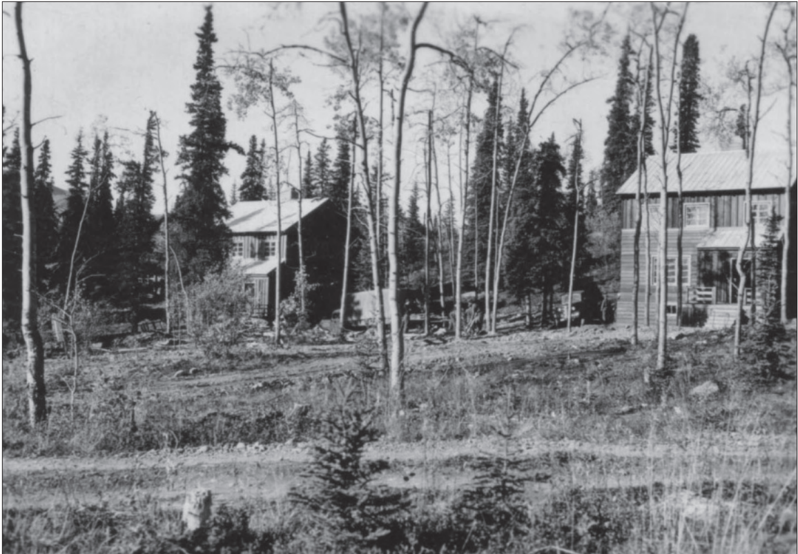
Figure 1.42. View to west of the two employee residences (Building 12 and Building 13), 1939. Note the small spruce trees planted by the CCC, the drive leading to Building 12, and the road in the foreground. This road, constructed in 1932, originally led to the dog kennels before the kennels were moved in 1939 (NPS, Alaska Regional Office, Regional Cultural Resources (RCR) program files).
