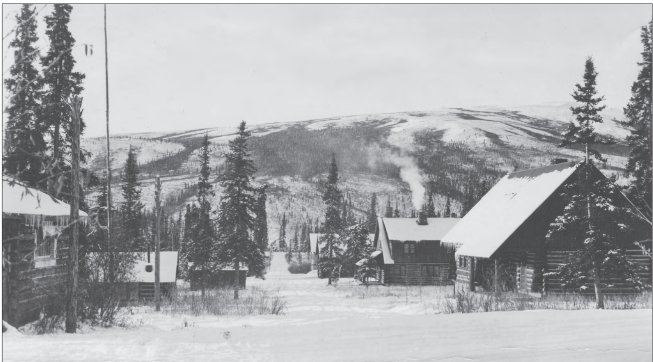
Figure 1.52. View south down the main headquarters road, c. 1940-1941. Buildings from left to right: original park office (Building 22, use in 1941 unknown), one-car garage that was the original electric light shop (Building 110), temporary one-car garage built in 1938, machine shop and garage (Building 102), warehouse (Building 101), rangers' dorm (Building 21), and administrative building that was the original employee's quarters (Building 11). Note the utility pole without lines north of Building 110. Note the herbaceous quality of understory vegetation growing near the roadway (DENA 3-7.7, Denali National Park and Preserve Museum Collection).
