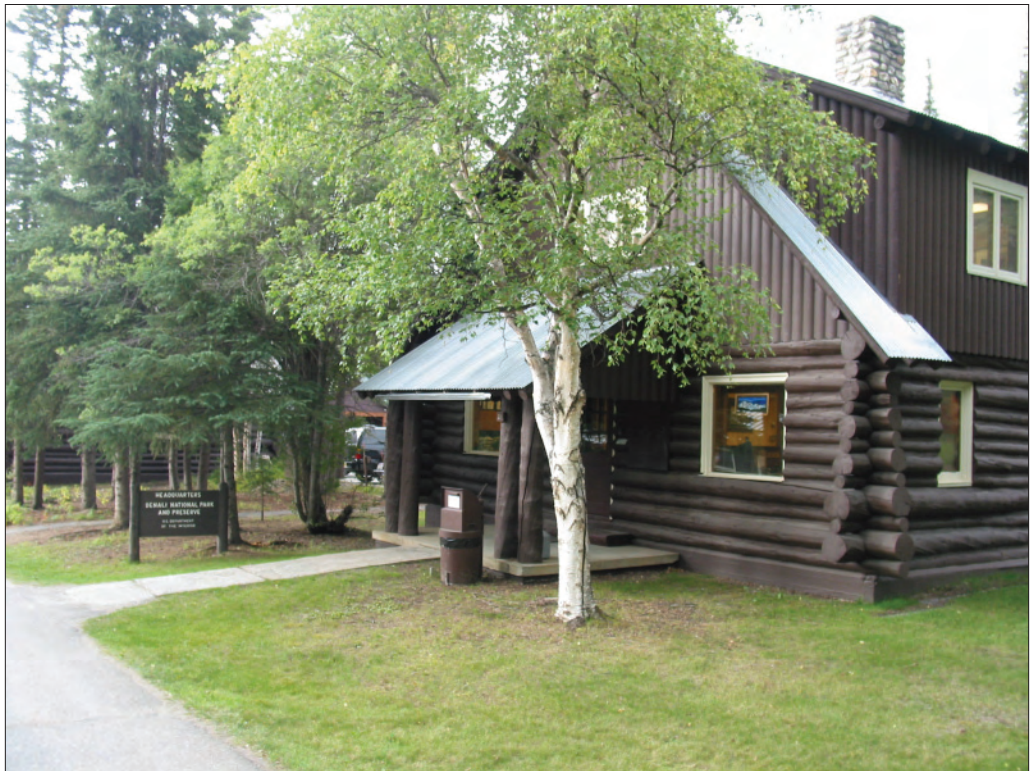
Figure 3.23. View southwest of the administration building (Building 21, original rangers' dorm), August 2005. Note building changes including the replacement windows and roofing material. Also note Building 101 (original warehouse, far left behind the grove of evergreen trees), the lawn around the building, and the asphalt main headquarters road at the left of the image (OCLP).
