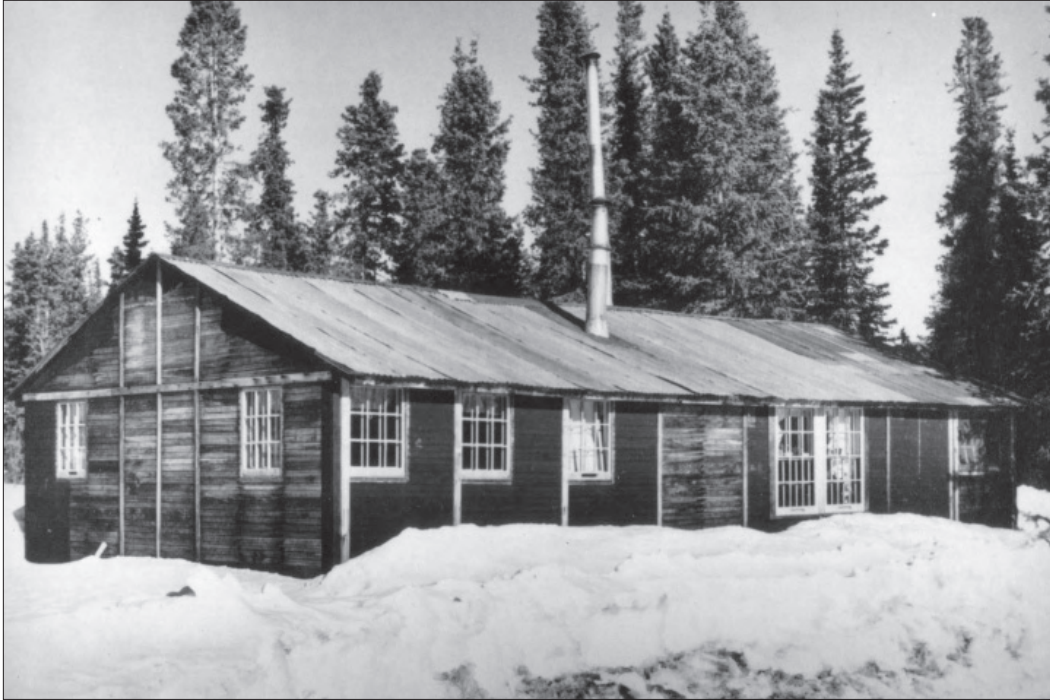
Figure 1.57. Quarters 24 (Building 123, original infirmary at the CCC camp), c. 1950. According to a label on the photograph, this residence was also known as "Mosquito Manor." (DENA 7-10, Denali National Park and Preserve Museum Collection).
