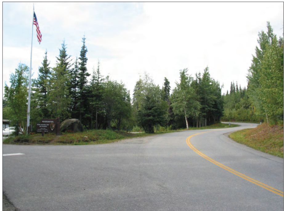
Figure 4.27. Circulation and Parking - Improve Sight-Distances at Park Road - Treatment Task 3.B - As seen in this photograph of existing conditions, the clearance of brush, understory and trees from the inside of the adjacent curve on the Denali Park Road would greatly improve sight-distances at the Headquarters entrance without impacting the historic landscape (OCLP, 2006).
