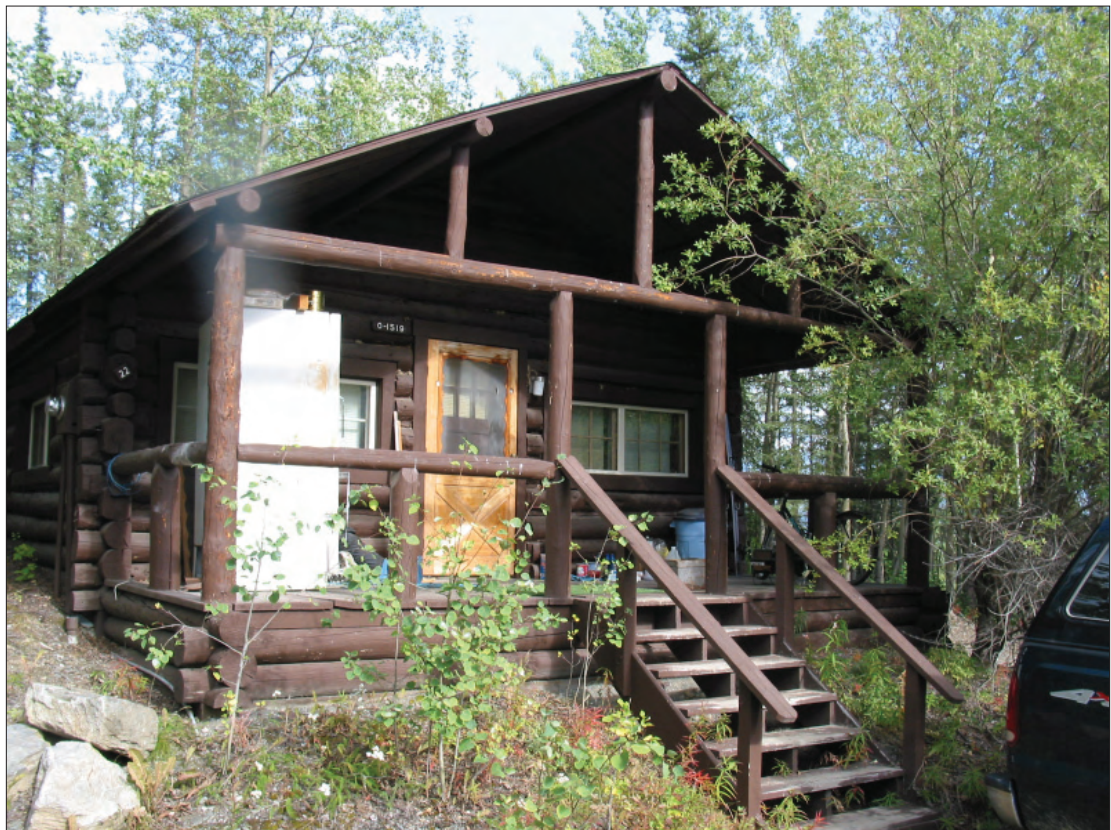
Figure 3.34. View of southwest facade of Building 22 (original superintendent's office) in its current location north of the park road. This small building now serves as an employee residence. Note building changes including the front porch and stairs, and the painted peeled log exterior (OCLP, 2005).
