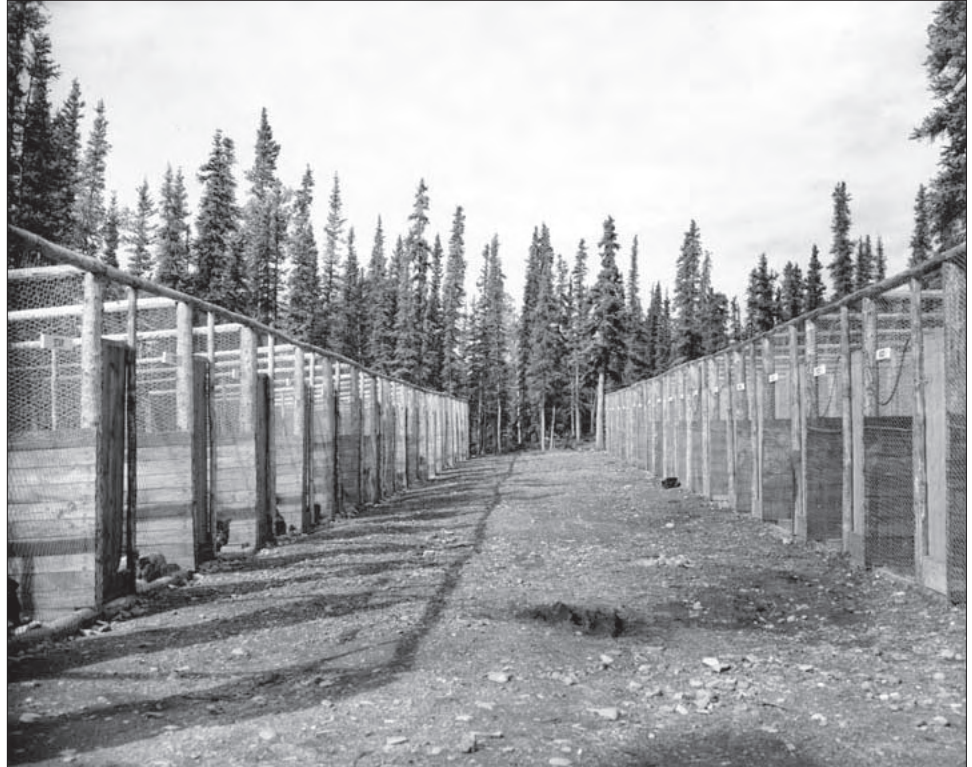
Figure 1.38. View west of the completed dog kennels, August 1938 (Ickes Collection, B75-175-303, Anchorage Museum of History & Art).
