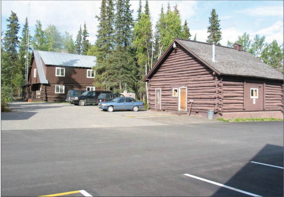
Figure 4.9. Circulation and Parking - Eliminate central parking and through-traffic - Treatment Tasks 1.A and 1.C - Remove bituminous pavement proliferating at the center of the district after WWII. Existing conditions shown above detract greatly from the historic character of the property (OCLP, 2006).
