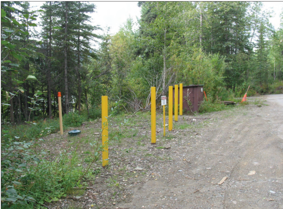
Figure 2.15. Safety bollards mark the location of a fuel storage tank (August 2005, OCLP).
