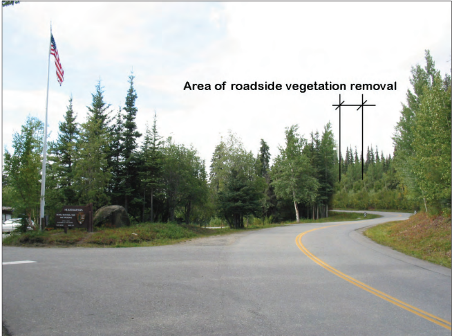
Figure 4.28. Circulation and Parking - Improve Sight-Distances at Park Road - Clear trees and brush from adjacent curve - Treatment Task 3.B - As seen in this photo-simulation, immediate improvements to sight-distances on the park road may be economically obtained (OCLP, 2007).
