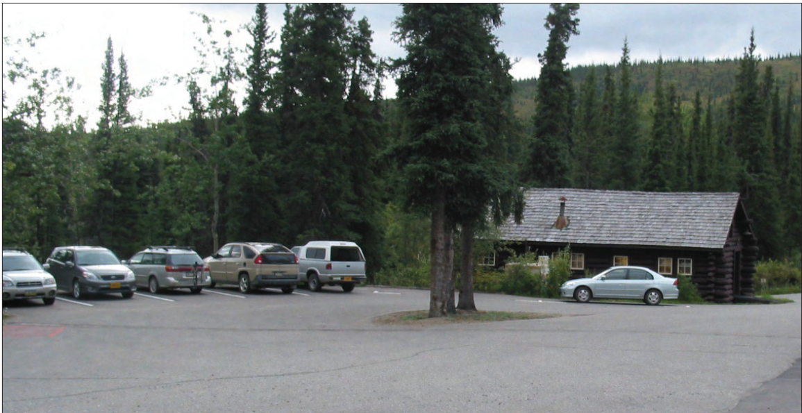
Figure 3.15. View southeast of the u-drive, August 2005. The parking area occupies the location of the oil and gas house (Building 108) and oil cans adjacent to the building depicted in the figure above. The island of mature evergreens is the same group depicted (left) in the figure above. Building 106 (original barn) is seen to the right (OCLP)..
