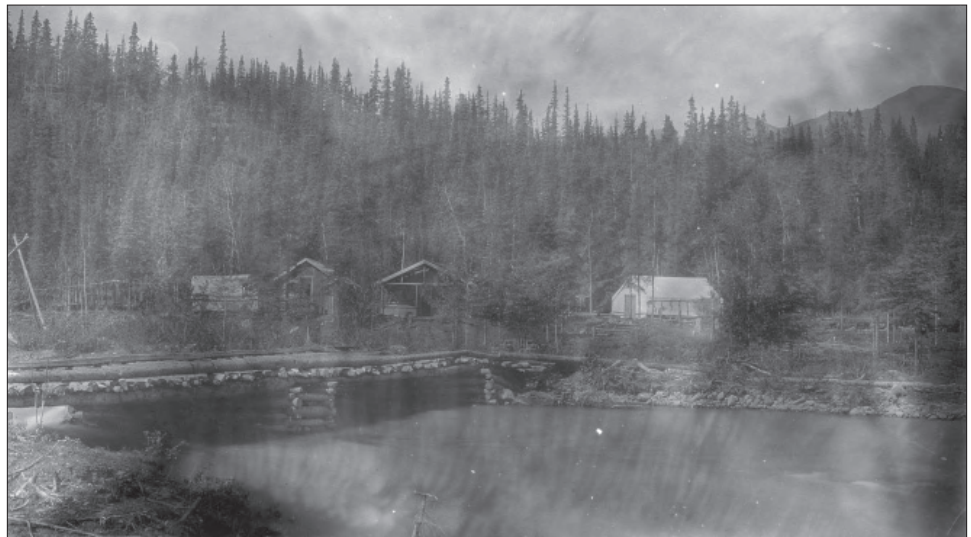
Figure 1.2. View to the southwest of the Riley Creek headquarters area, July 31, 1922. Buildings from left to right: tent (use unknown), superintendent's office, superintendent's "home cabin," small building (possibly "the necessary outbuilding") and a large tent, which was probably the storehouse and workshop. Also depicted is Riley Creek (foreground), a log bridge over the creek with crib piers and log decking, what appears to be a tri-pod phone line at far left, and a small area bounded by a post and rail fence (Dartmouth College Library).
