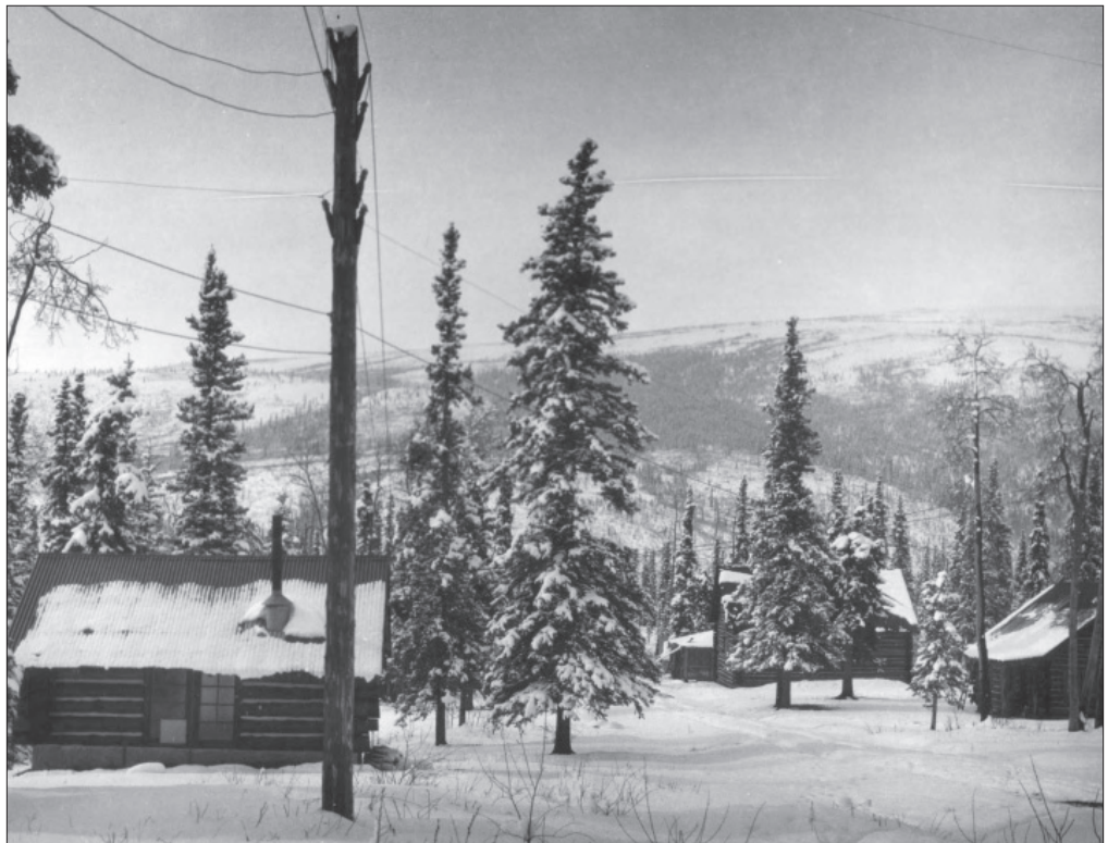
Figure 1.29. View of new utility poles carrying electric and telephone wires, 1932. Buildings depicted in the photograph include, from left to right: electric light house (Building 110), combination machine, workshop, blacksmith shop (original garage, workshop, and blacksmith shop, built in 1927), warehouse (Building 101), and rangers' quarters (built in 1928). The main headquarters road (covered in snow) runs between the buildings (photo center) (DENA 3-34, Denali National Park and Preserve Museum Collection).
