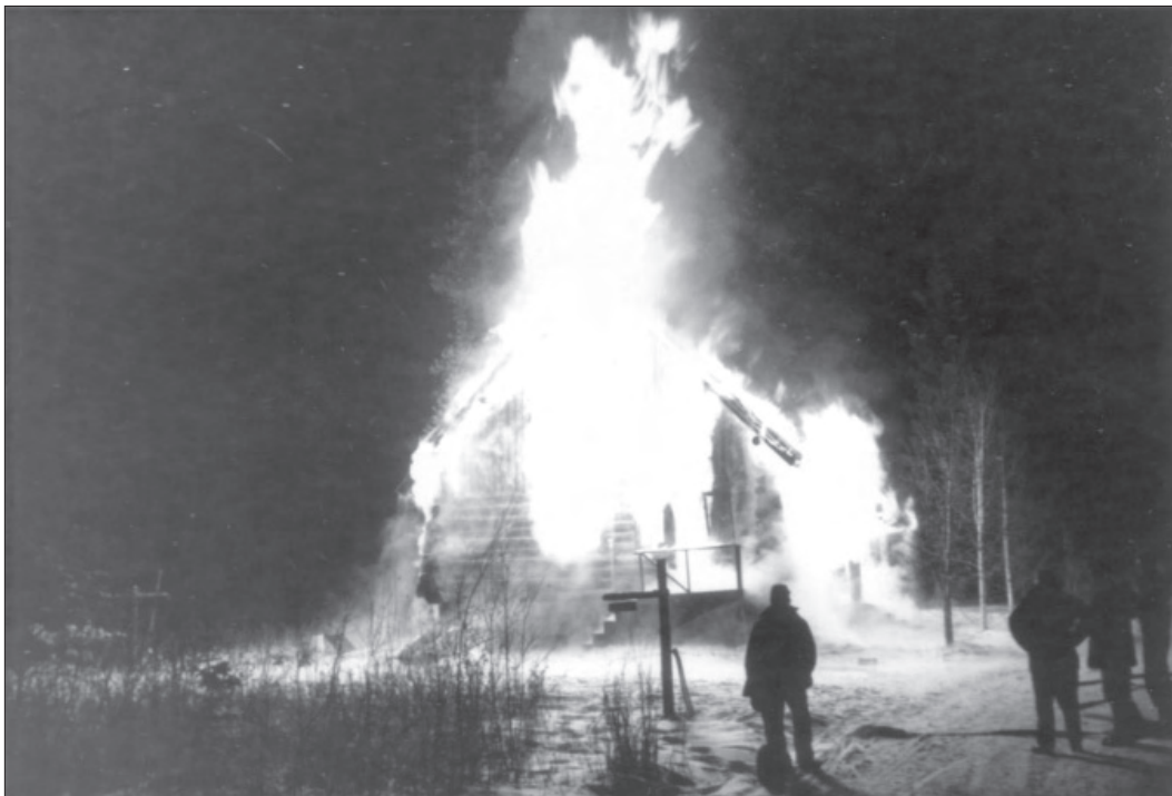
Figure 1.60. View of the employee's residence (Building 11) on fire, November 3, 1950 (DENA 8-9, Denali National Park and Preserve Museum Collection).
