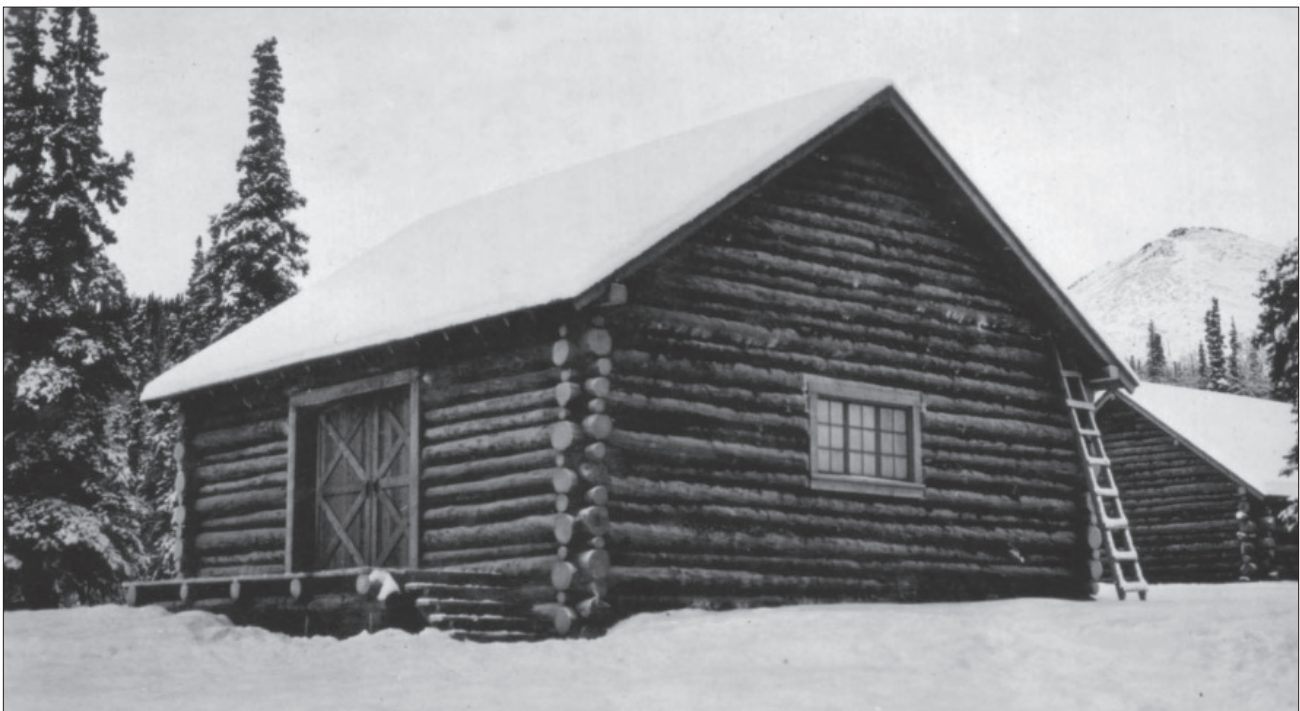
Figure 1.19. View northwest of the warehouse (Building 101) built in 1928 and the ranger quarters (right) built in 1928-29, photo dates to c. 1929-1930 (DENA 1501, Denali National Park and Preserve Museum Collection).
