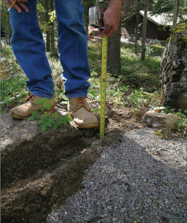
Figure 4.17. Circulation and Parking - Enhance Roadside Character and Vegetation - Treatment Task 2.A - Remove windrows of sand found developing at road shoulders. Accumulations of sand develop into windrows at the shoulder of Denali Park Headquarters roadways impeding the flow of surface drainage from the roadway, and destroys roadside vegetation (OCLP, 2006).
