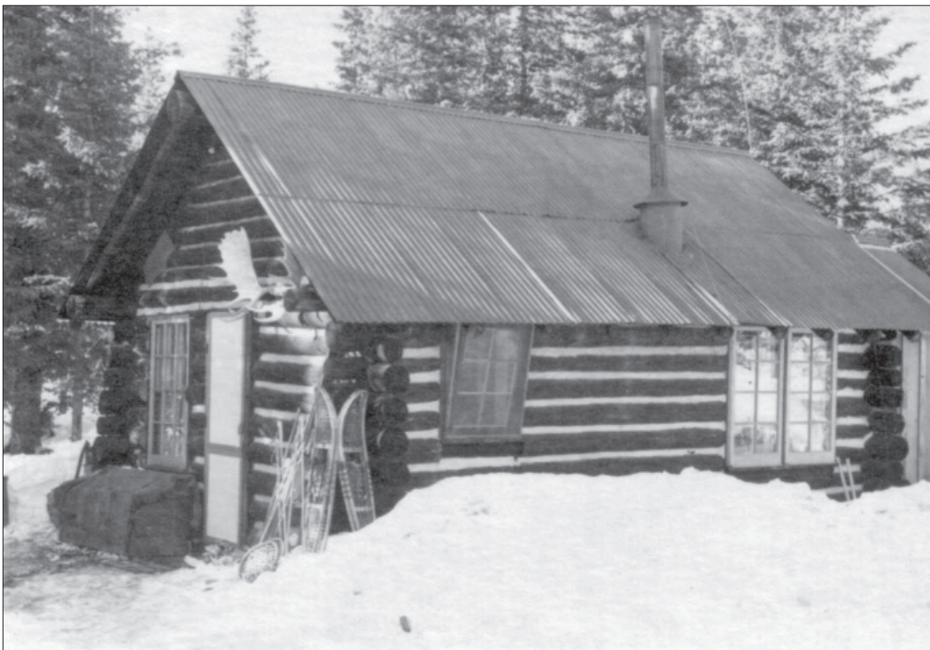
Figure 1.58. Laborers' quarters (Building 6), March 1950 (DENA 7-7, Denali National Park and Preserve Museum Collection).
