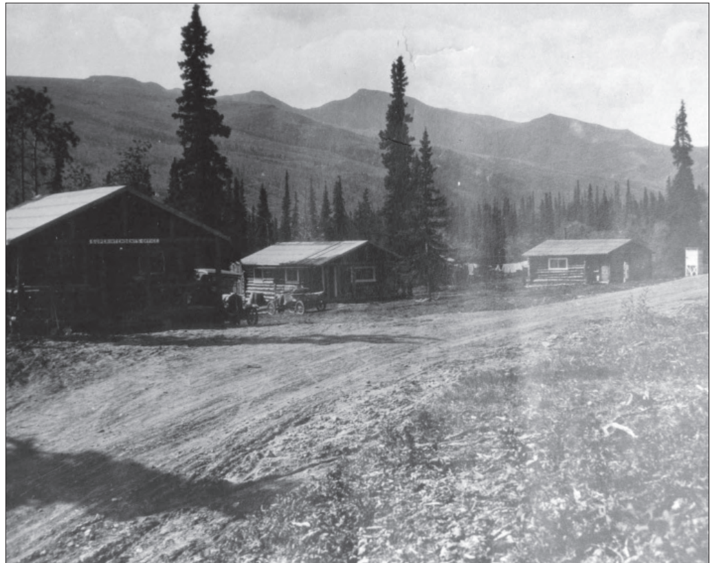
Figure 3.1. View southwest from park road, mid-1920s, prior to construction of the flagpole. Pictured from left to right is the superintendent's office (Building 22), original superintendent's cabin, and original clerk's cabin (DENA 4-2, Denali National Park and Preserve Museum Collection).
