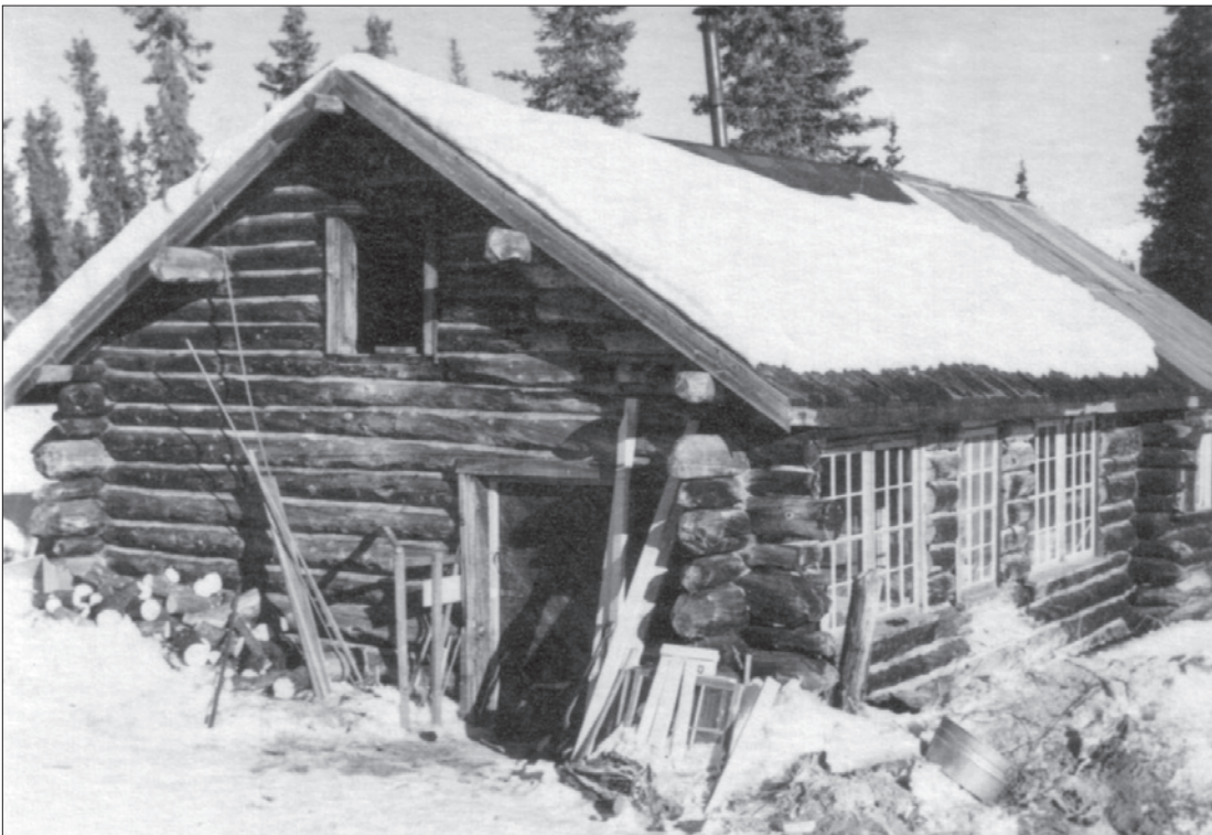
Figure 1.56. Carpentry shop (Building 106, original barn), March 1950 (DENA 3-14, Denali National Park and Preserve Museum Collection).
