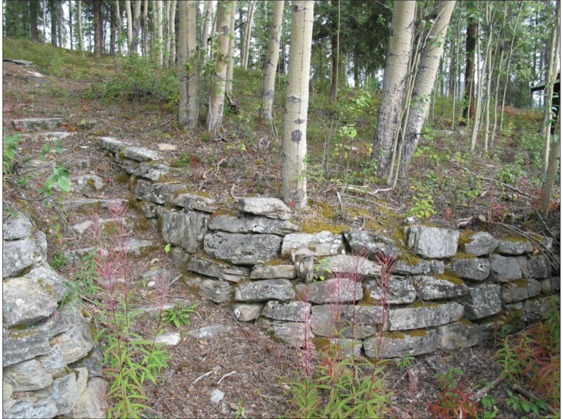
Figure 3.31. View northeast of stone retaining wall and steps (111A) built by the CCC in 1939 (August 2005, OCLP).
