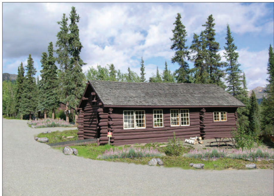
Figure 4.23. Circulation and Parking - Enhance Roadside Character and Vegetation - Treatment Tasks 2.B, 2.C and 2.D - This photo simulation depicts the effects of removing excess post WWII pavement (2.B), the protection of road shoulders with carefully placed boulder barriers (2.C), and resurfacing the bituminous drainage swale at the front door to Building 106 with stone rubble (OCLP, 2007).
