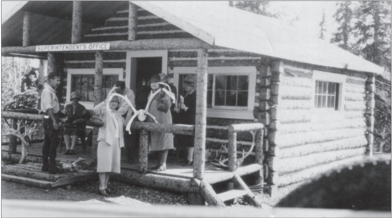
Figure 1.12. View south of the superintendent's office or park office (Building 22) in its original location along the south side of the park road, July 1, 1927. Note the sign above the porch entrance. This appears to be the same sign hung on the wood frame superintendent's office at the first headquarters at Riley Creek (see Figure 1.5) (DENA 14976, Denali National Park and Preserve Museum Collection).
