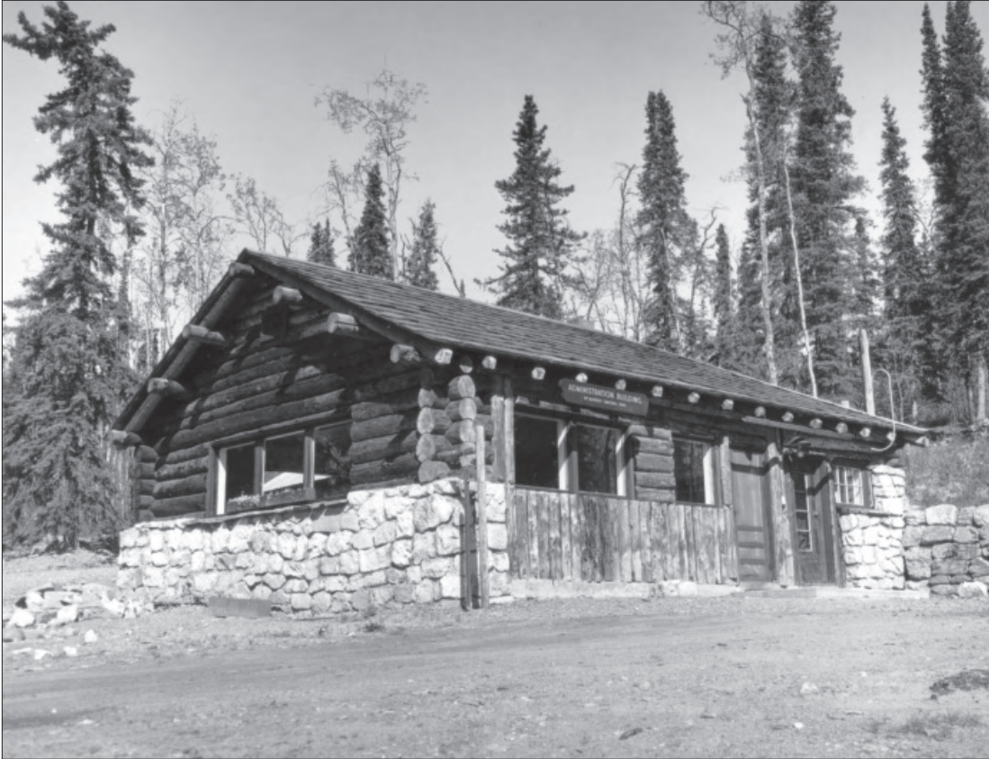
Figure 1.55. View northwest of the administrative building (Building 111, original superintendent's garage), c. 1946-1950. Note the gravel driveway in front of the building and the stone retaining wall (111A) (DENA 3-8, Denali National Park and Preserve Museum Collection).
