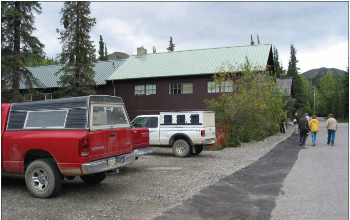
Figure 3.17. View northwest of parking area behind Building 102 (original machine shop and garage), August 2005. The dark pavement is a recently added drainage swale (OCLP).
