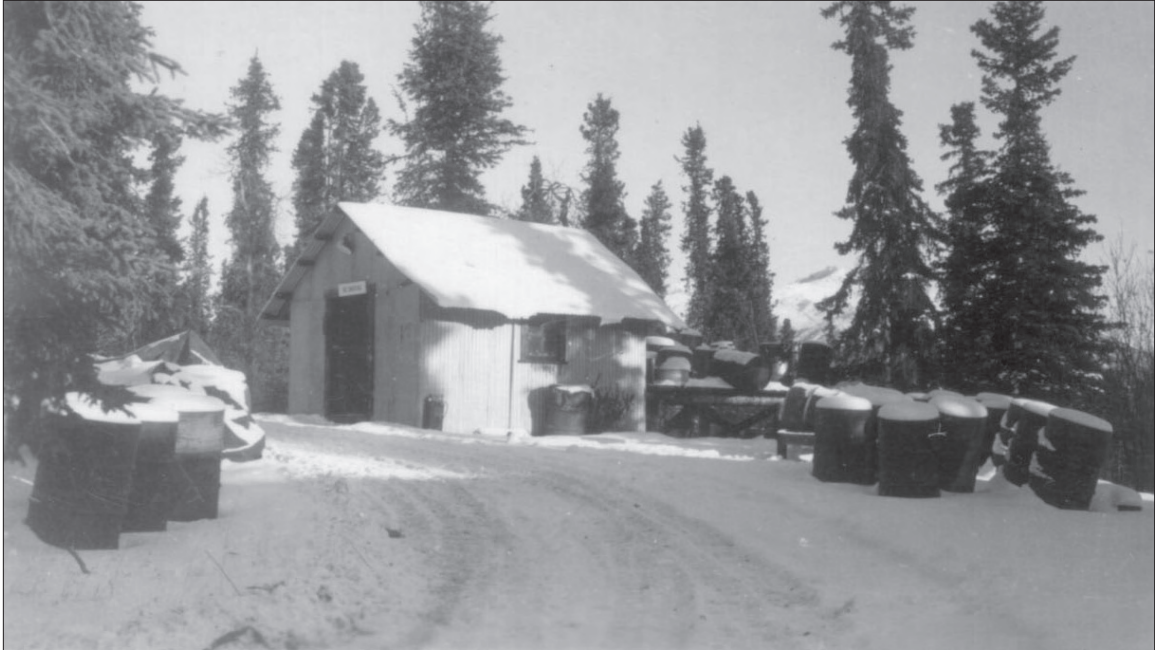
Figure 3.14. View northeast of the u-drive leading to the oil and gas house (Building 108), c. 1950. Note the narrow width of the drive (DENA 10483, Denali National Park and Preserve Museum Collection).
