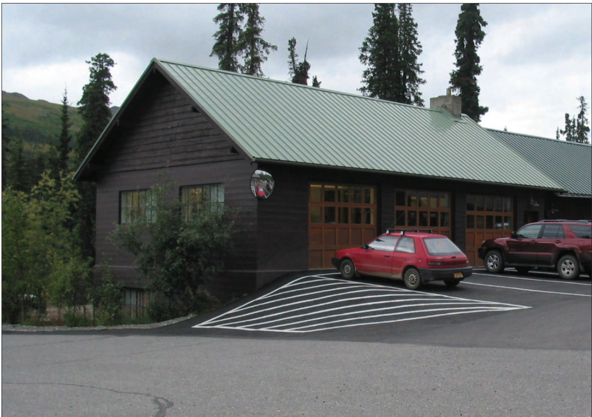
Figure 3.38. View looking southwest toward Building 102 (original garage and repair shop), August 2006. Note building changes including the painted concrete exterior and the roof surface. Also note the asphalt pavement leading to faux garage doors (parking spaces), service court at right, and the north-south headquarters road at left in the foreground (OCLP).
