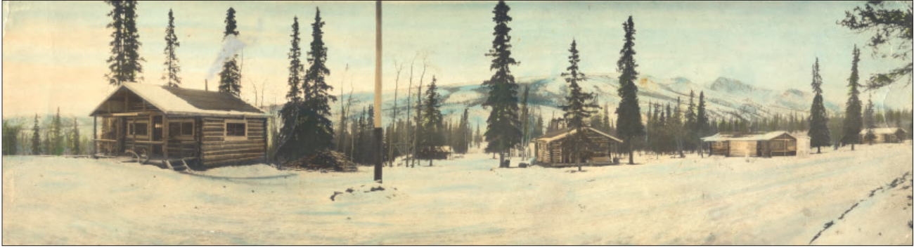
Figure 1.18. Panoramic view of the park headquarters, showing flag pole installed at the intersection of the park road (foreground) and the main headquarters road (center, back of flag pole). Also note the park buildings, from left to right: superintendent's office (Building 22), rangers' cabin (center, distance), superintendent's cabin, clerk's cabin, and chief ranger's cabin at far right (DENA 3555, Denali National Park and Preserve Museum Collection).
