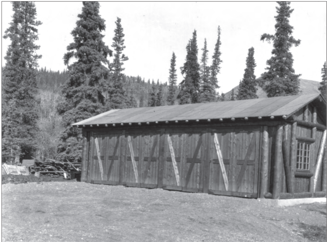
Figure 1.27. View northwest of the garage (Building 103), c. 1937 (DENA 3-33, Denali National Park and Preserve Museum Collection).
