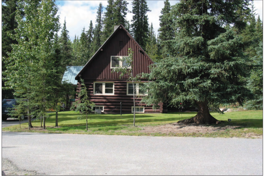
Figure 4.24. Circulation and Parking - Enhance Roadside Character and Vegetation - Treatment Task 2.F - Establish an eight-foot-wide buffer of native vegetation between the edges of headquarters roads and areas of managed turf. Maintained turf, such as this lawn surrounding the historic Superintendent's residence, is widely enjoyed by Headquarters residents for social events and for play during the brief summer season (OCLP, 2006).
