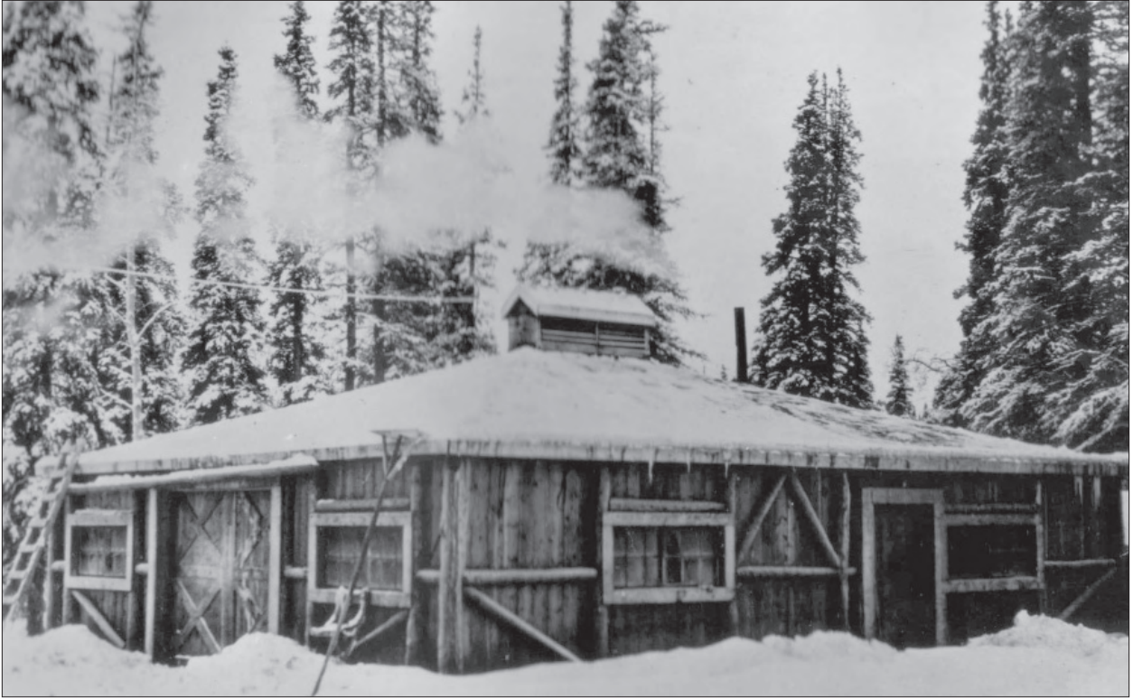
Figure 1.16. Combination garage, workshop, and blacksmith shop located to the west of the wood frame barn (near the present Building 102), c. 1927-1930. Also note the tent structure on the right, the use of which is unknown. (Nyberg Photo Album, DENA 1501, Denali National Park and Preserve Museum Collection).
