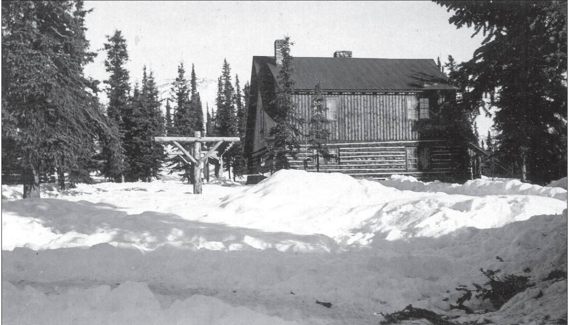
Figure 3.18. View north of rectangular area between the warehouse (Building 101, not depicted), garage (Building 103, not depicted), rangers' dorm (Building 21, depicted), and the laborer's quarters (Building 6, just visible behind trees, left). Although it is difficult to determine the use of the area closest to the service road (foreground), it is evident by the location of the log clothes line that parking would not have occurred between Building 6 and Building 21. Unnumbered photograph, Denali National Park and Preserve Museum Collection)
