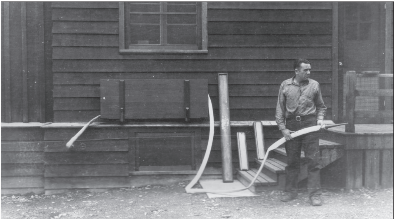
Figure 1.48. Weather proof fire hose box and hose connections, c. May 1940. A note attached to the original photo from a superintendent's monthly report, dated the same month, remarked "weather proof fire hose box and hose connections installed at buildings supplied with water." Depicted is one of the two employee's residences (Building 12 or 13) built by the CCC in 1938 (National Archives and Records Administration, College Park, MD).
