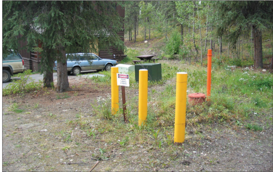
Figure 4.44. Small-Scale Features - Replace prominent safety bollards with appropriate rustic measures - Treatment Task 1.B - Replace non-historic steel bollards and otherwise visually prominent safety barriers with non-historic alternatives that are consistent with the historic character of the landscape. In this view of existing conditions, the visual prominence of both the barriers and the utility features detract from the rustic character of the landscape (OCLP, 2006).
