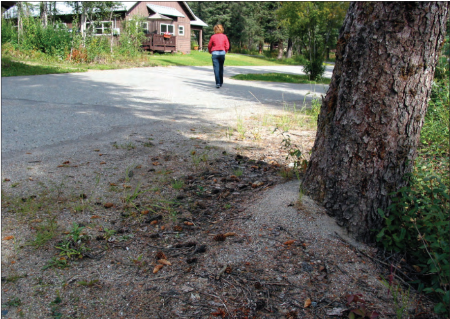
Figure 4.18. Circulation and Parking - Enhance Roadside Character and Vegetation - Treatment Task 2.A - Remove windrows of sand found developing at road shoulders. Over time, accumulation of roadside sand, has the visual effect of widening the roadway, promoting roadside parking that further damages vegetation (OCLP, 2007).
