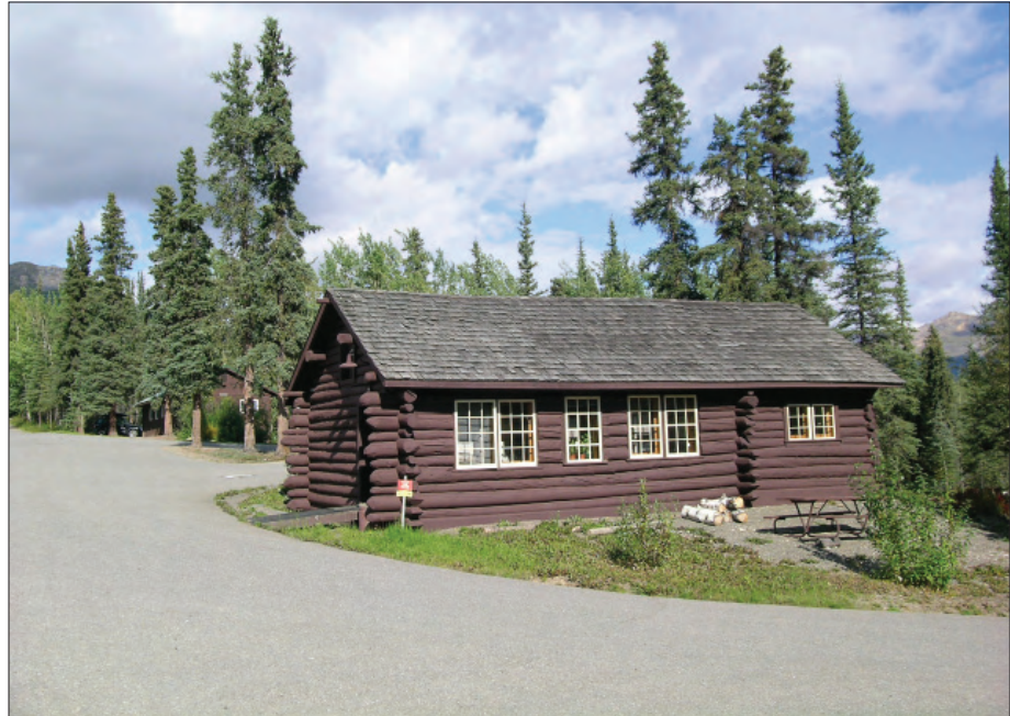
Figure 4.22. Circulation and Parking - Enhance Roadside Character and Vegetation - Treatment Tasks 2.B, 2.C and 2.D - The piecemeal widening of roadways and paved surfaces as illustrated by this photograph, have encroached on the setting of historic log buildings and compromises the historic character of the Denali Park Headquarters District (OCLP, 2006).
