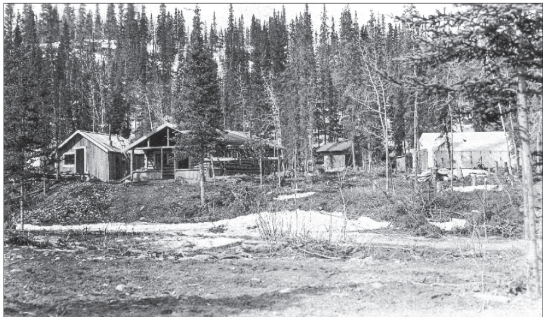
Figure 1.4. View southwest of the headquarters, along west side of Riley Creek. Buildings left to right include a small structure obscured by trees (use unknown), superintendent’s office, superintendents “home cabin,” small frame structure (possibly frame meat and storehouse), very small frame structure (possibly “necessary building”) and a large tent, which was probably a storehouse and workshop (DENA 4678, Denali National Park and Preserve Museum Collection).
