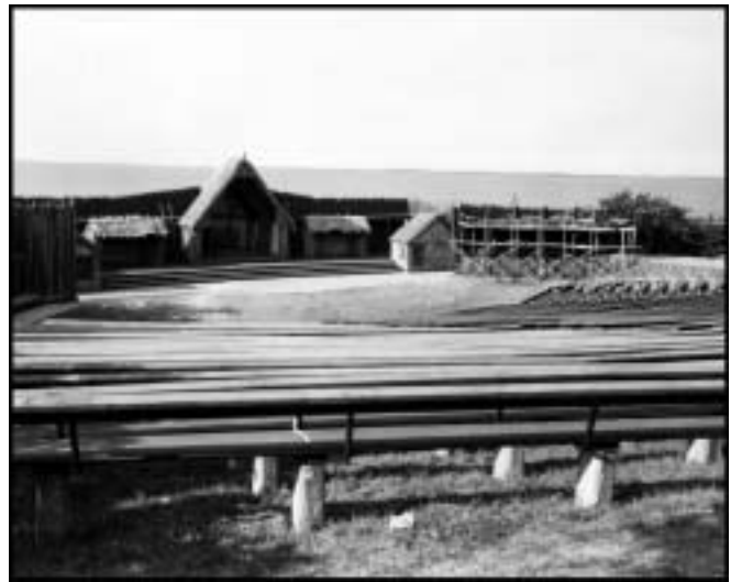
FIGURE 23. The Waterside Theater after the building sets were changed in appearance from log to wattle in May 1955
