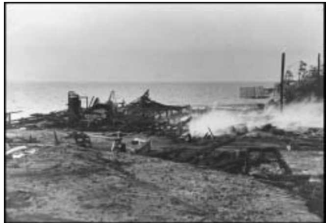
FIGURE 42. Waterside Theatre fire damage, July 1947
