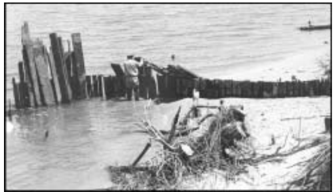
FIGURE 53. Jetty under construction east of Fort Raleigh, ca. 1950
