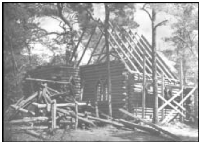
FIGURE 22. The WPA chapel at Fort Raleigh being demolished, April 1952
