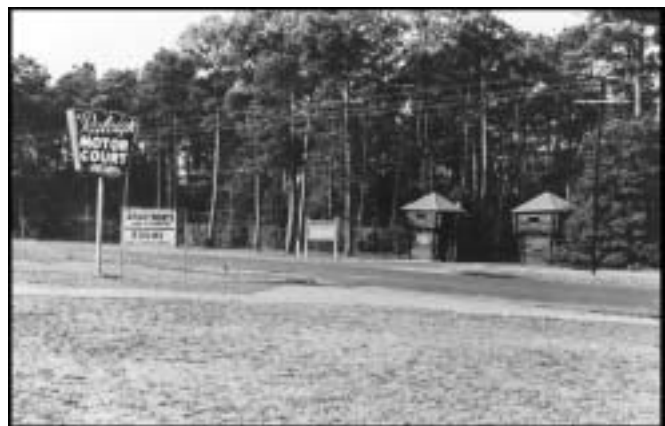
FIGURE 20. View of front gate to Fort Raleigh, February 1960
