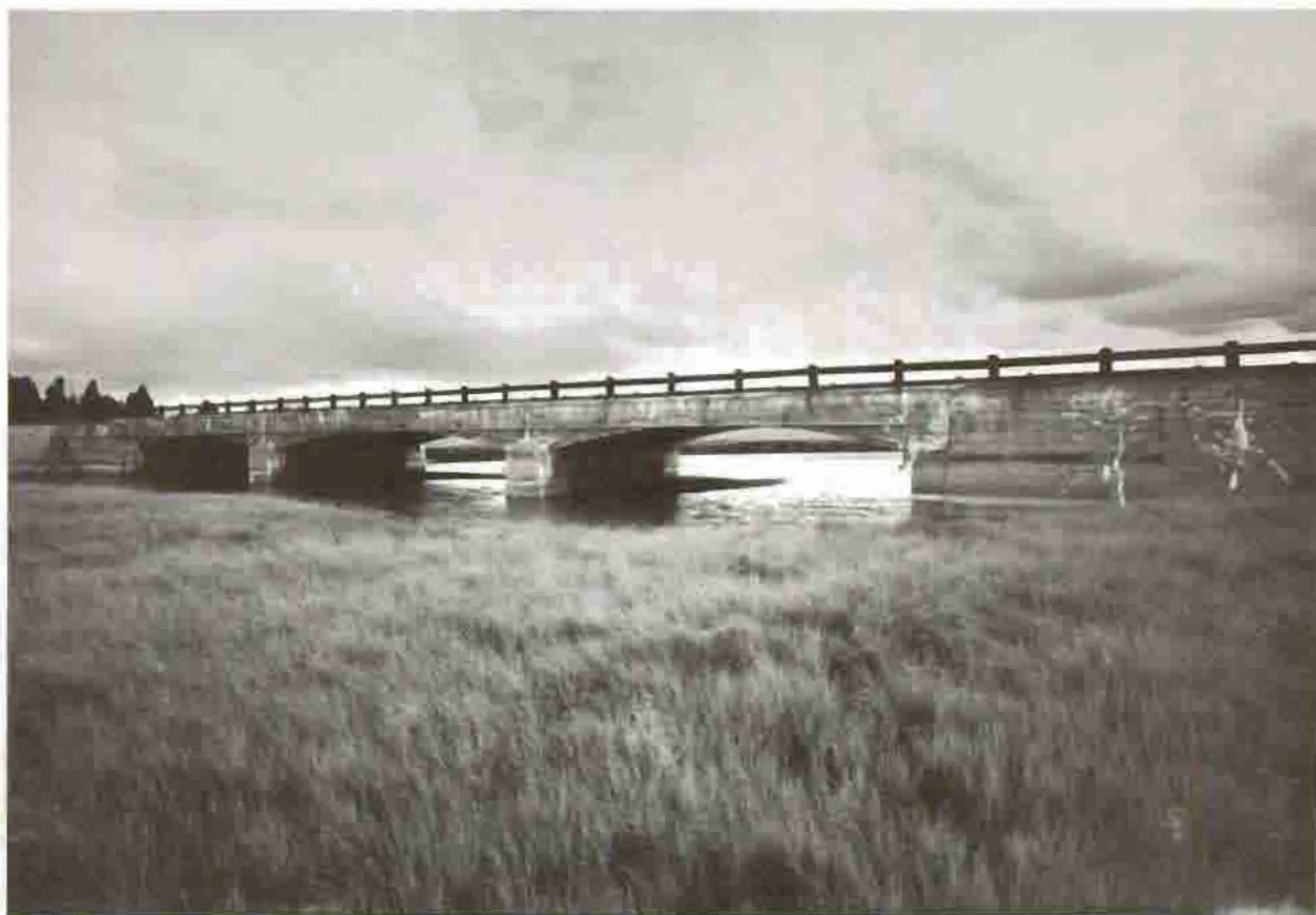
Pelican Creek Bridge, 1989 Courtesy Historic American Engineering Record, Jet Lowe
