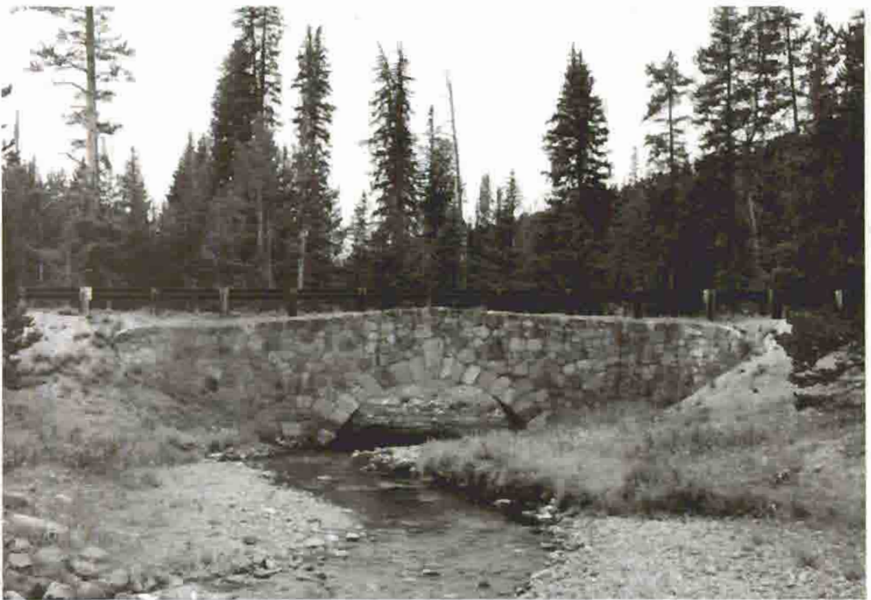
Cub Creek Bridge, 1989 Courtesy Historic American Engineering Record, Jet Lowe, 1989
