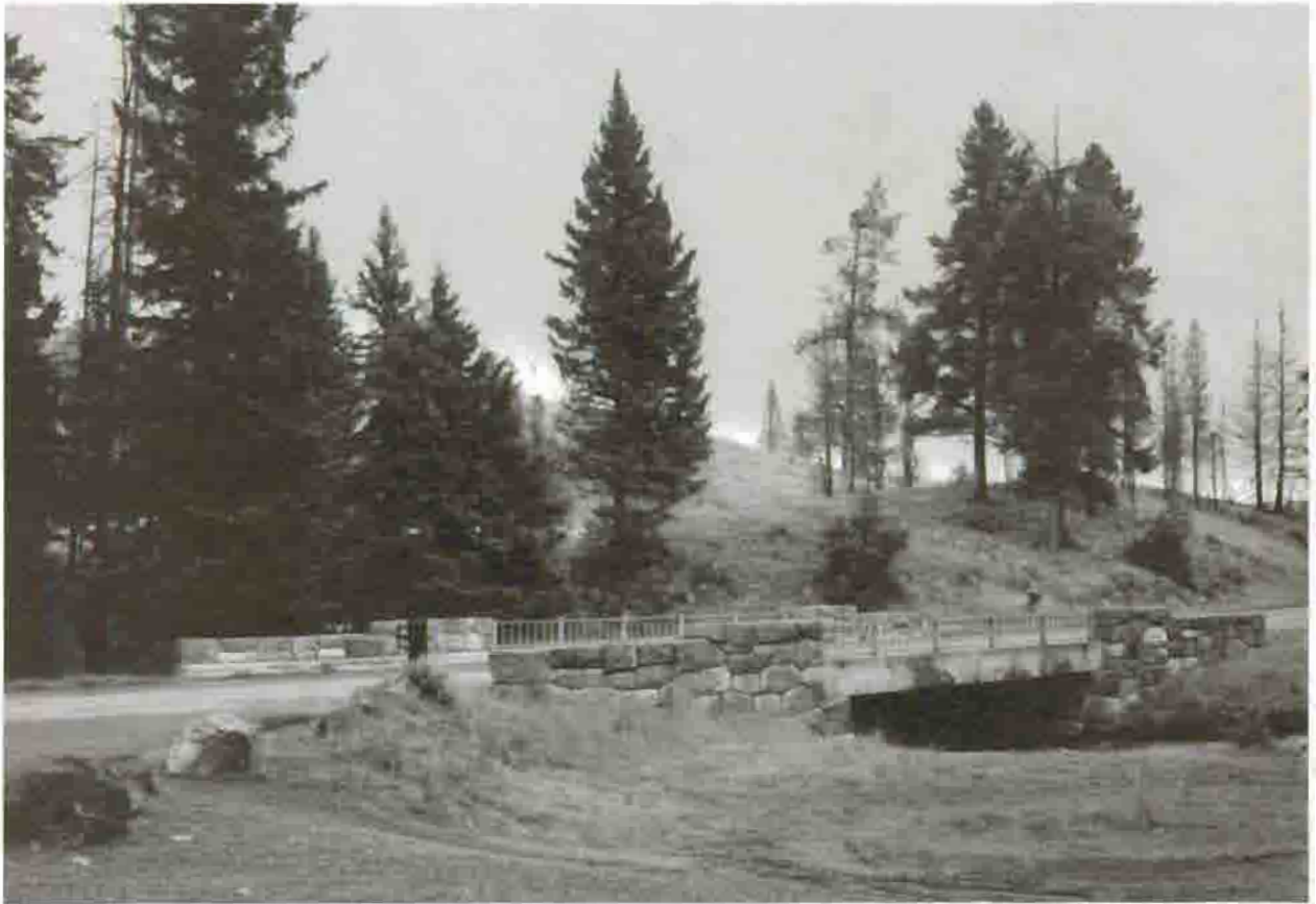
Lava Creek Bridge, 1989 Courtesy Historic American Engineering Record, Jet Lowe, 1989
