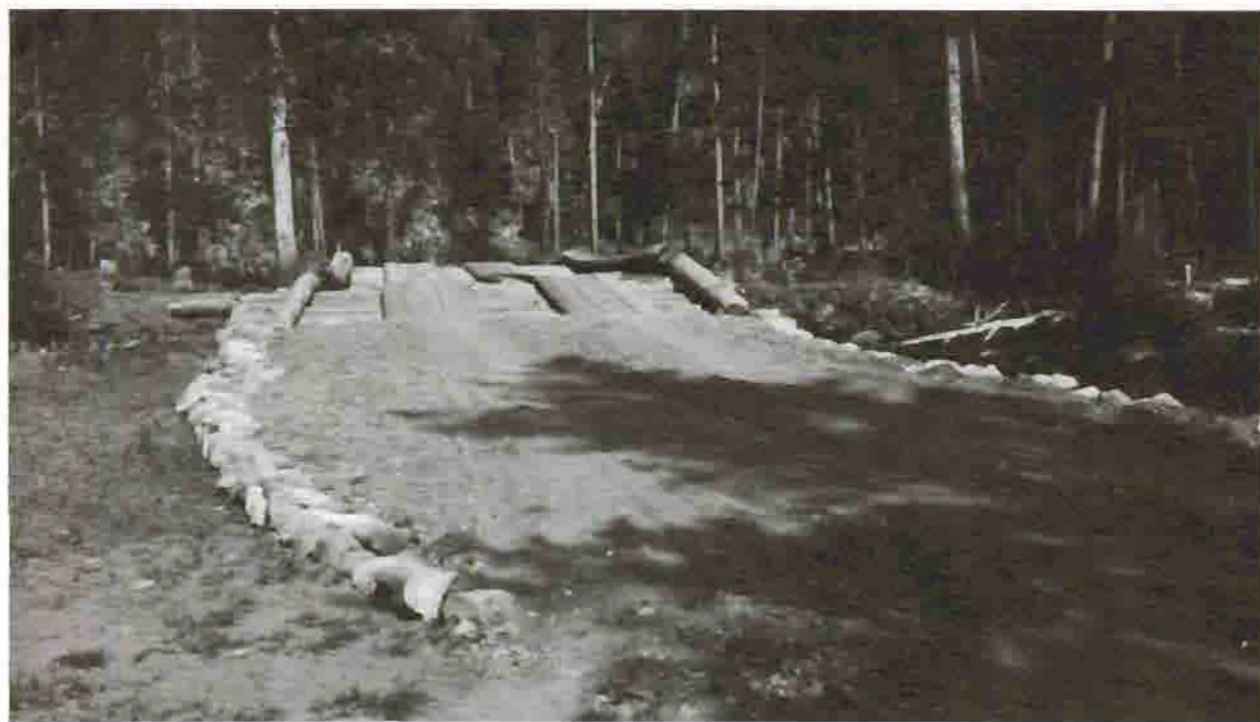
Pebble Creek Bridge, 1930 Courtesy Yellowstone National Park Archives
