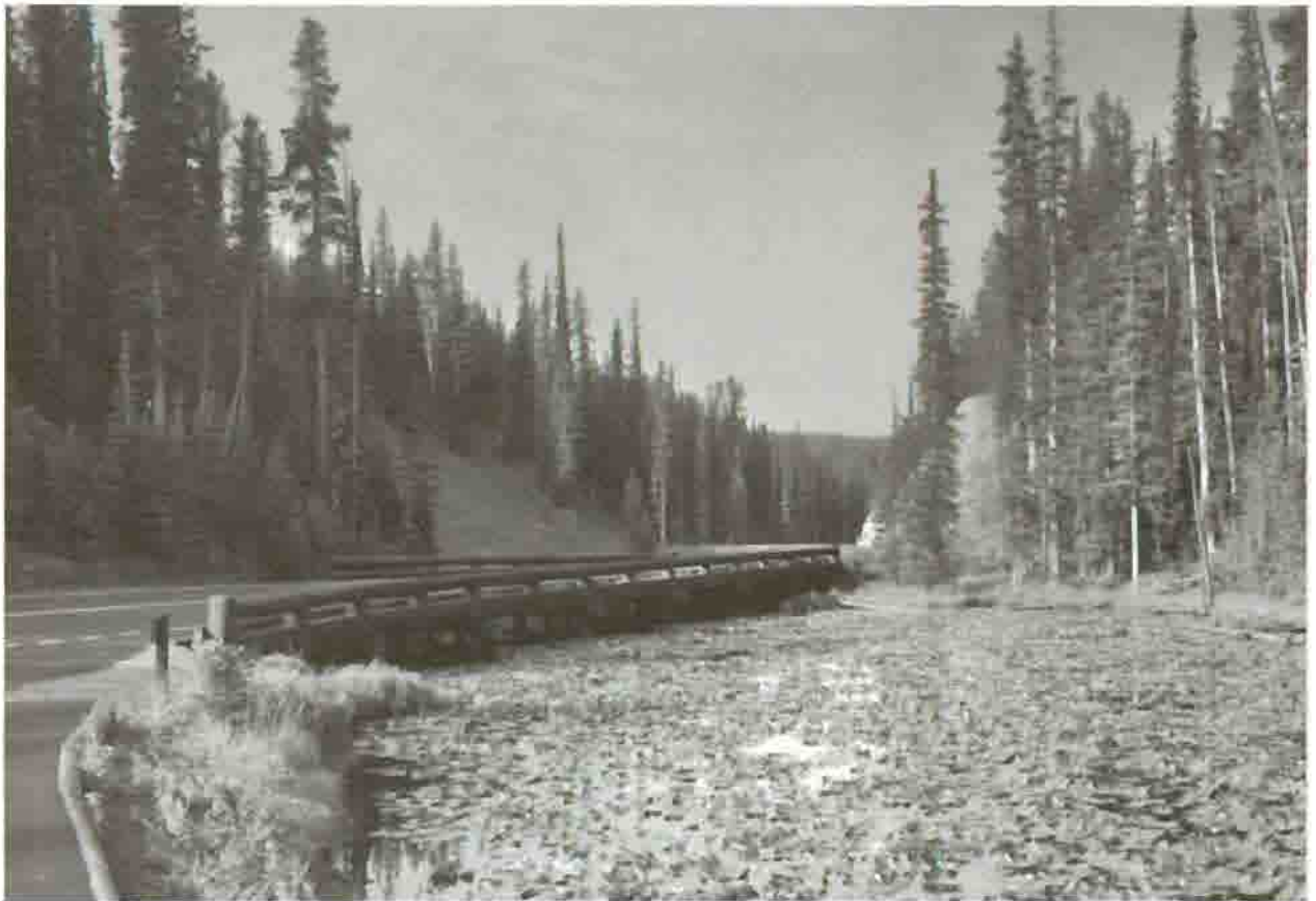
Isa Lake Bridge, 1989 Courtesy Historic American Engineering Record, Jet Lowe, 1989
