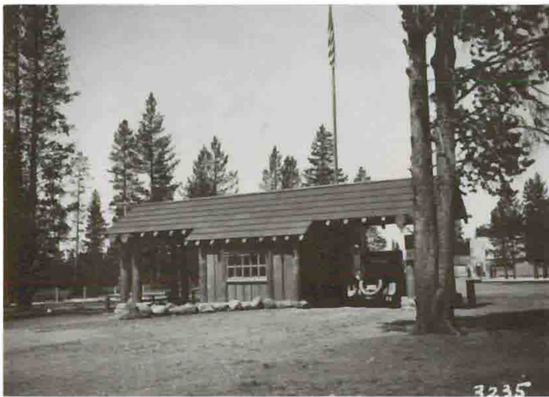
West Entrance Station, 1924 Courtesy Yellowstone National Park Archives
