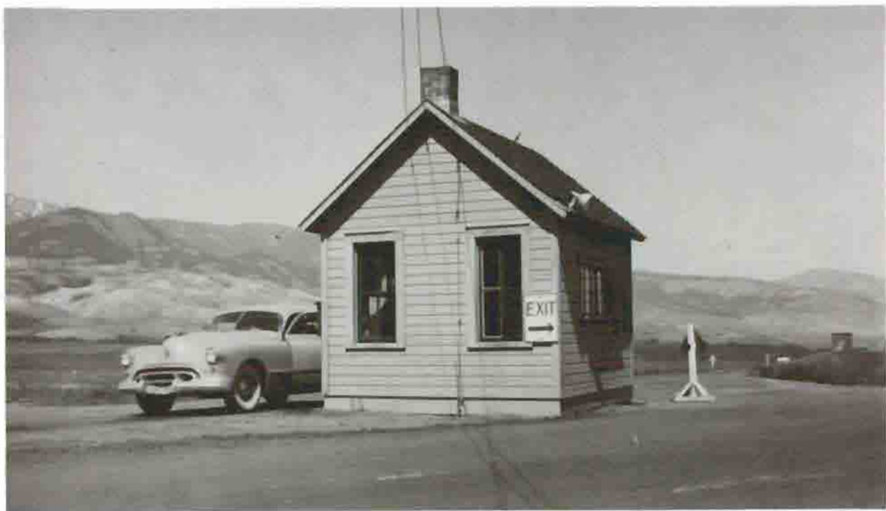
North Entrance Checking Station, 1949 Courtesy Yellowstone National Park Archives
