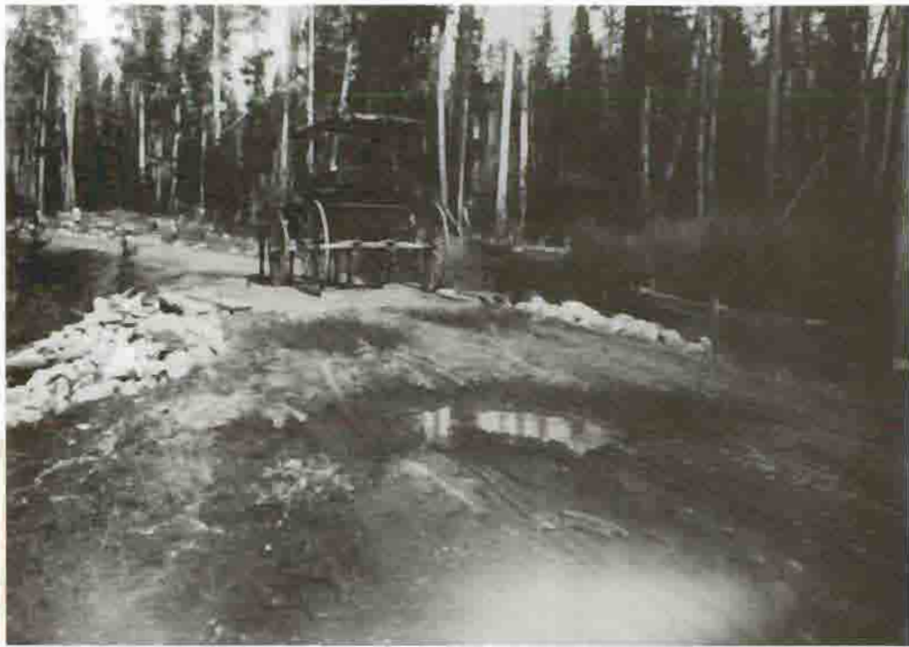
1 to 2 Milepost on Old Faithful to West Thumb Road, 1912 Courtesy Yellowstone National Park Archives
