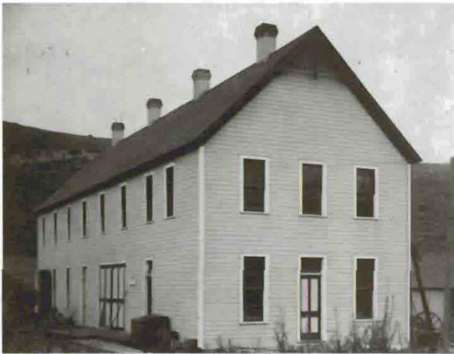
Bunkhouse and Shops, 1917 United States Army Corps of Engineers Courtesy Yellowstone National Park Archives
