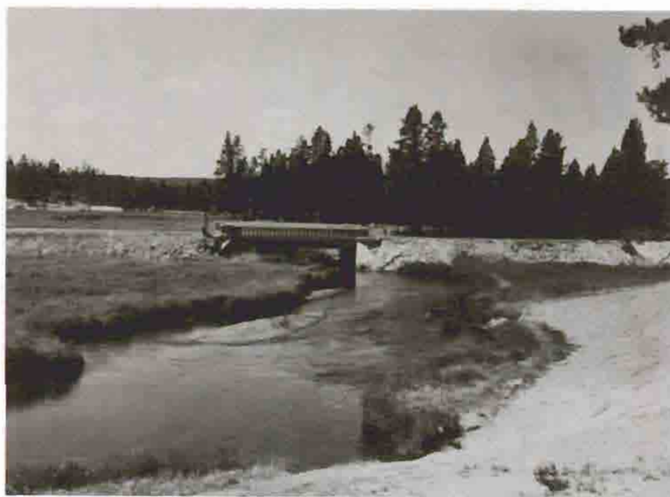
Gibbon River Bridge Near Norris Junction, 1953 Courtesy Yellowstone National Park Archives
