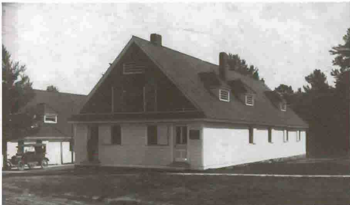
Commissary, 1917 United States Army Corps of Engineers Courtesy Yellowstone National Park Archives
