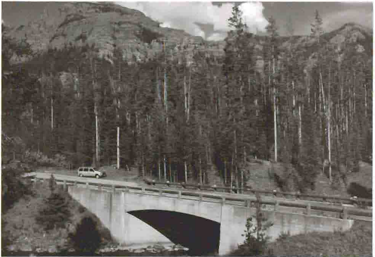
Soda Butte Creek Bridge Courtesy Historic American Engineering Record, Jet Lowe
