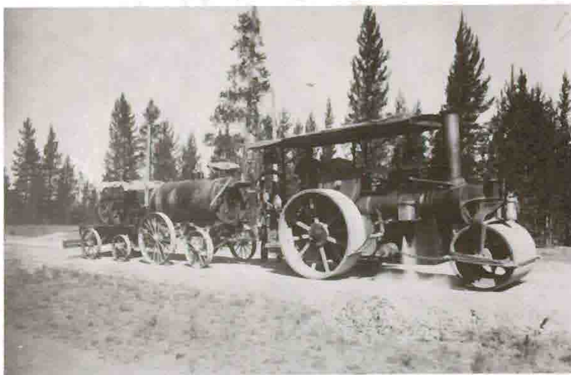
Oiling Road Two Miles from West Entrance, 1915 Courtesy Yellowstone National Park Archives
