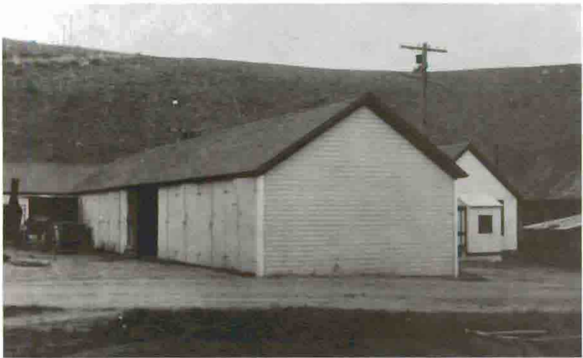
Shed, 1917 United States Army Corps of Engineers Courtesy Yellowstone National Park Archives
