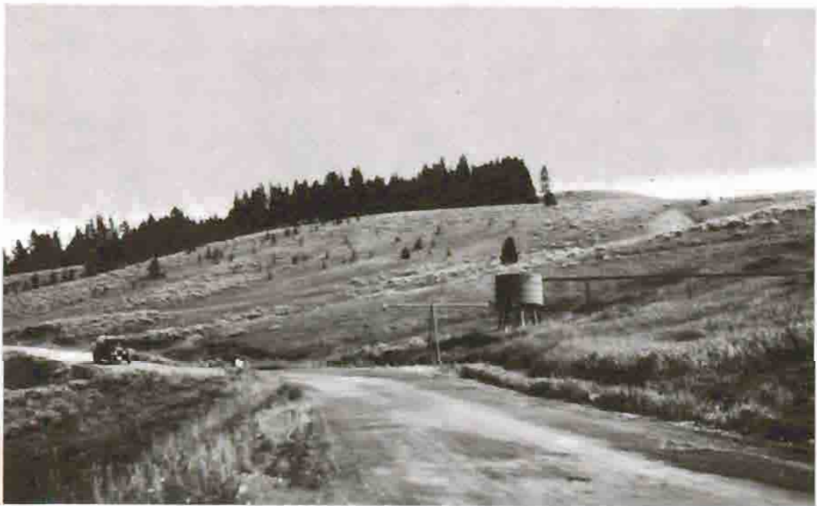
Old Water Tank, 7 Milepost, Lake to Canyon Road, 1929 Courtesy Yellowstone National Park Archives
