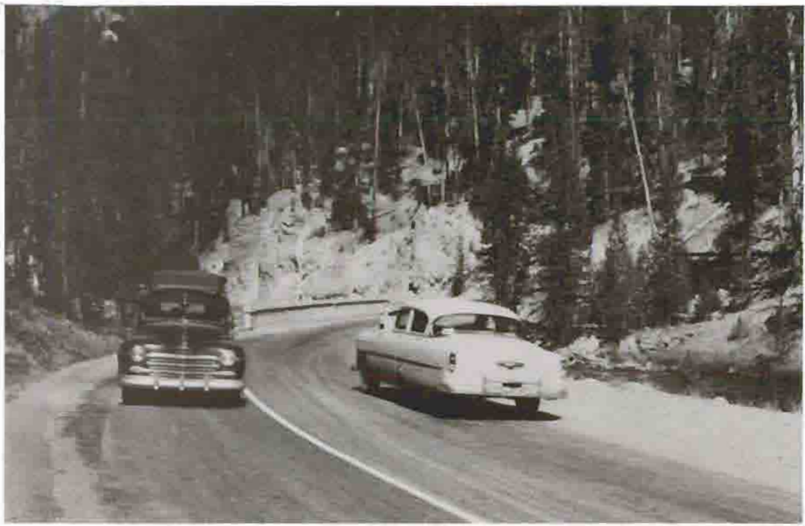
Gibbon River Bridge in Gibbon Canyon, 1953 Courtesy Yellowstone National Park Archives
