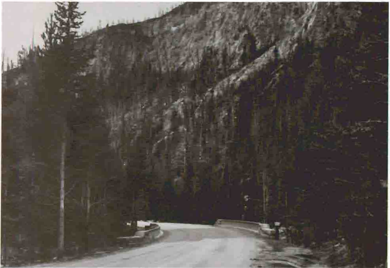
Gibbon River Bridge, 1989 Courtesy Historic American Engineering Record, Jet Lowe, 1989
