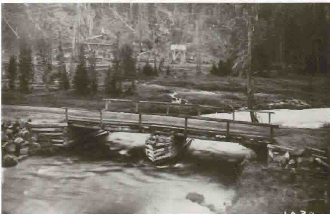
Gibbon River Bridge Below Wylie Camp Lunch Station, 1912 Courtesy Yellowstone National Park Archives
