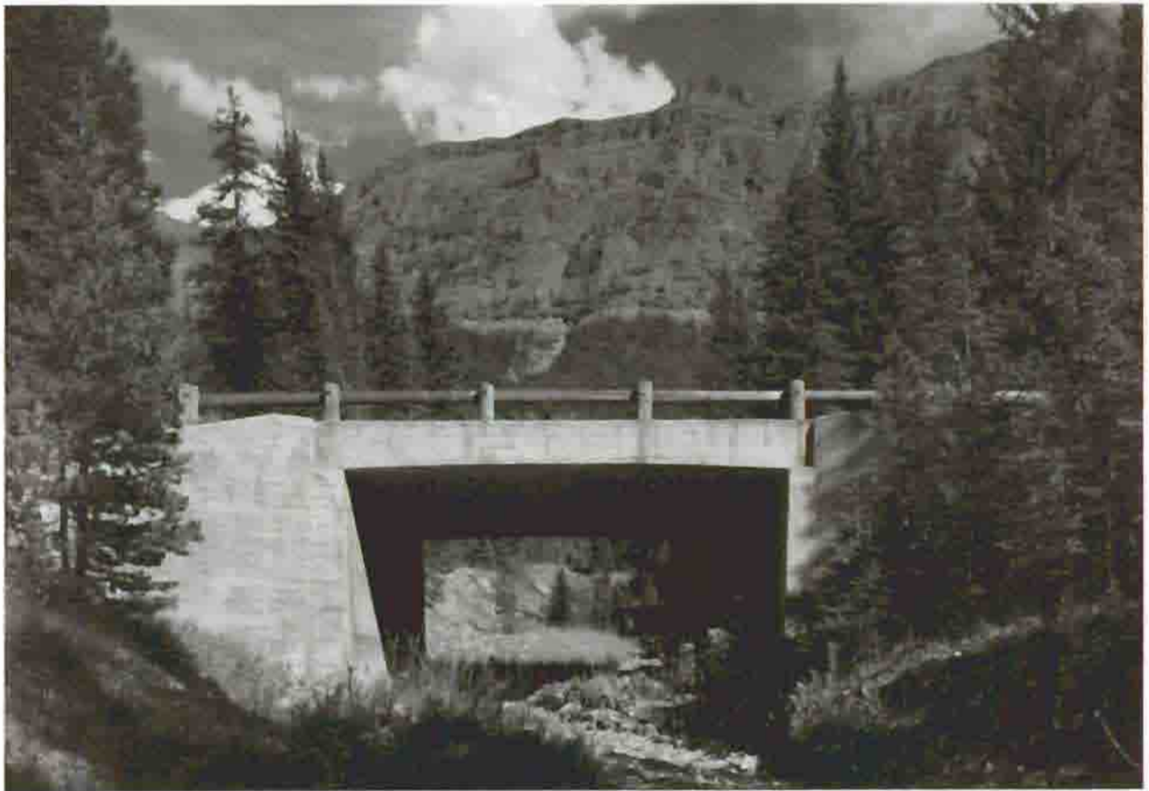
FHWA Creek Bridge Courtesy Historic American Engineering Record, Jet Lowe, 1989
