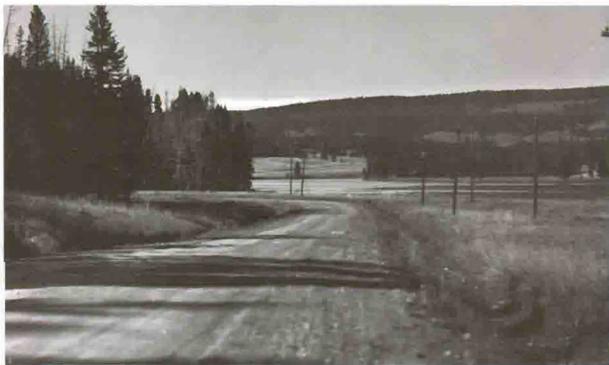
Telephone Lines Along Lake to Canyon Road, 1925 Courtesy Yellowstone National Park Archives
