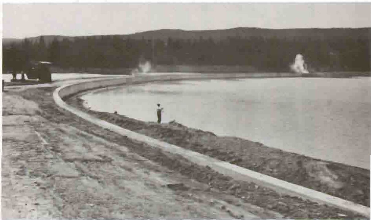
Bridge Bay Courtesy Yellowstone National Park Archives
