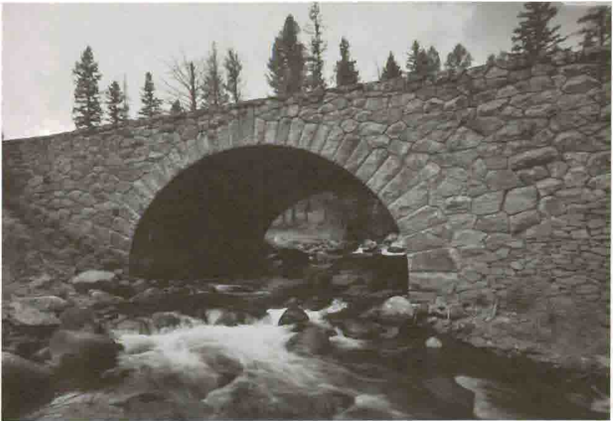
Crawfish Creek Bridge, 1989 Courtesy Historic American Engineering Record, Jet Lowe
