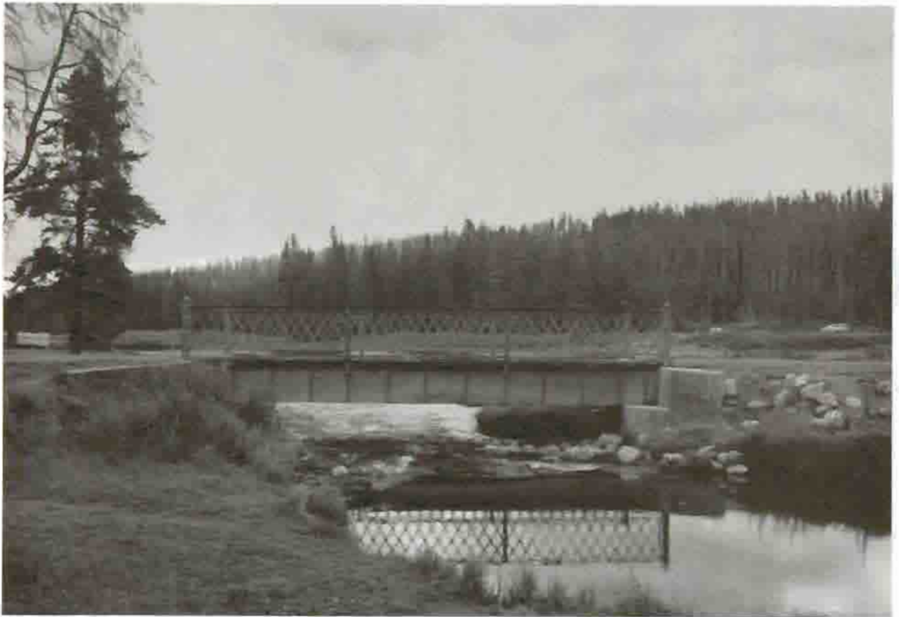
Obsidian Creek Bridge, 1989 Courtesy Historic American Engineering Record, Jet Lowe, 1989
