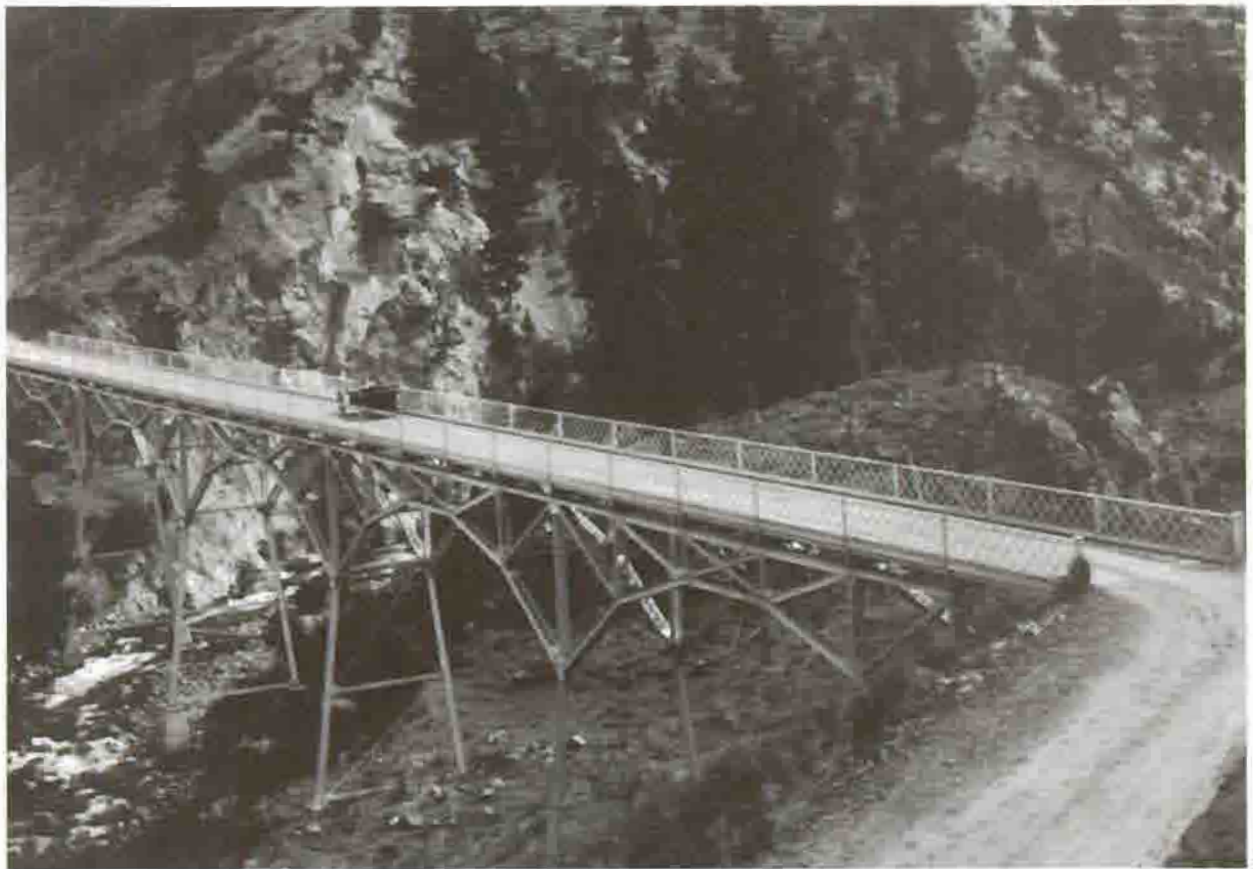
Gardner River Bridge, 1917 Courtesy Yellowstone National Park Archives
