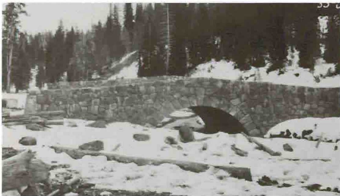
Cub Creek Bridge, 1929 Courtesy Yellowstone National Park Archives
