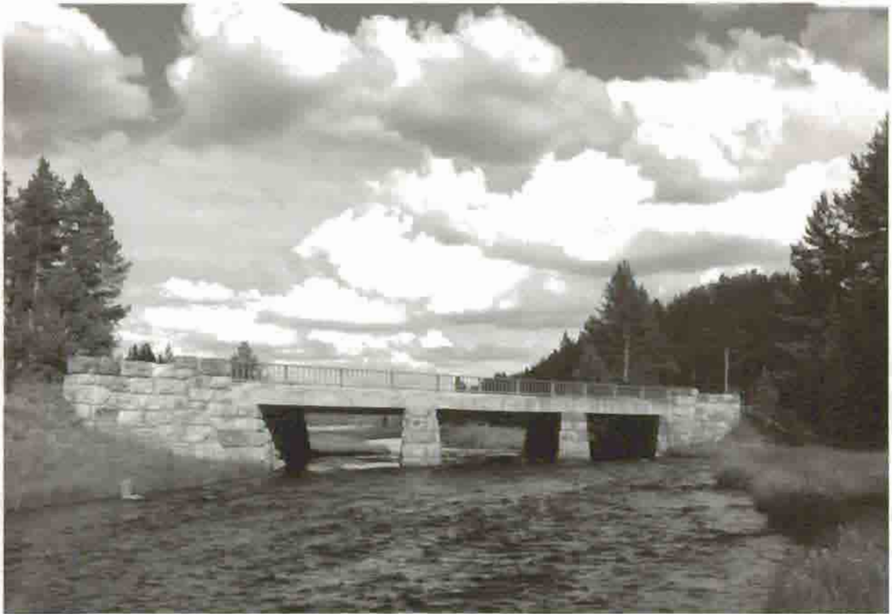
Nez Perce Creek Bridge, 1989 Courtesy Historic American Engineering Record, Jet Lowe, 1989
