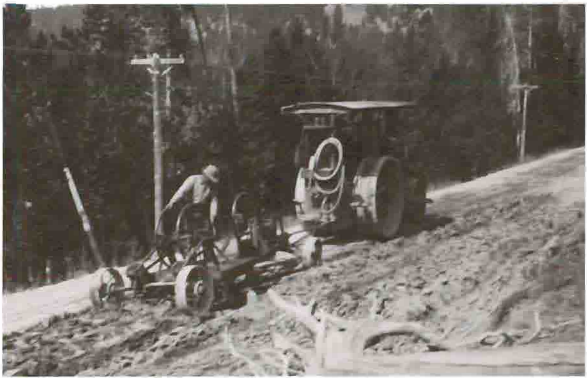
Steam Roller and Grader near Frying Pan Springs, 1917 Courtesy Yellowstone National Park Archives
