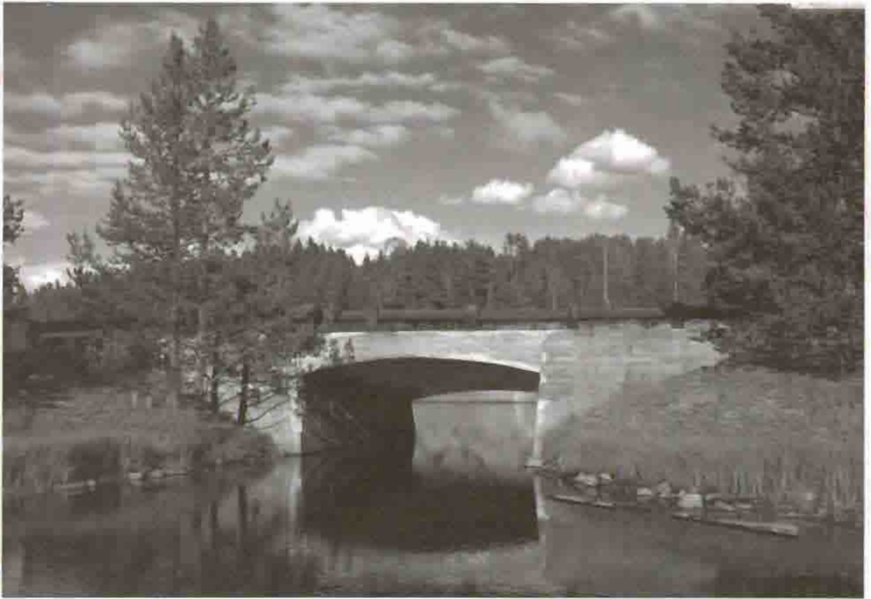
Otter Creek Bridge, 1989 Courtesy Historic American Engineering Record, Jet Lowe, 1989
