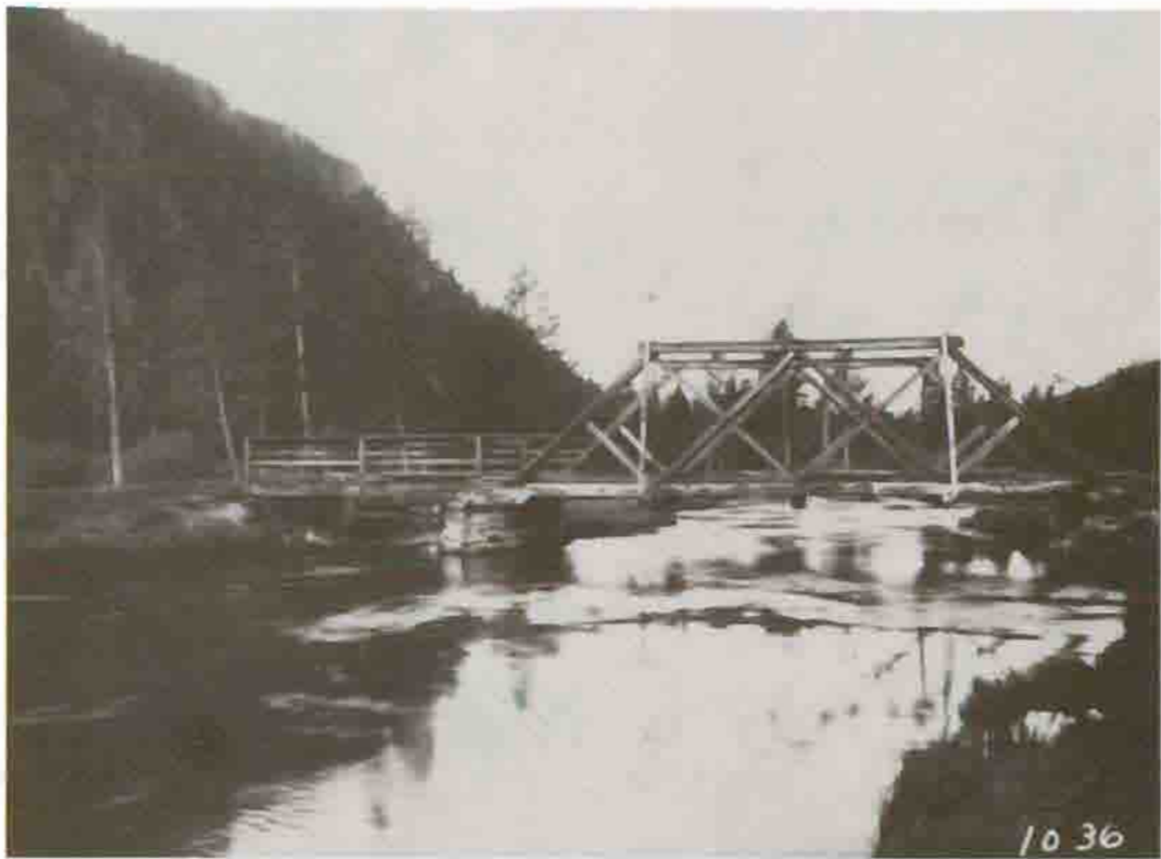
Gibbon River Bridge Near Madison Junction, 1912 Courtesy Yellowstone National Park Archives
