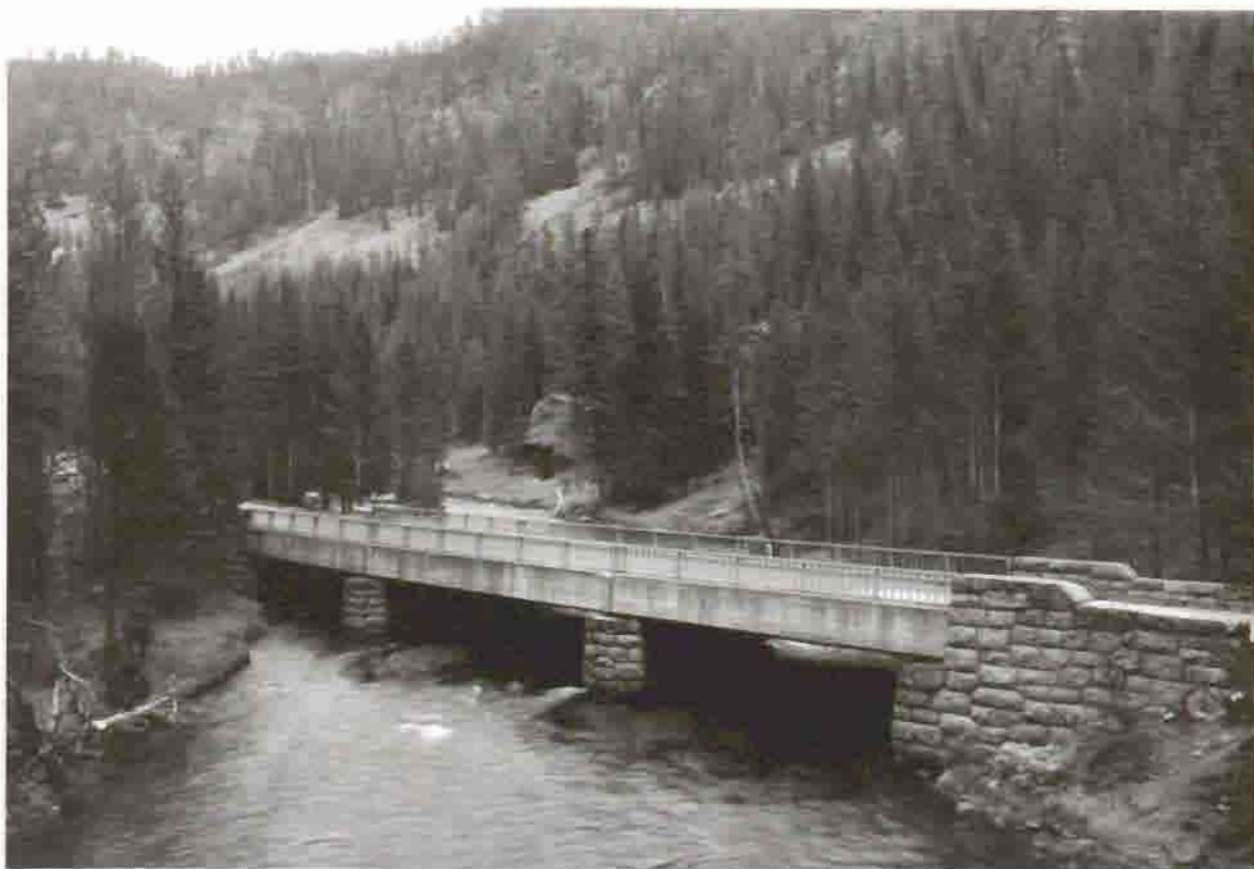
Gibbon River Bridge, 1989 Courtesy Historic American Engineering Record, Jet Lowe, 1989
