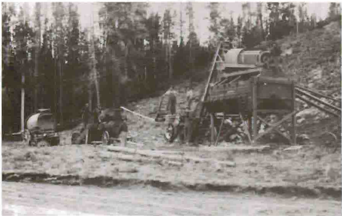
Rock Crusher, September, 1914 Courtesy Yellowstone National Park Archives
