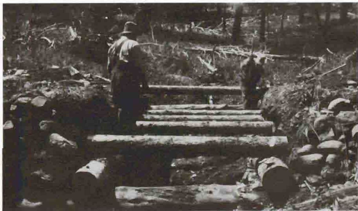
Culvert Construction on Cooke City Road, 1929 Courtesy Yellowstone National Park Archives
