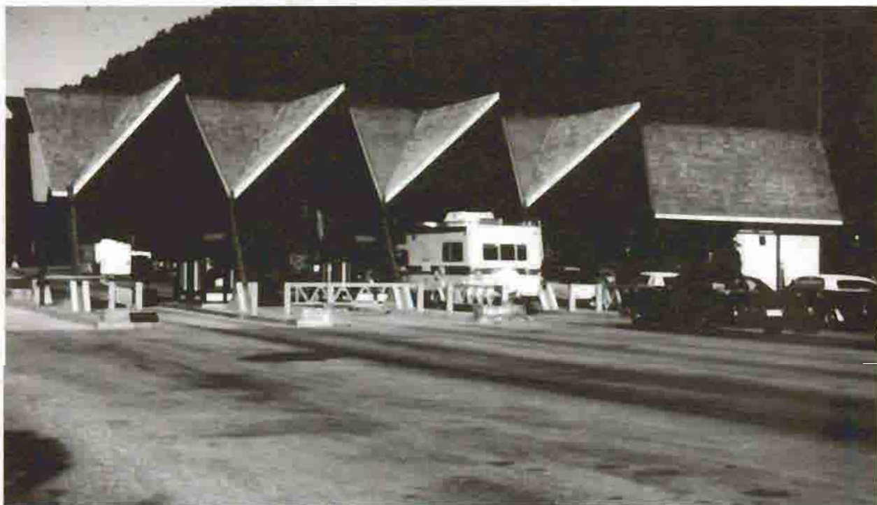
West Entrance Station, 1992 Courtesy Yellowstone National Park Archives
