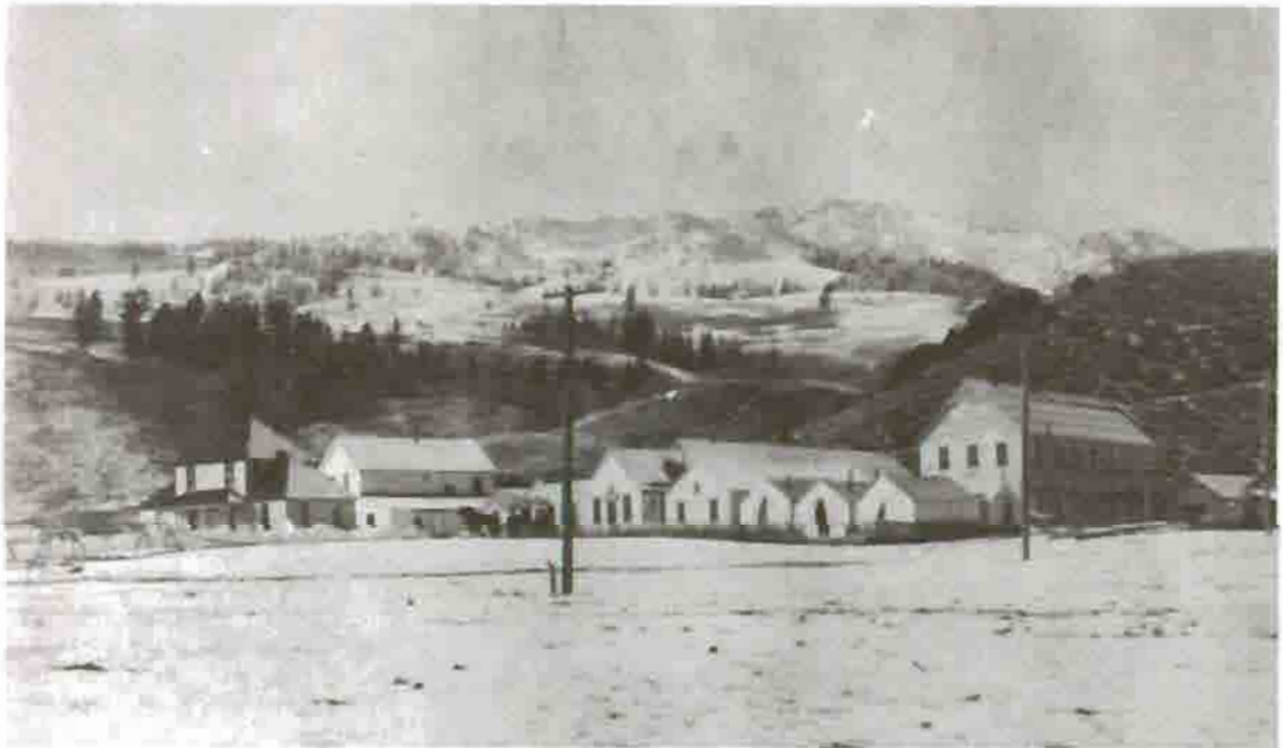
Old and New Engineers' Quarters at Mammoth Courtesy Yellowstone National Park Archives
