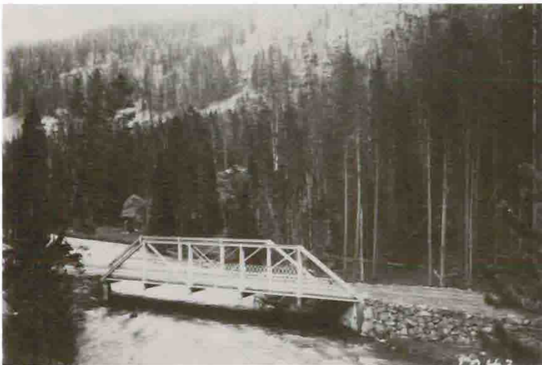
Gibbon River Bridge, 6 Milepost Norris Junction to Madison Junction, 1912 Courtesy Yellowstone National Park Archives
