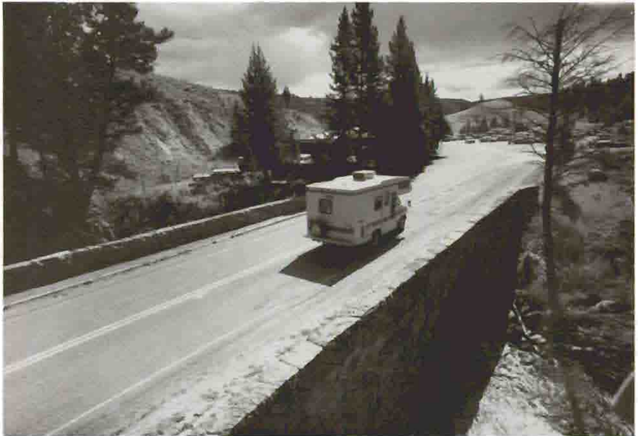
South Entrance Road Over Crawfish Creek Bridge, 1989 Courtesy Historic American Engineering Record, Jet Lowe
