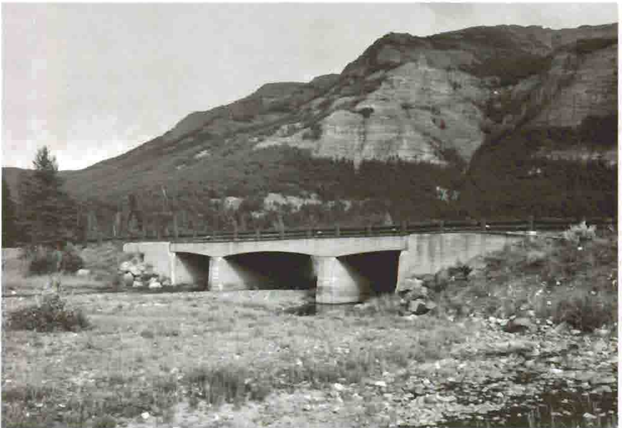
Pebble Creek Bridge, 1989 Courtesy Historic American Engineering Record, Jet Lowe, 1989
