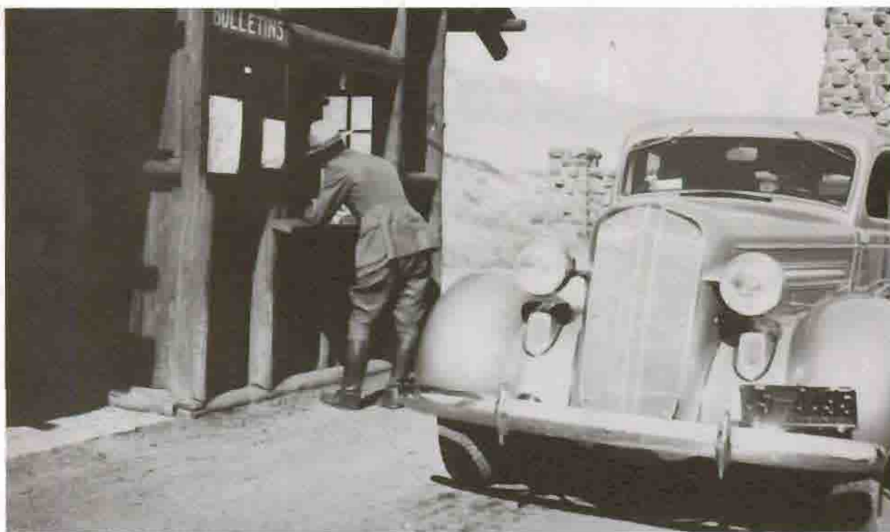
North Entrance Checking Station, 1936 Courtesy Yellowstone National Park Archives
