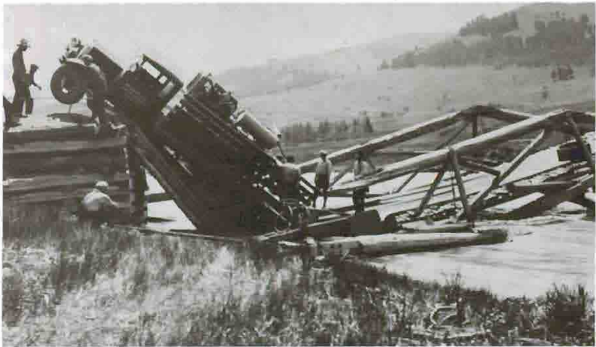
Lamar River Bridge Broken by Overload, 1932 Courtesy Yellowstone National Park Archives
