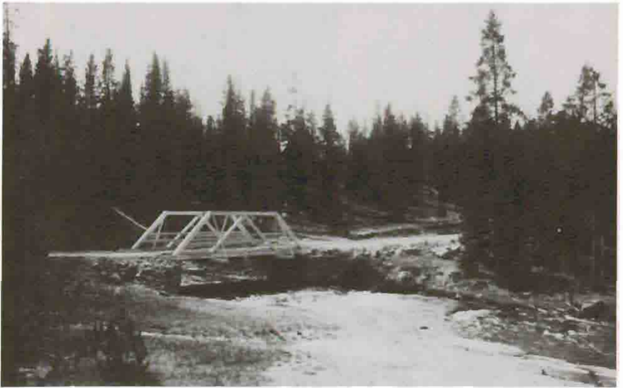
Firehole River Bridge, 1931 Courtesy Yellowstone National Park Archives
