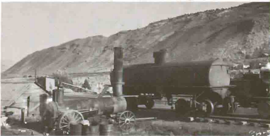
Improved Oil Heating Plant at Gardiner, July 26, 1927 Courtesy Yellowstone National Park Archives
