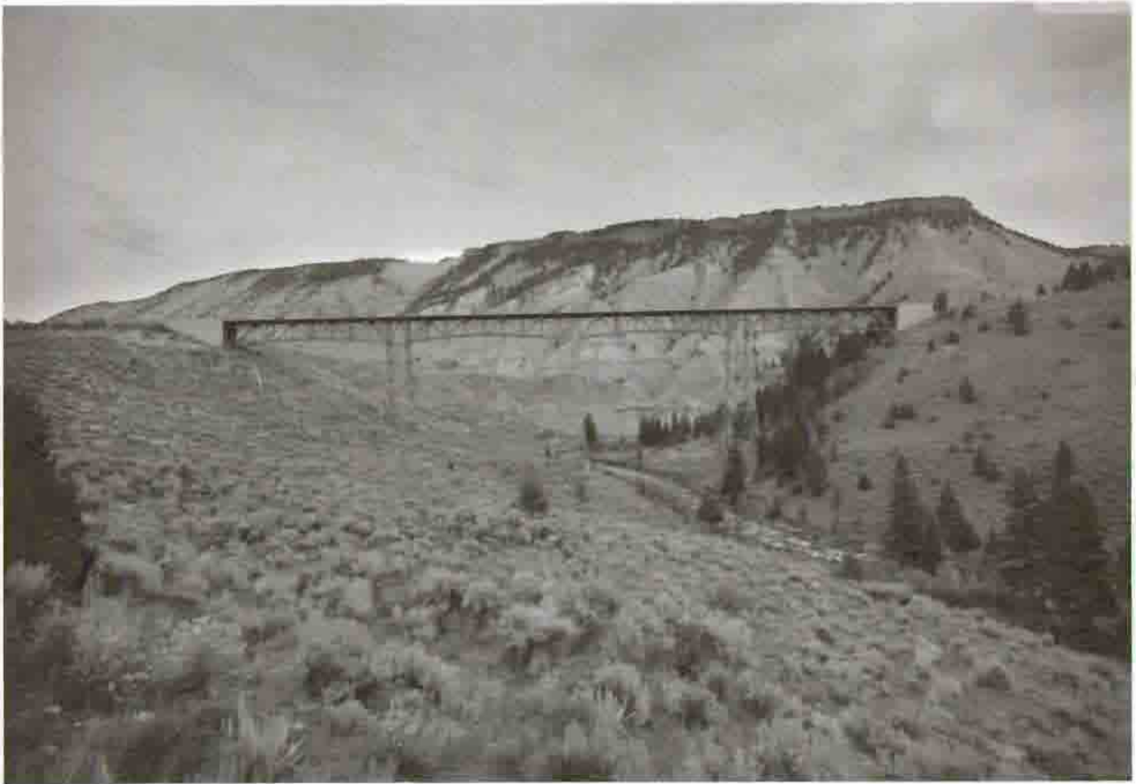
Gardner River Bridge, 1989 Courtesy Historic American Engineering Record, Jet Lowe, 1989
