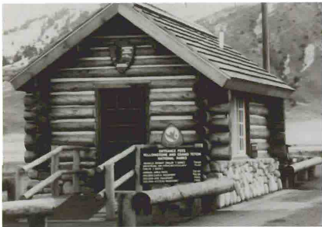
North Entrance Checking Station, 1990 Courtesy Yellowstone National Park Archives
