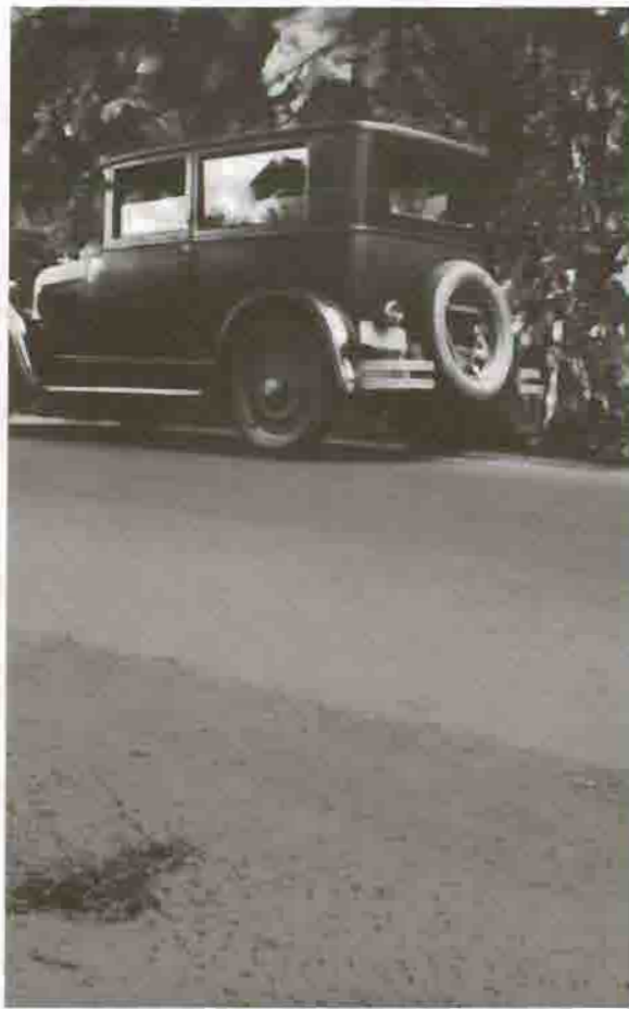
Showing Texture on Shoulder of California Oil Processed Road, March 1928 Courtesy Yellowstone National Park Archives
