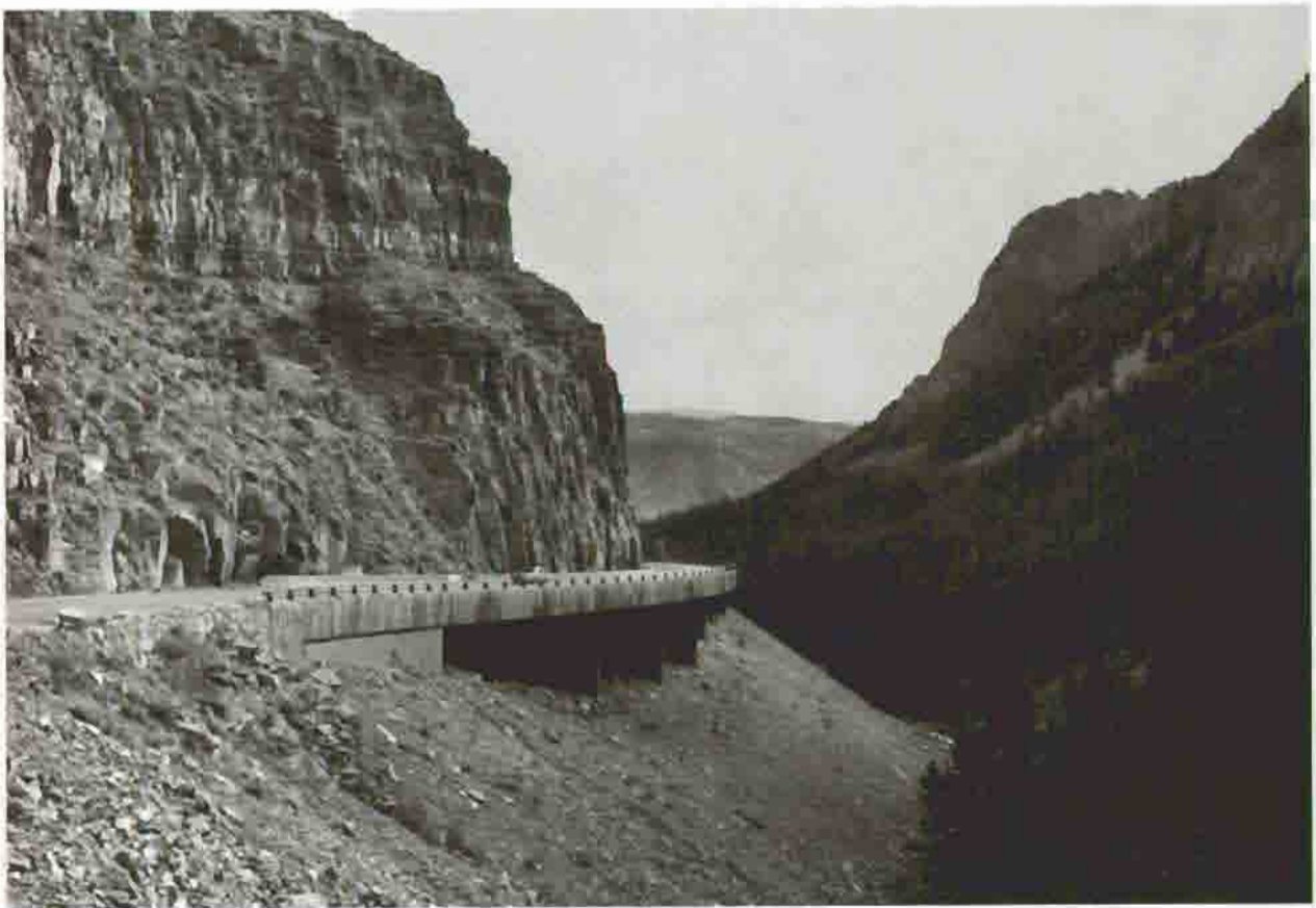
Golden Gate Viaduct, 1989 Courtesy Historic American Engineering Record, Jet Lowe, 1989
