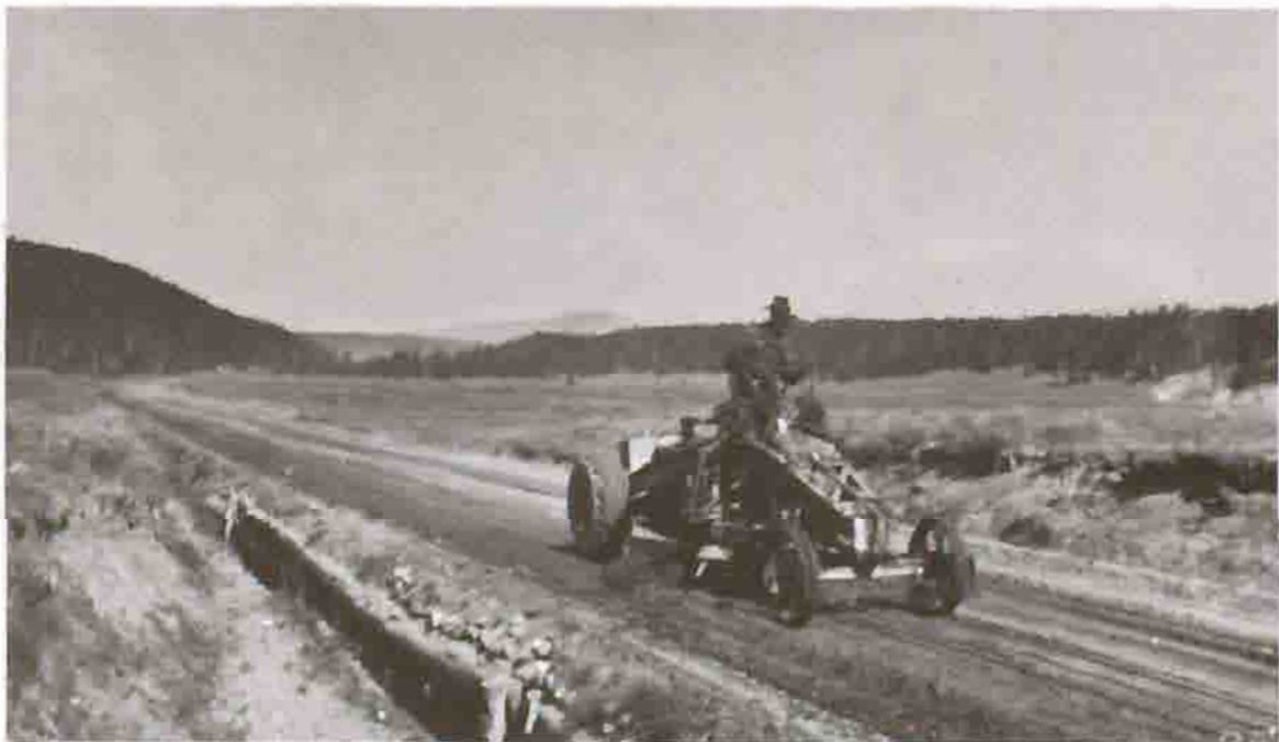
Experimental Sanding with High Clay Content, September 24, 1927 Courtesy Yellowstone National Park Archives
