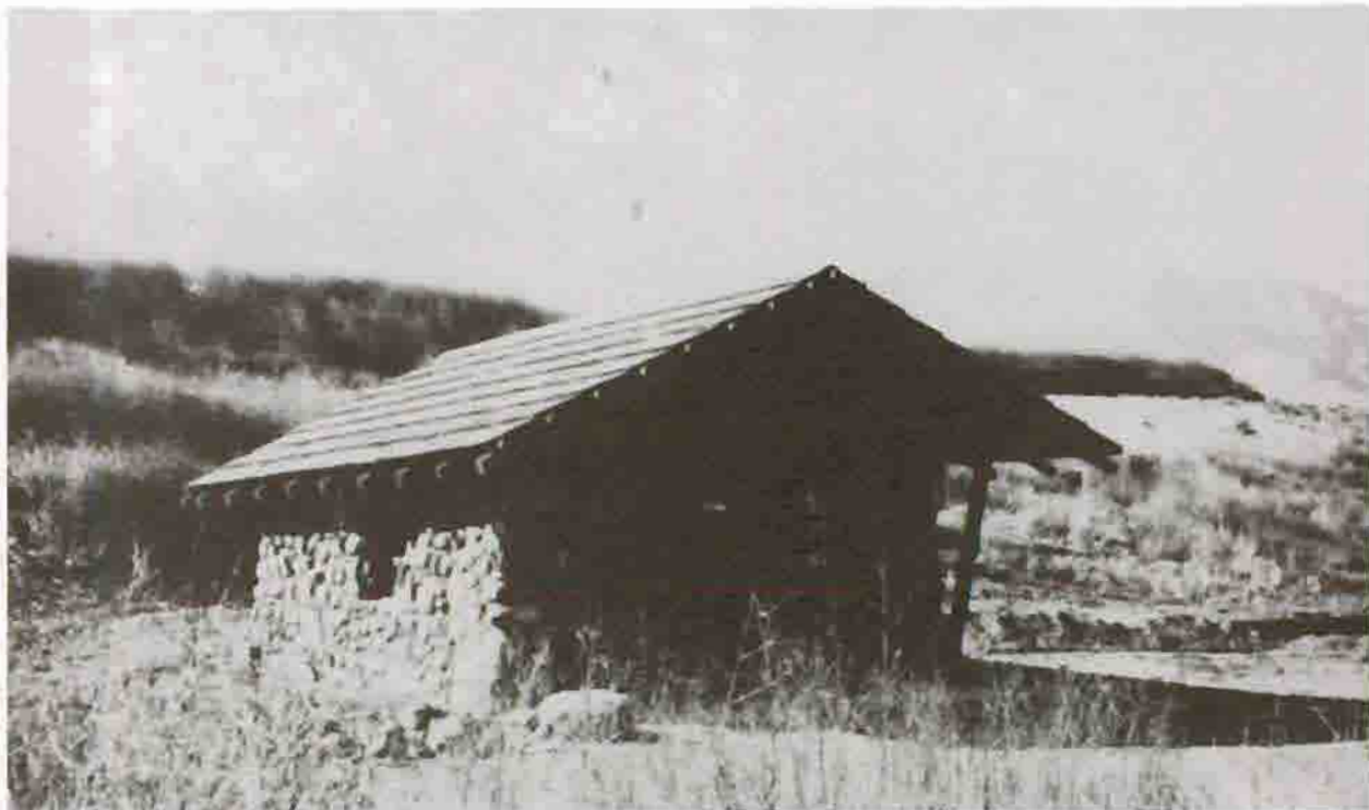
North Entrance Checking Station, 1922 Courtesy Yellowstone National Park Archives
