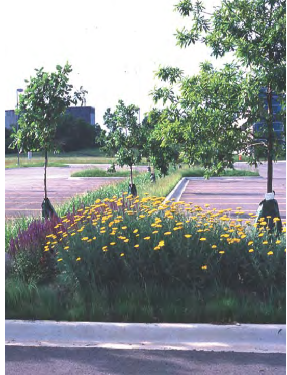
bioswale in a parking lot (Tellabs, Naperville, IL) (Conservation Design Forum)
