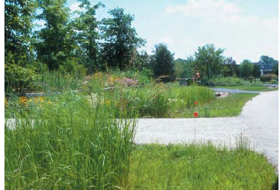
vegetated swales planted with native grasses and forb along the street
