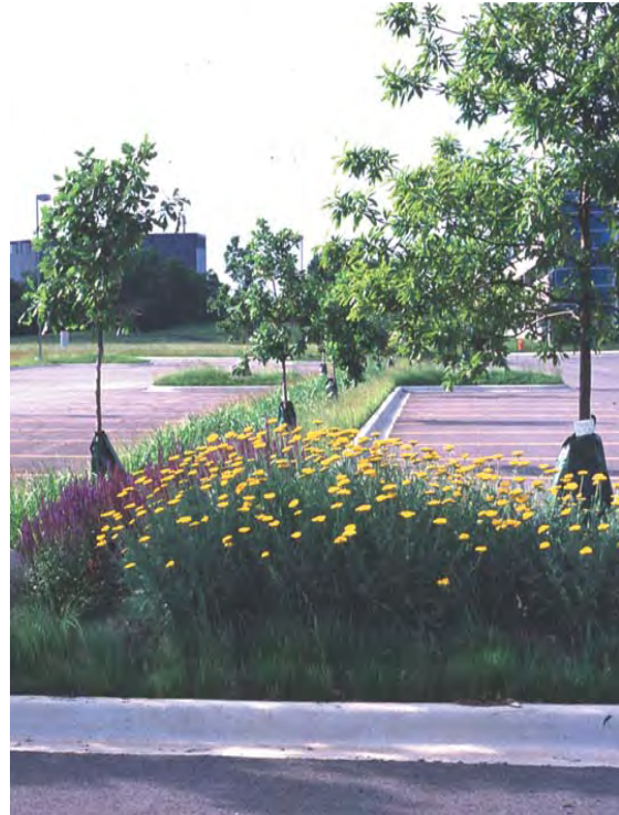
bioswale in a parking lot (Tellabs, Naperville, IL) (Conservation Design Forum)
