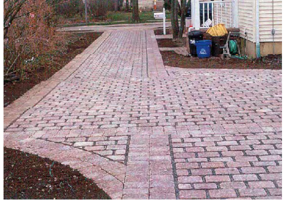
porous pavement employed in driveway
