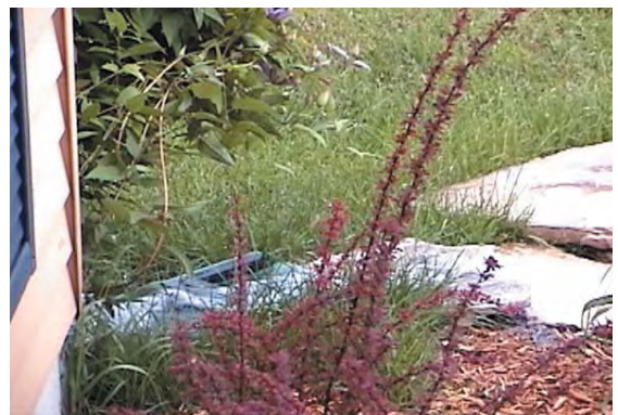
roof top down spout connects to rainwater garden (Glen Ellen, IL)
