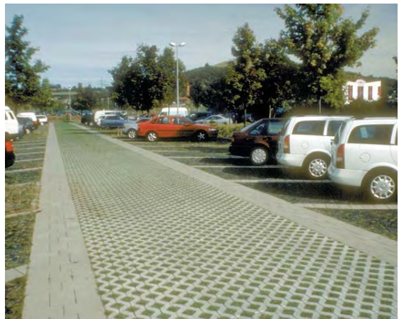
porous pavement in parking lot
