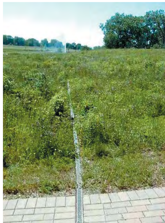
filter strips/level spreader
