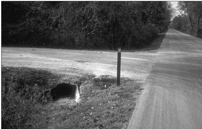
Photo 7. One of the responses to natural features evident at the park is the use of culverts and swales to carry stormwater away from the Tour Road.
