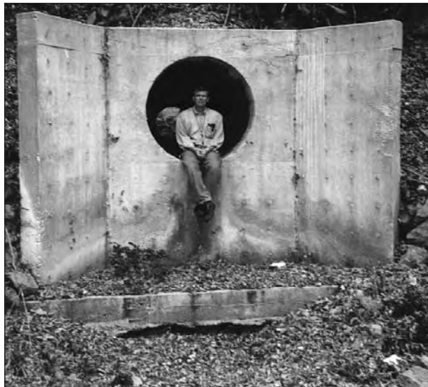
Photo 55. This large concrete culvert conveys stormwater from Manley Branch beneath the former Missouri-Pacific Railroad grade. The volume and velocity of the flow is currently undercutting the structure.
