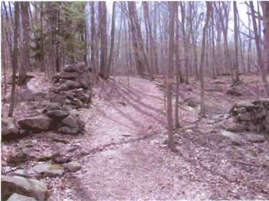
View west of stone lined ditch diverting water from a small stream (right side of path) across the footpath leading to Weir Pond and into an adjacent wetland, 2003 (OCLP).
