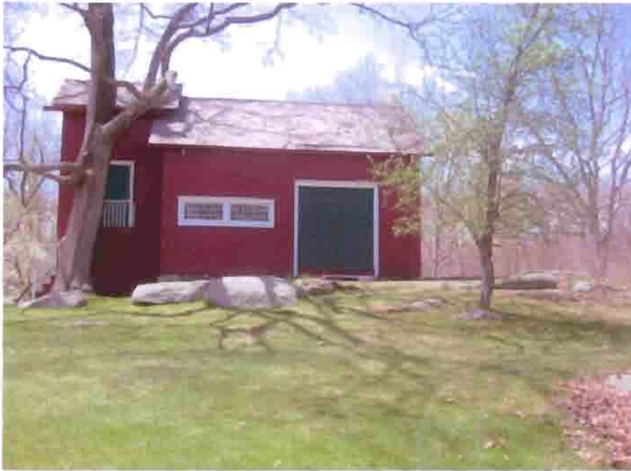
View north of the Weir studio, 2003 (OCLP).
