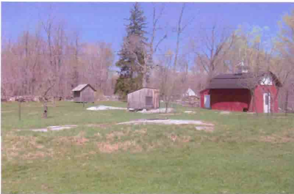
View north (left to right) of the Weir/Young corn crib, animal shelter, and ice house, 2003 (OCLP).
