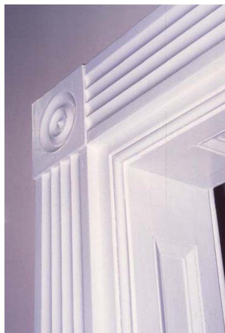
Figure C – 21 Fluted door casing
