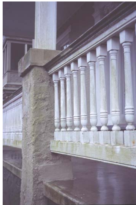
Figure C – 13 Front porch balustrade
