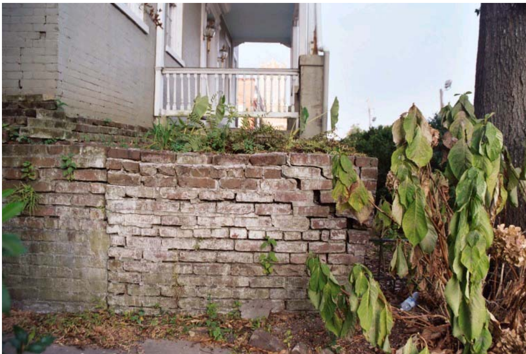
Figure 4 Retaining wall at northeast corner
