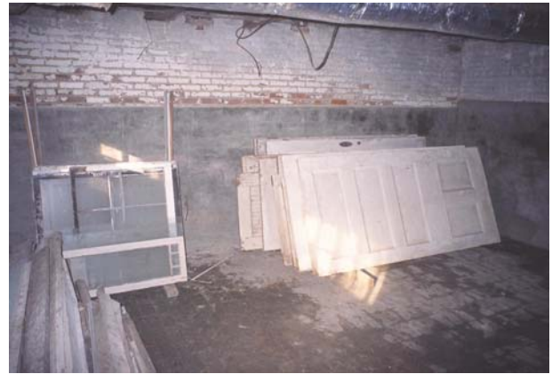
Figure C - 16 Original doors in storage in Room 001
