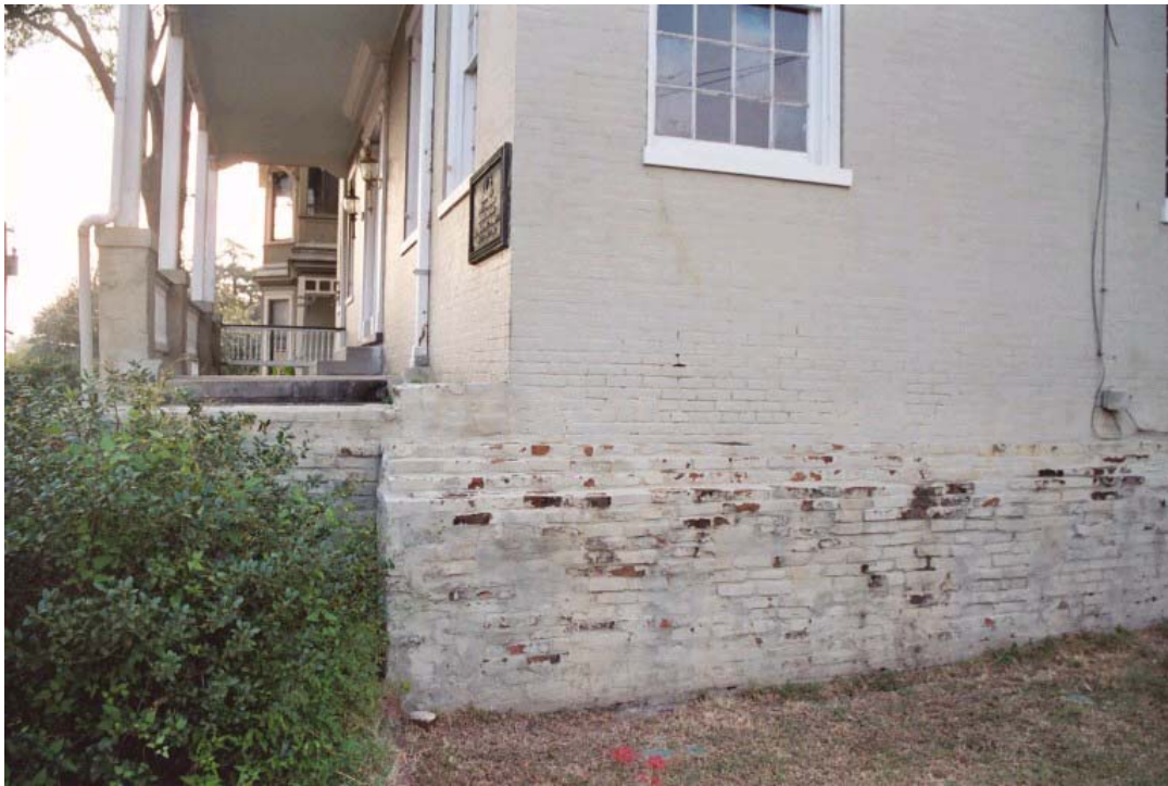
Figure 3 Retaining wall at northwest corner
