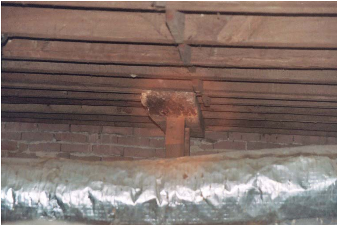
Figure 2 Added supports under northeast room (Room 101)
