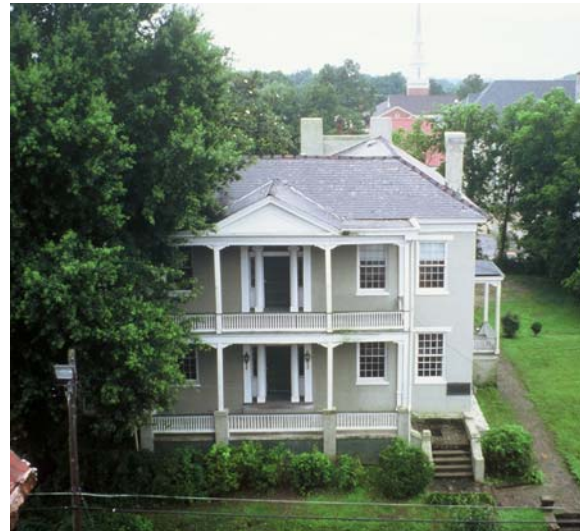
Figure B - 1 Front view of the house
