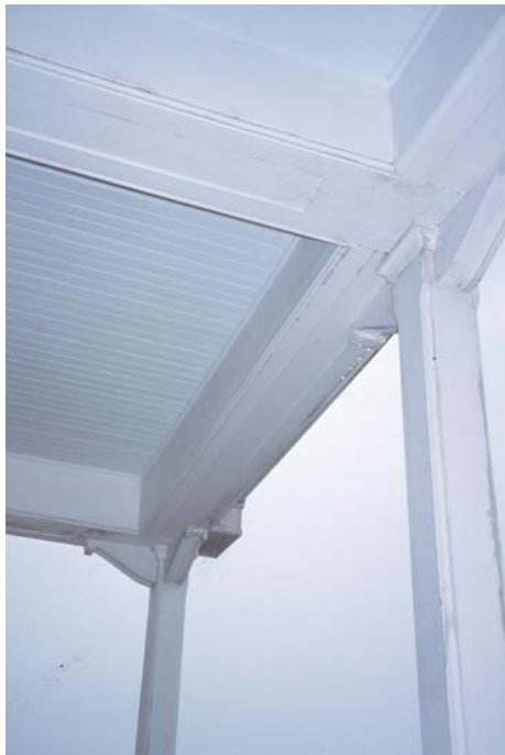
Figure C – 14 Construction of the front porch
