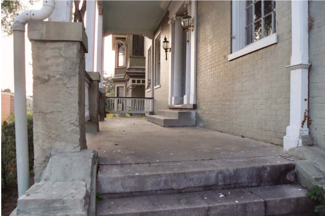
Figure 5 Concrete front porch
