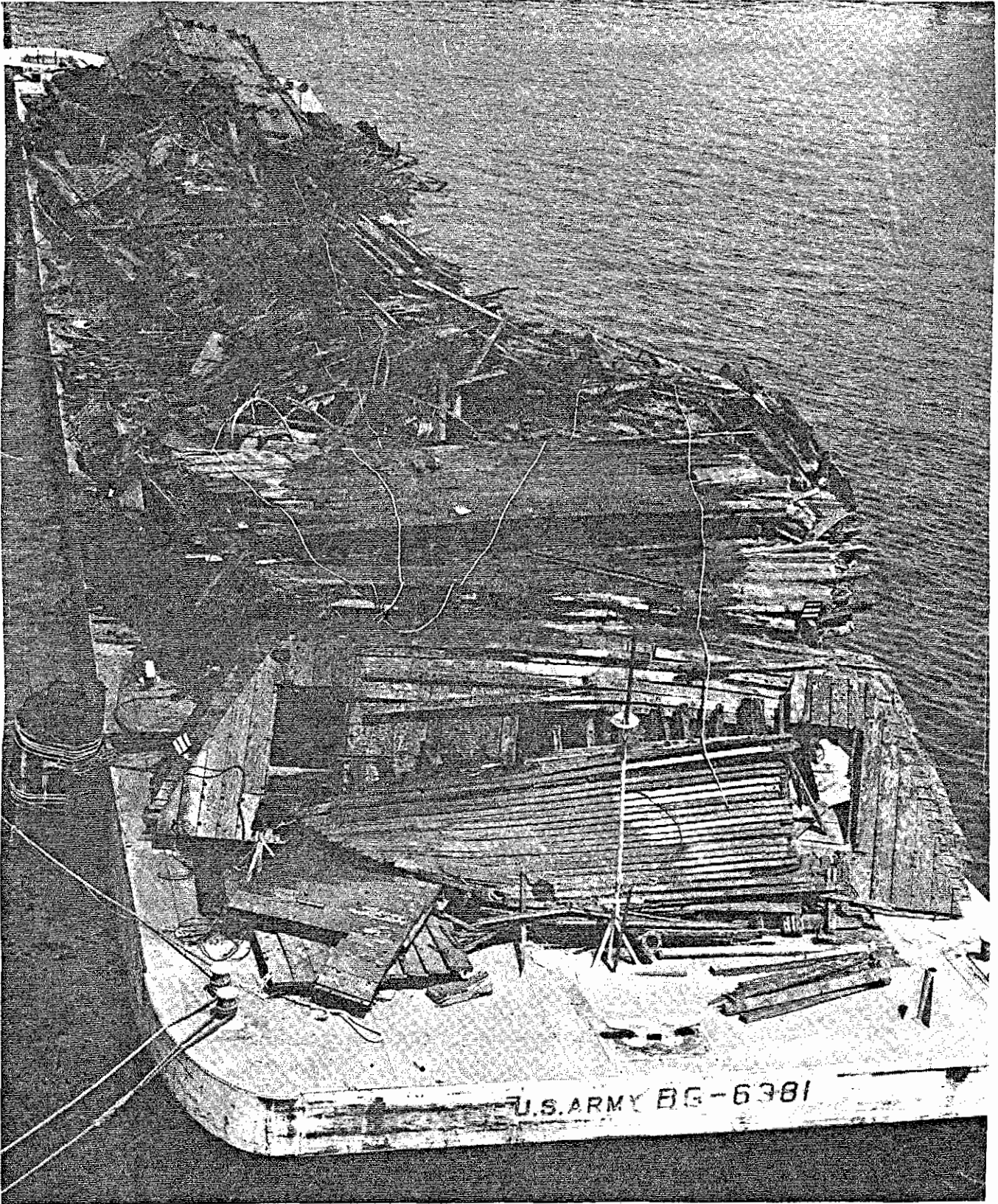
Figure 4: Cairo fabric upon arrival at Pascagoula in 1965. The undocumented dismantling of many components that later magnified the difficulty of an accurate restoration had not yet begun. Mississippi Agricultural and Industry Board photo.
