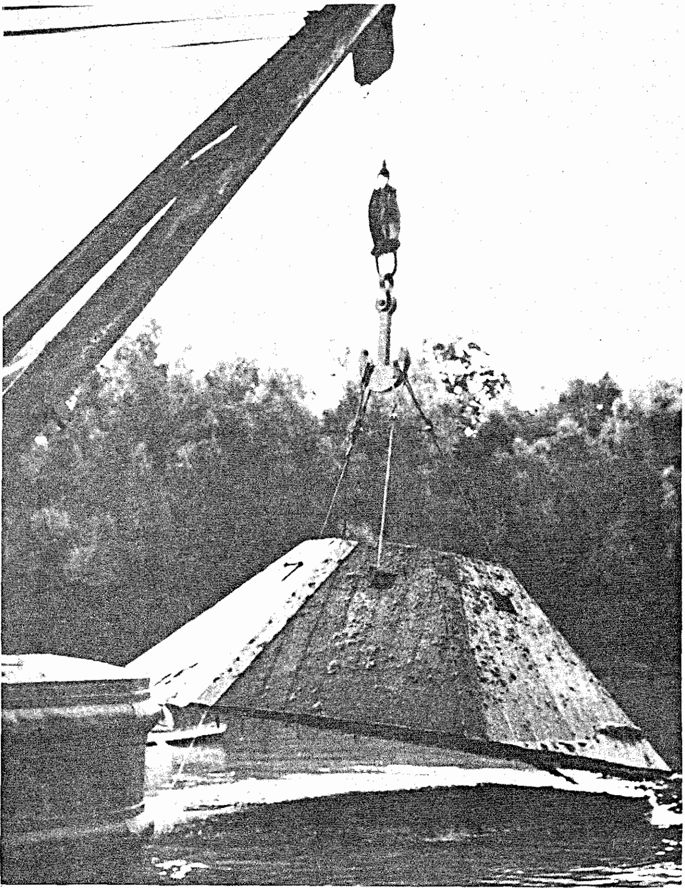
Figure 1: The pilothouse as it appeared immediately after removal from the hurricane deck in September 1960. Allowed to deteriorate since this photo, now only the armor sheathing survives. Mississippi Agricultural and Industry Board photo.
