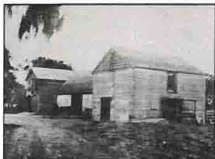
Figure 14. From left: carriage house, older tabby brick portion of barn, and later nineteenth-century addition.
