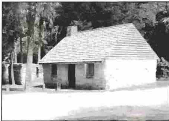
Figure 17. Restored Cabin E1.
