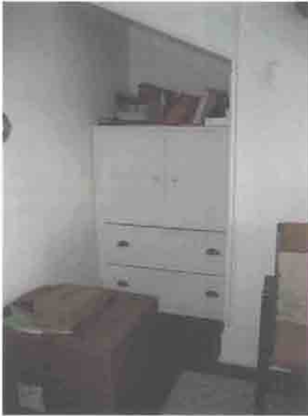
Figure 2.80. Room 306, recess with built-in wood cabinet.
