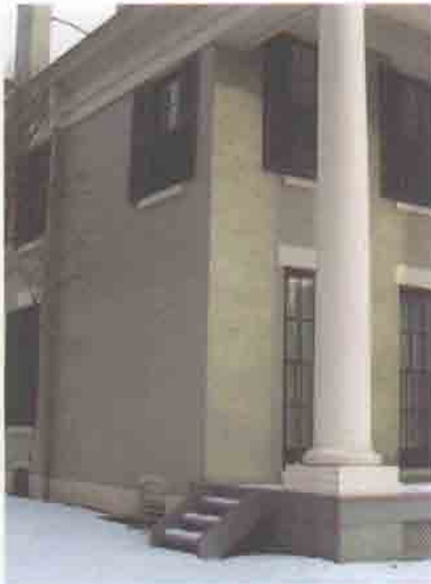
Figure 2.6. Northwest corner of original building.
