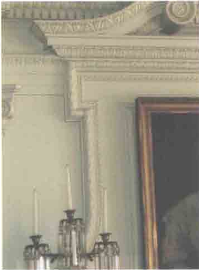
Figure 2.42. Room 108 (Dining Room), ornamental moldings of mantelpiece.
