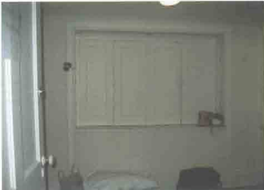
Figure 2.75. Room 302 (Hall), south- wall linen closet.
