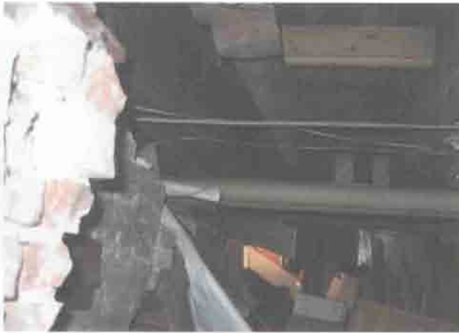
Figure 2.24. Room 001a (central brick furnace chamber), interior.
