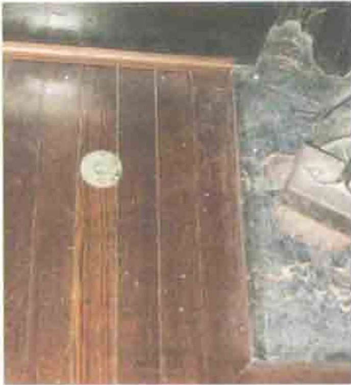
Figure 2.39. Room 107 (Living Room), unidentified floor feature.
