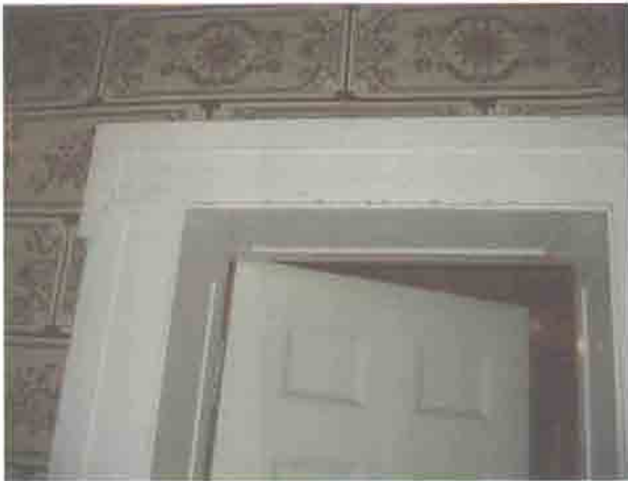
Figure 2.55. Room 201 (Second-Story Stair Hall), pre-1938 doorway.
