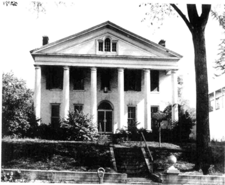
Figure 1.34. West facade, circa 1965.
