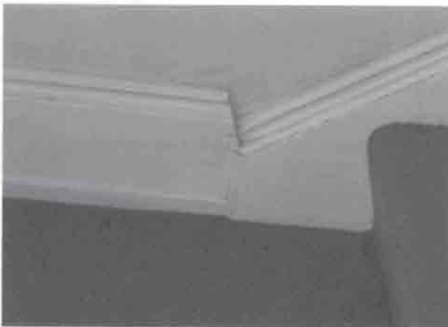
Figure 2.73. Room 301 (North Staircase), baseboard.
