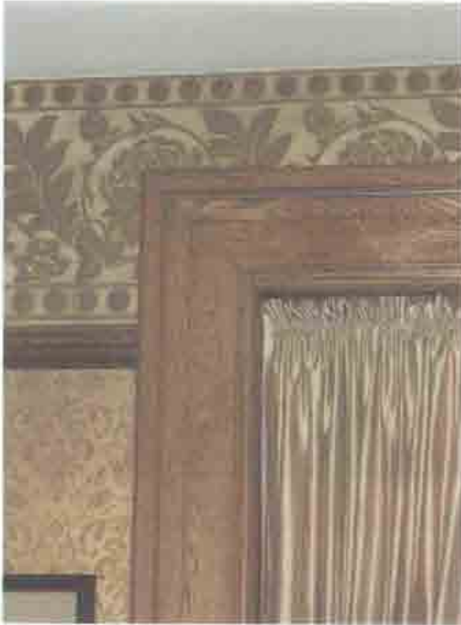
Figure 2.34. Room 104 (Library), molded oak casing.
