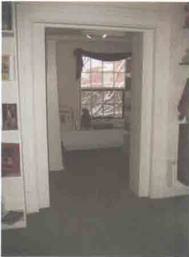
Figure 2.65. Room 208, north wall, 1896 window converted to doorway in 1938.
