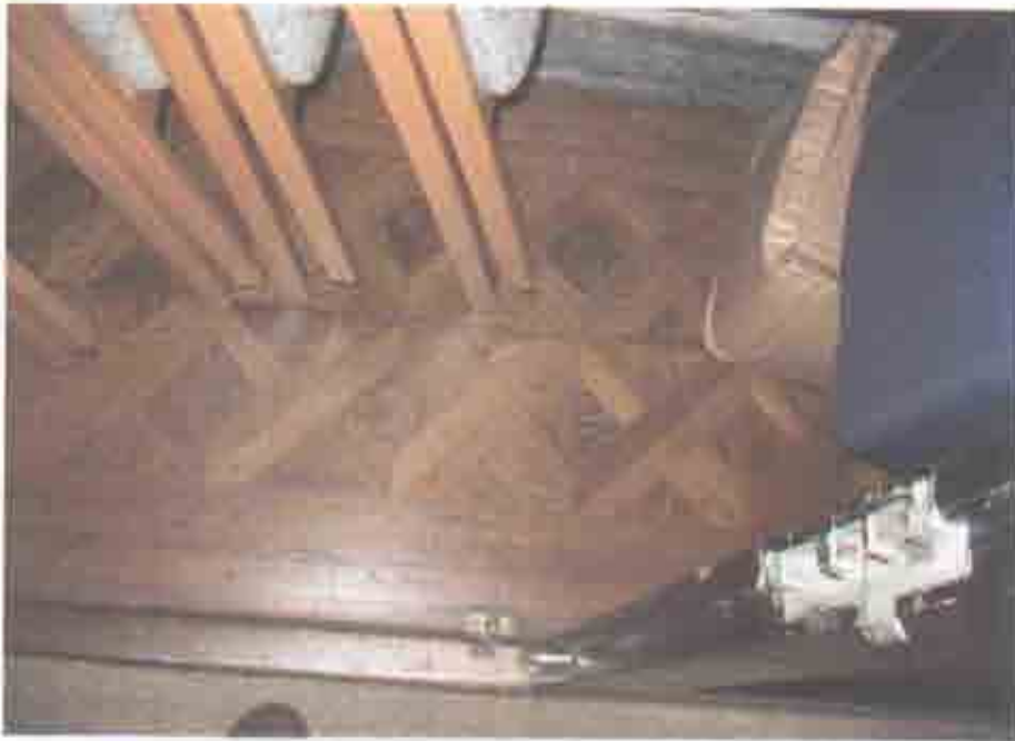
Figure 2.30. Room 101 (Vestibule), ca.-1885 parquet flooring.
