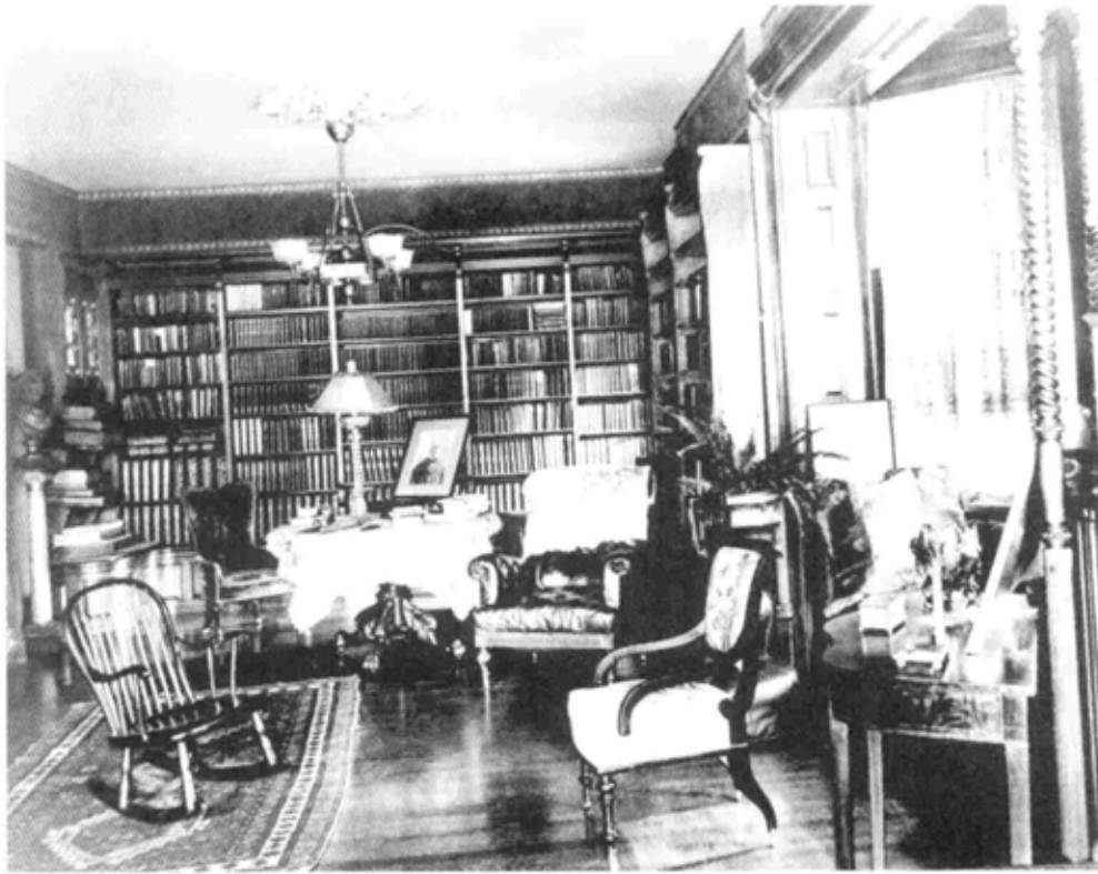
Figure 1.40. Library (room 104), looking east, fall 1901.
