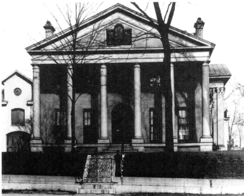
Figure 1.30. West façade, circa 1930.
