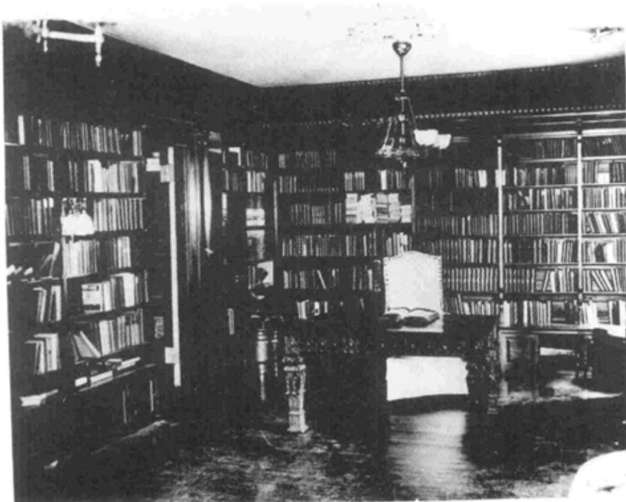
Figure 1.48. Library (room 104), looking east, circa 1934.
