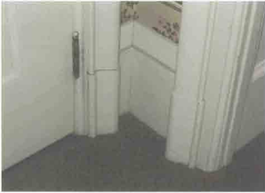
Figure 2.32. Room 102 (Front Hall), ogee casing and plinth blocks.
