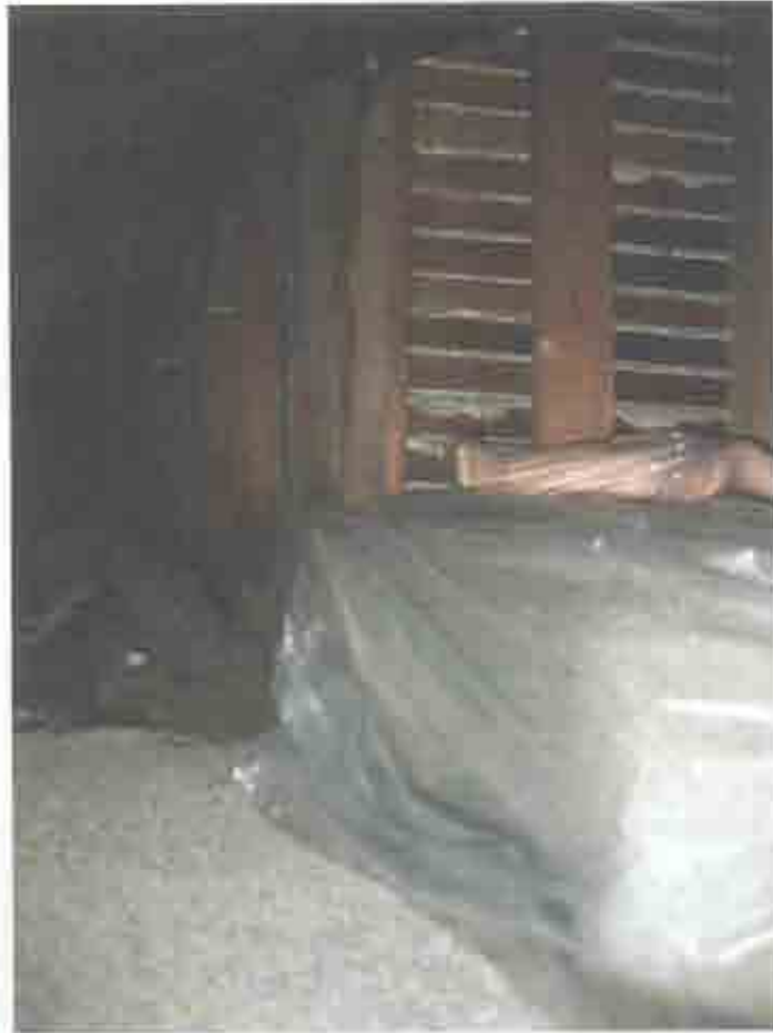
Figure 2.71. Room 308a, looking west toward dormer cheek wall.
