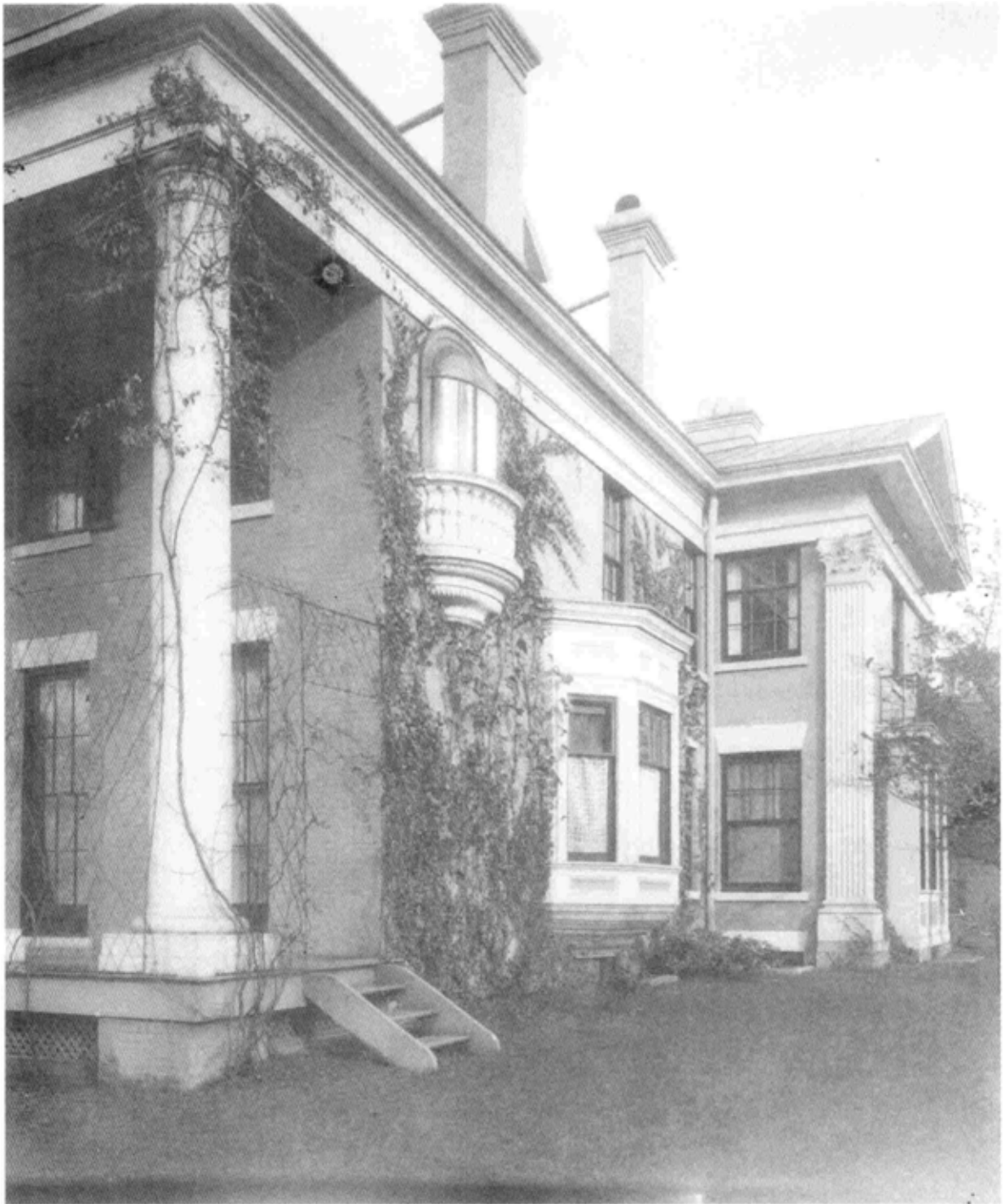
Figure 1.27. Southwest corner, showing 1865 portico, 1885 bay window, 1891 oriel window, and 1896 rear addition, circa 1921.
