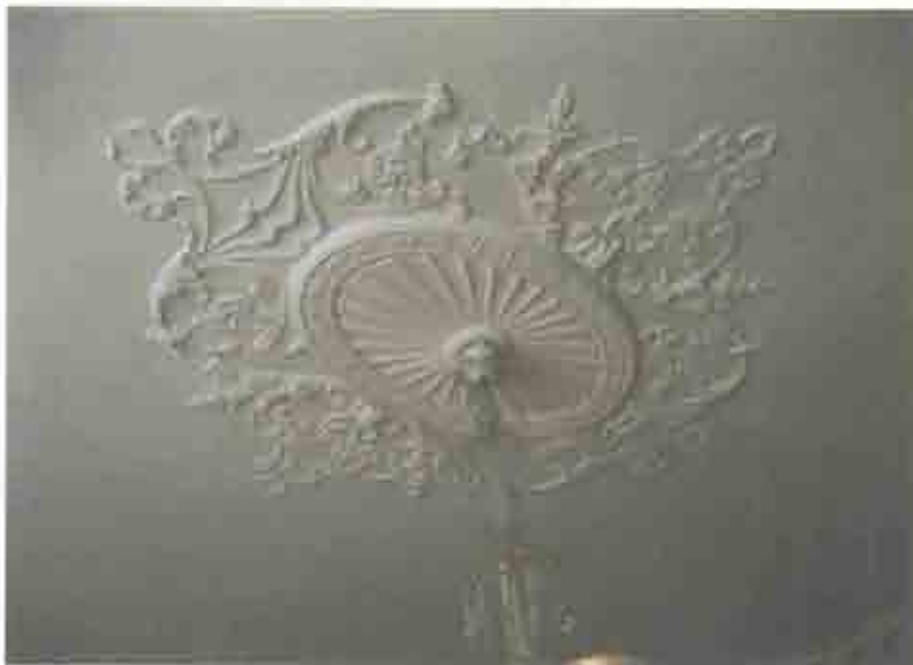
Figure 2.45. Room 108 (Dining Room), ceiling medallion.
