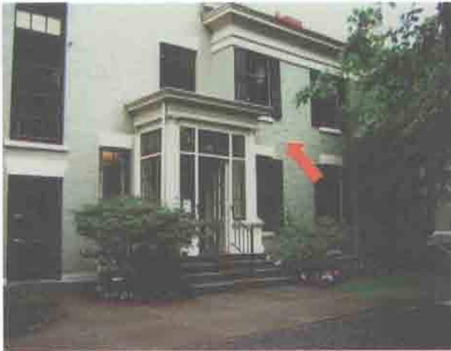
Figure 2.13. North elevation, location of brickwork scars from formerly attached barracks building.
