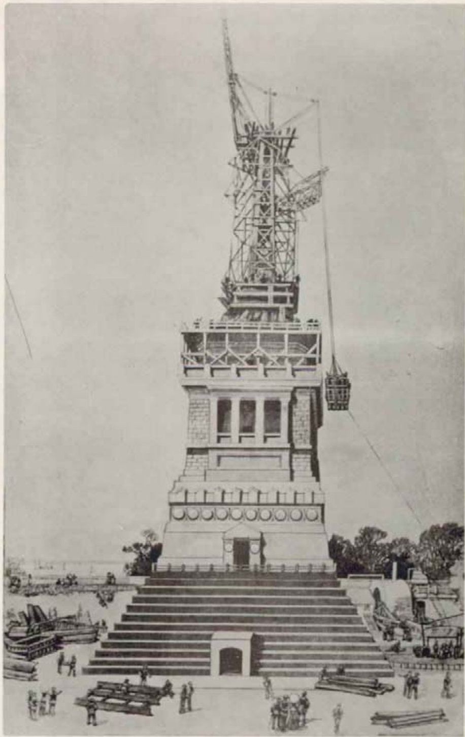
Construction of the pedestal, early 1886. From a sketch in Leslie's Weekly .
