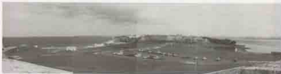
Figure 15. Composite photograph, East View, 1971 (View 1). Vista from el Morro showing parking lot, parallel parking along the roads, trees in Parcel B, and the general open character of the site. Photography by Richard C. Crismon.
