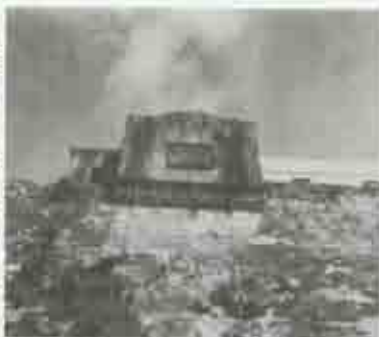
Figure 49. Curtain wall between la Concepción and las Palmas Bastion with Cristo Chapel above. (Photo by N. Crismon, 1990.)
