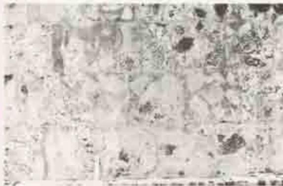
Figure 6. Cast composite stone of merlon on north wall of Santa Barbara Battery. Photo by J. Jacob, 1988.
