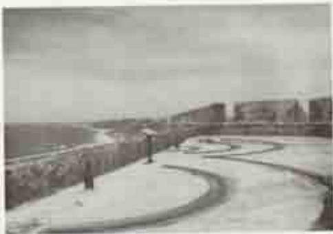
Figure 25. Two 1850's gun emplacements on Ochon Bastion. (Photo by E.B. Oliver, 1986.)
