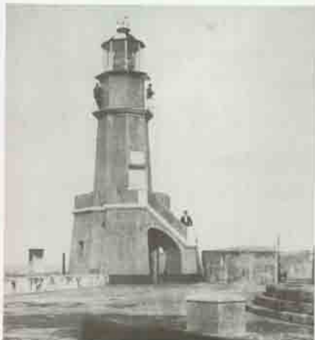
Figure 46. First American lighthouse, built on the base of the damaged Spanish lighthouse. (National Archives, 24-10-42-13B.)
