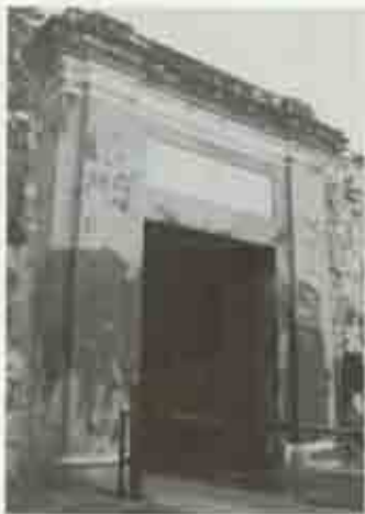
Figure 46. West elevation of San Juan Gate. (Photo by S. Crissom, 1996.)
