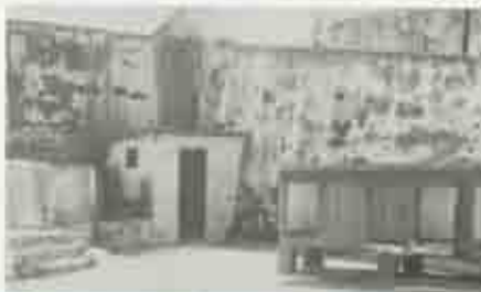
Figure 41. World War II latrine, demolished. (J. Boucher, HNS, 1960.)
