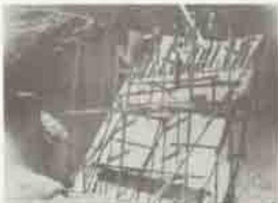
Figure 35. Reconstructed scarp wall, Santo Domingo Bastion, May 1938. (NARS NPS Archives.)
