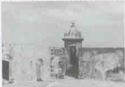
Figure 61. Sentry Box at San Antonio Bastion. (Photo by R. Crisson, 1990.)
