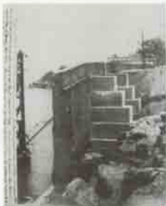
Figure 31. New concrete counterforts for the curtain wall between Santa Elena and San Agustín Bastions, 1938. (SAJU NMS Archives.)
