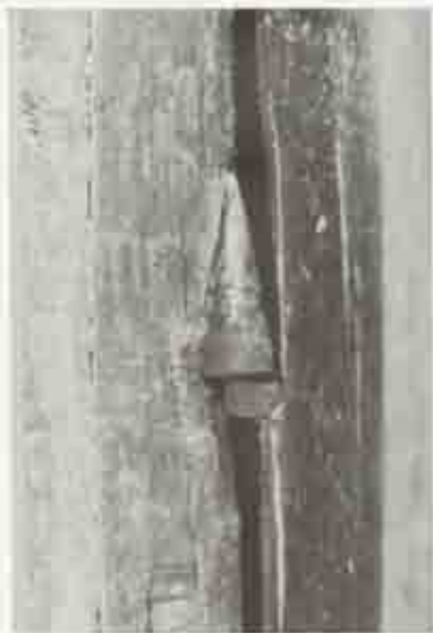
Figure 19. Capachico hinge from shutter on Troops' Quarters, San Cristóbal. Photo by J. Jacob, 1987.
