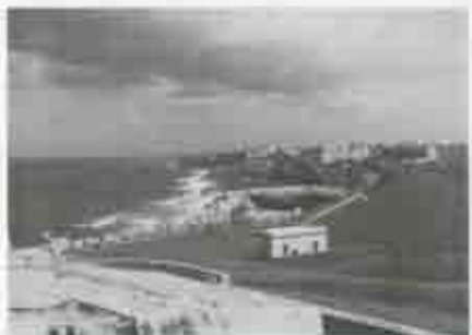
Figure 60. North walls with San Antonio Bastion in foreground, cemetery below. (Photo by W. Crissan, 1990.)
