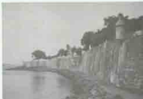
Figure 44. San Juan Gate to San Agustin Section at far left. (Photo by R. Crismon, 1990.)
