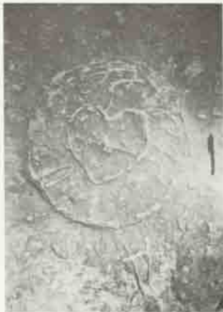
Figure 15. Floor of small chamber adjacent to the passageway to the magazine under Austria Bastion, el Morro. (NARS photo, 1942.)
