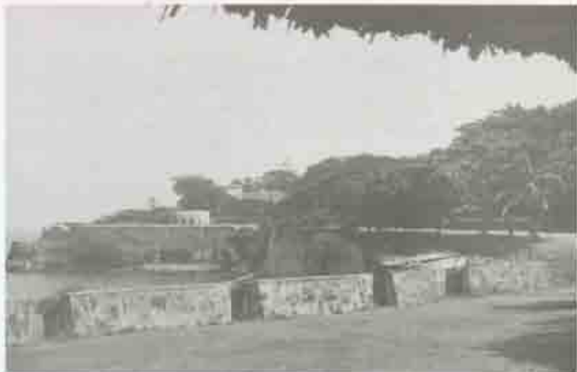
Figure 27. Condition of the west city wall in vicinity of the San Agustín (foreground) and Santa Elena (background) bastions, ca. 1960. (K&JH VHS Archives.)
