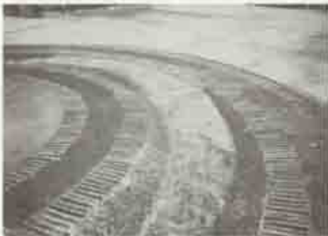
Figure 34. Tracks for an 1815's gun emplacement; note groove in dark stone from the iron rail. (Photo by S.R. Cliver, 1988.)
