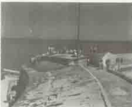
Figure 40. World War II concrete signal platform on top of the high wall, existing. (S&W HNS files.)
