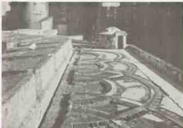
Figure 27. Tracks for 1860's gun emplacements on Santa Barbara Bastion. (J. Soucher, 2532, 1960.)
