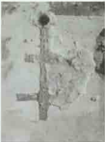
Figure 30. Double cross imprint in the casemate wall plaster, possibly from a bracket. (G.S. Cliver, 1990.)
