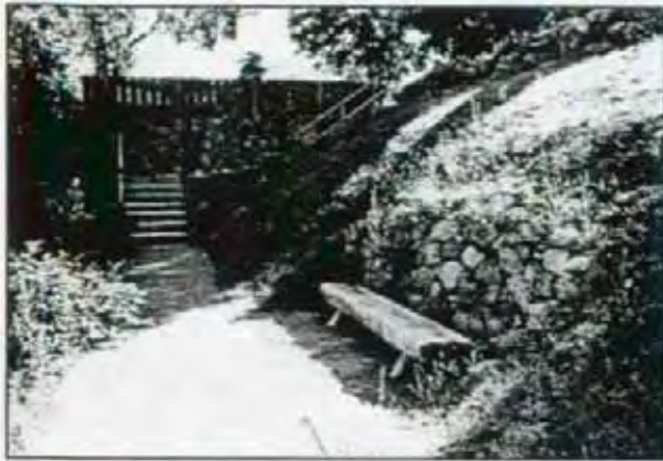
Figure 4.11. View of the south stairway leading to the lower industrial area. Stair lifts have been proposed here to provide persons with special needs with better access to the lower industrial area and eliminate the current system of using golf carts. (OCLP 2002)
