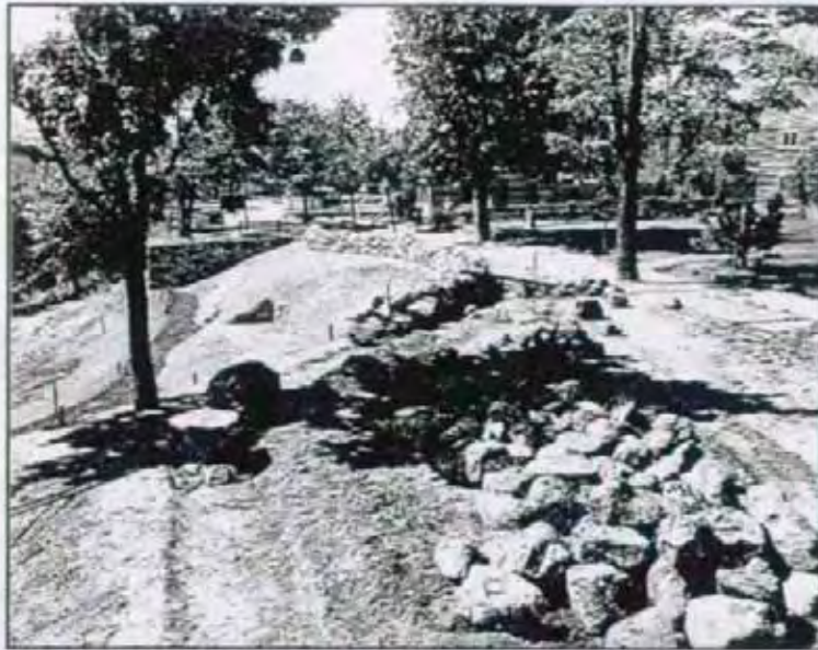
Figure 3.12. View south in 1954 of construction of the free-standing stone wall, the alignment of which likely corresponds to the westward extent of archeological investigations on the hillside. The slope has been graded, but it is unclear if this is intended to reflect the seventeenth-century contours of the bluff. By opening day, the sidewalk along Central Street was removed, but the path leading to the Iron Works House and barn, along the former driveway, remained. The extant north stairway to the industrial complex would be built next to the tree on the left. (SAIR #1169)
