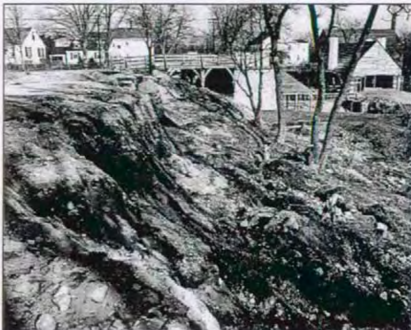
Figure 3.10. In this view looking north in 1953, the comparatively finished setting of the reconstructed iron works plant contrasts with archeological work underway along the hillside. The path and bridge between blast furnace and forge is in place. The two trees on the hillside closest to the camera will eventually be removed for the hillside path. (SAIR #1062)
