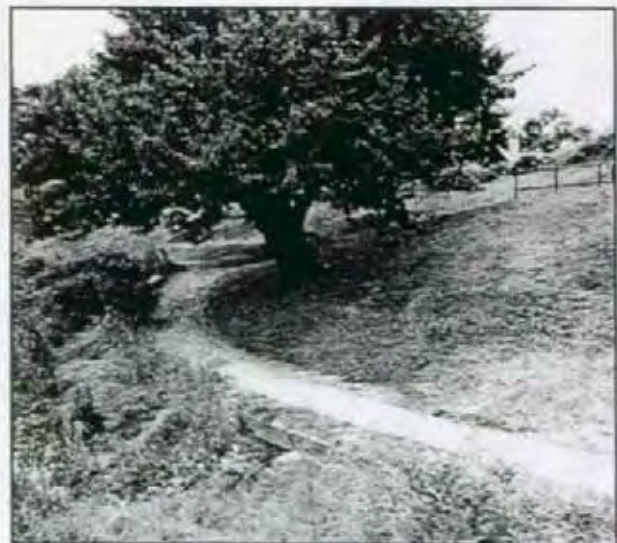
Figure 4.14. This segment of the path leading from the upper terrace to the industrial complex does not meet American with Disabilities Act requirements. Steep portions such as this, and in other areas of the industrial area, are chronically plagued with erosion problems that make for hazardous walking surfaces. (OCLP 2002)
