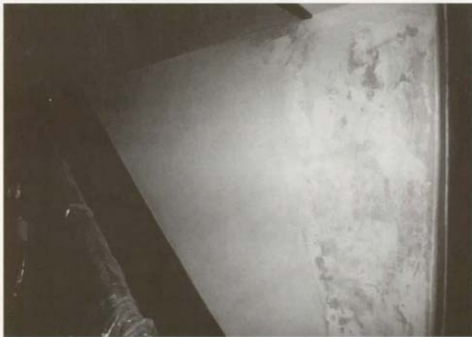
Second Floor Rear Hall Stairway: After Replastering
