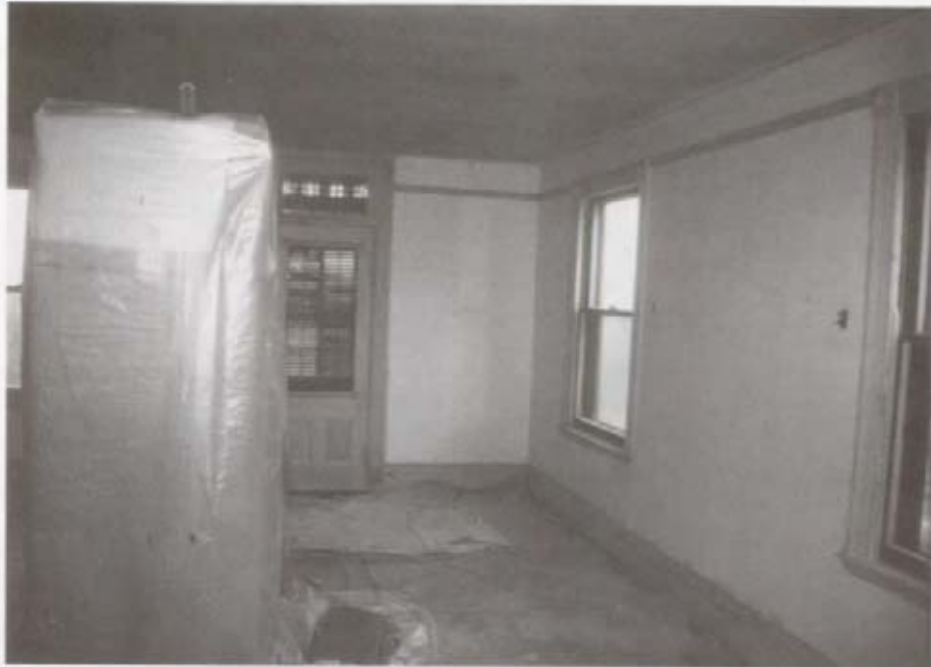
Mother's Room: During Restoration (wallpaper removed, picture molding lowered).
