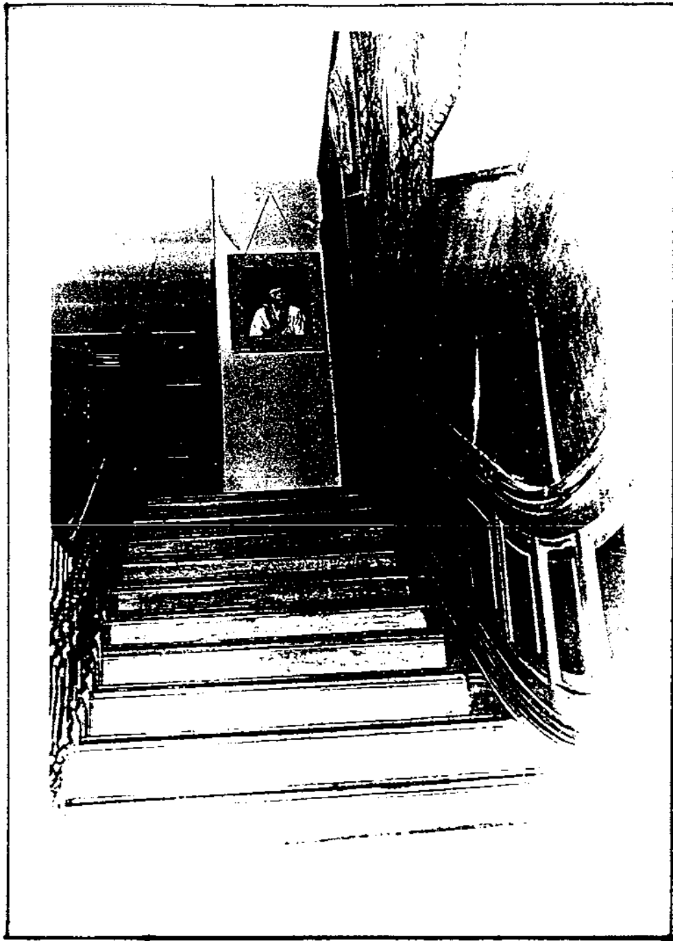
Fig. 1. Main staircase; Front Hall (Room 101) looking east, 1948. Photographic collection, SAHI NHS. After 1948, the rectangular wall at the top of the stairs was changed to an arch.
