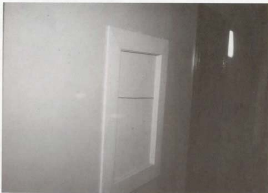
Typical Firebox Location in Hallway: Before Restoration
