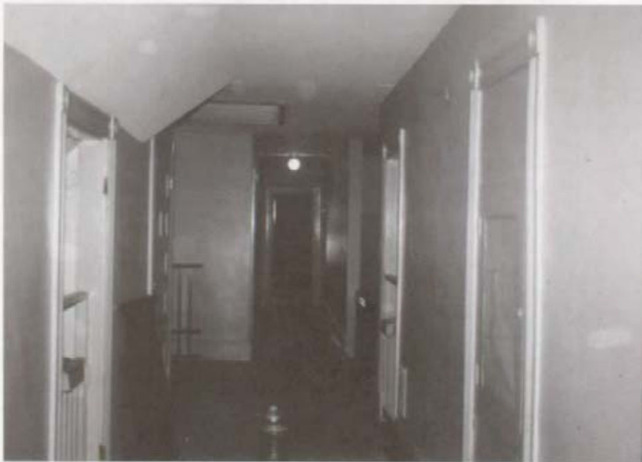
Third Floor Hall: Before Restoration
