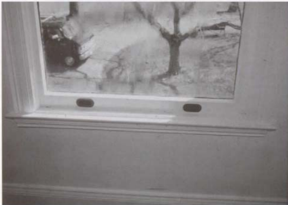
Typical Window Sash Condition After Restoration
