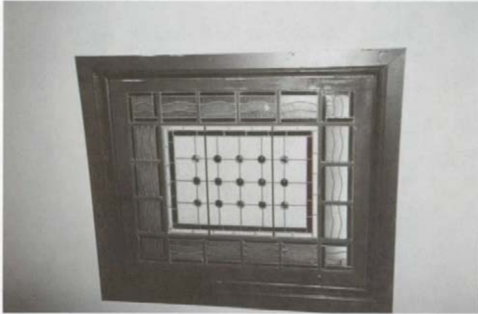
Figure 41. Stained-glass skylight over main stairway, second-story hall.
