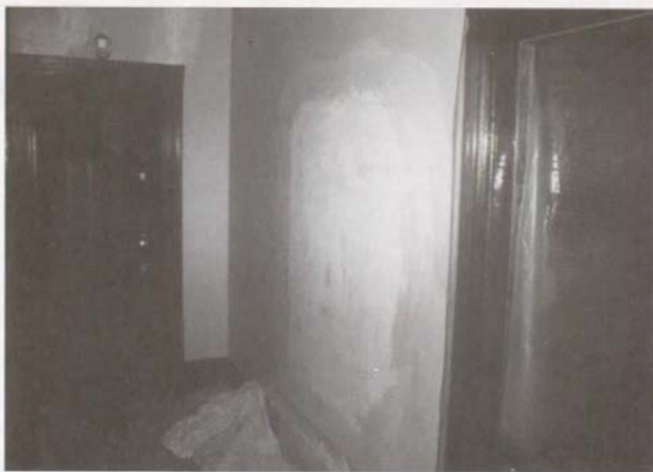
Typical Firebox Location After Removal and Replastering
