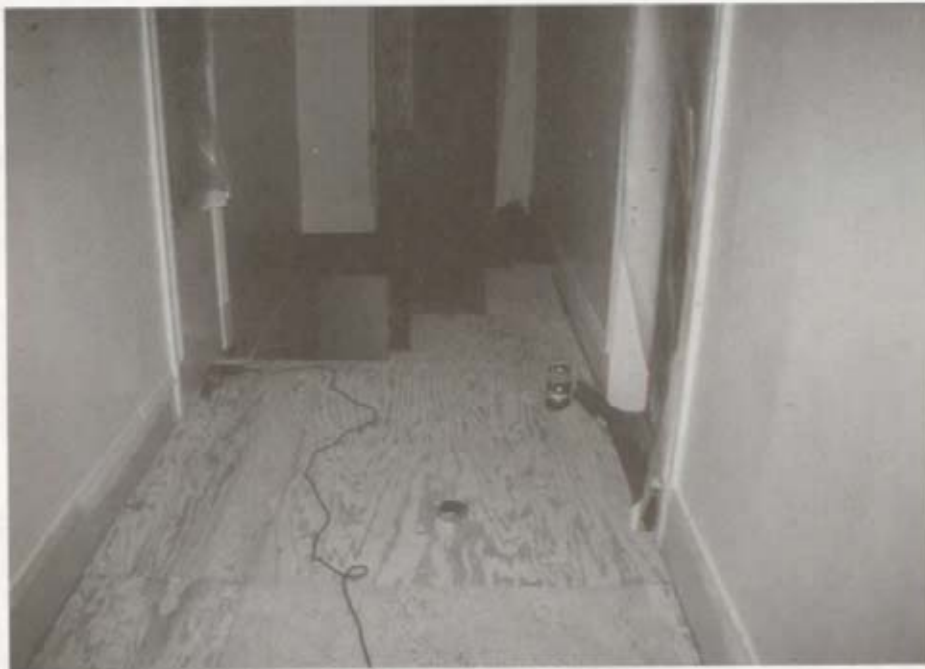
Third Floor Hall: Plywood Installed On Floor
