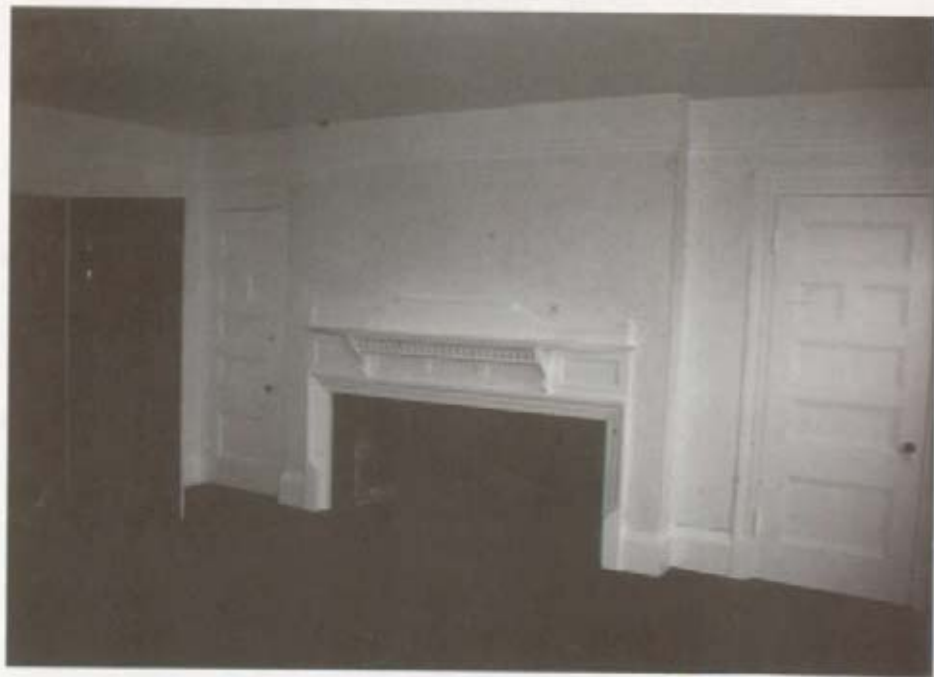
South Bedroom: After Restoration (ready for wallapering).
