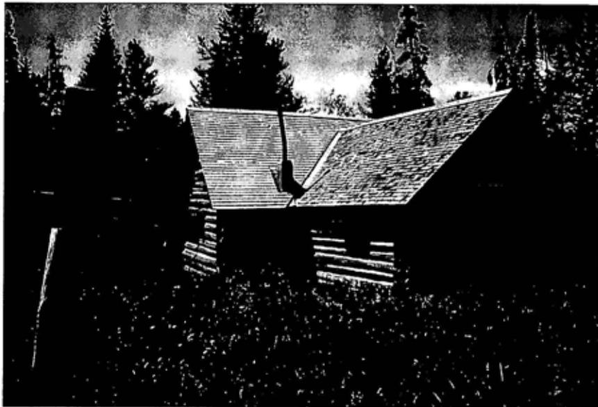
Figure 1. Crevice Mountain Cabin (Yellowstone National Park Slide File #15,021).
