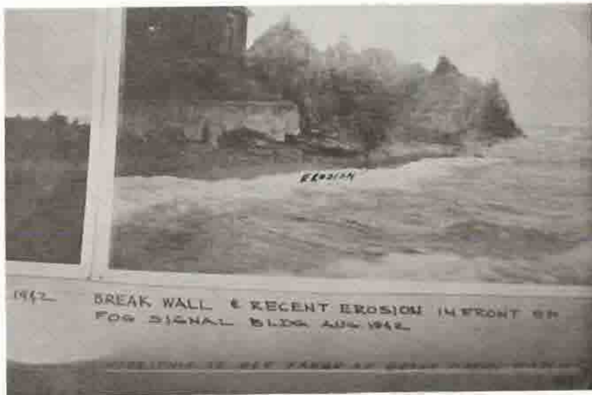
Illustration 26 Retaining Wall Photograph shows area of erosion. Park Files--August 1942
