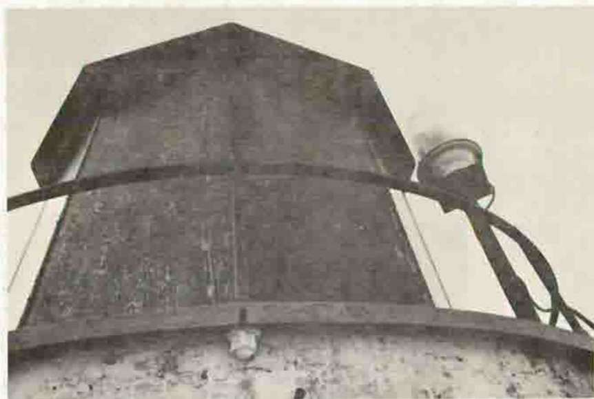
Illustration 8 Lantern Section and 1972 Automatic Light on Lighthouse Tower 1977
