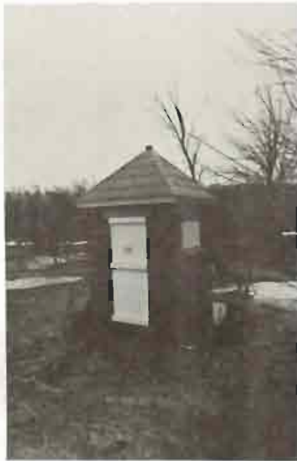
Illustration 54 1909 Privy Looking Southeast 1977
