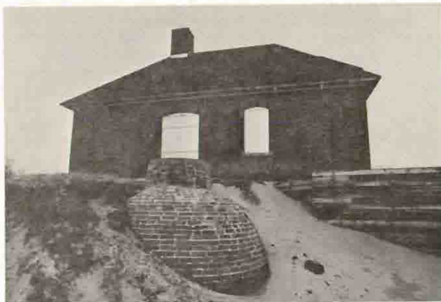
Illustration 25 Brick Cistern near Fog Signal House 1977
