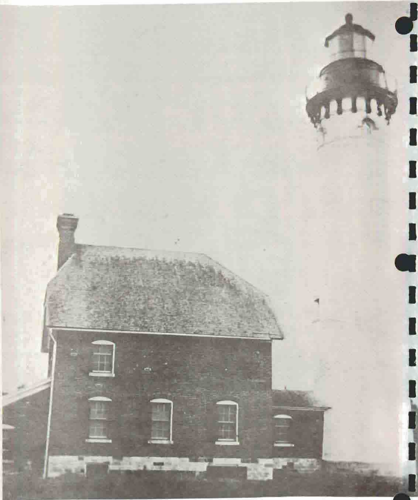
Illustration 35 Attached Dwelling Viewed from the North, 1904 (Photograph No. 26-LG-49-6B Record Group 26, National Archives)
