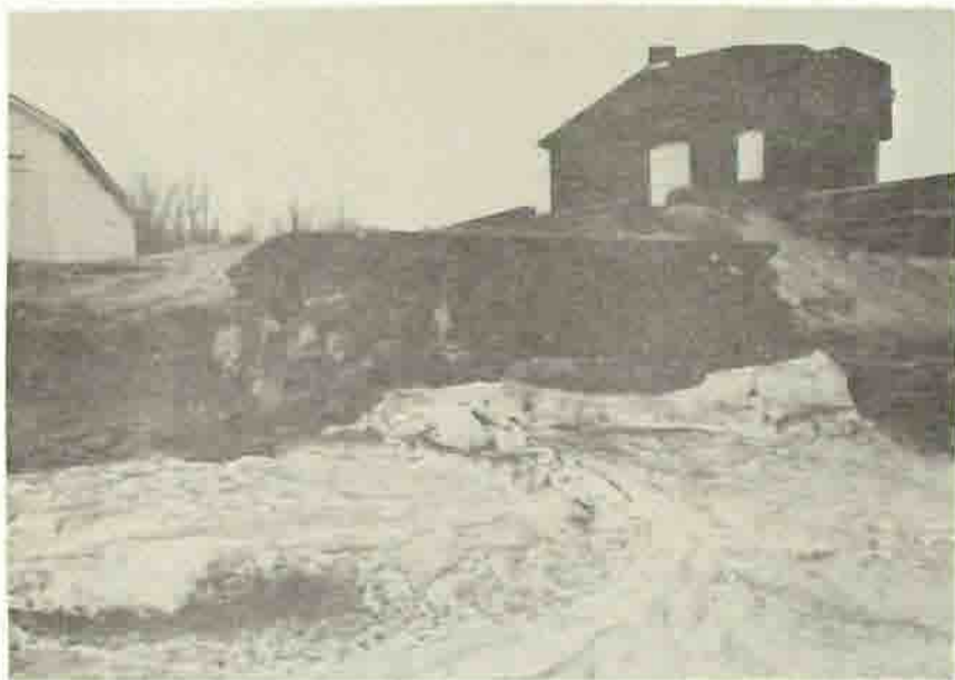
Illustration 29 Old Section of Retaining Wall on the East 1977
