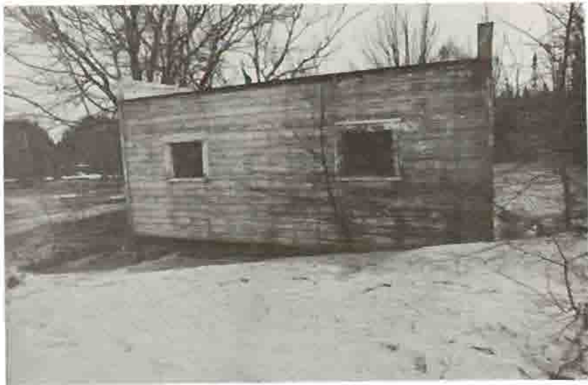
Illustration 56 Rear of Garage 1977
