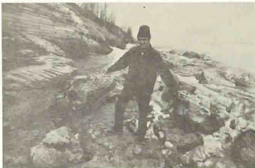
Illustration 33 Fallen Section of Retaining Wall 1977
