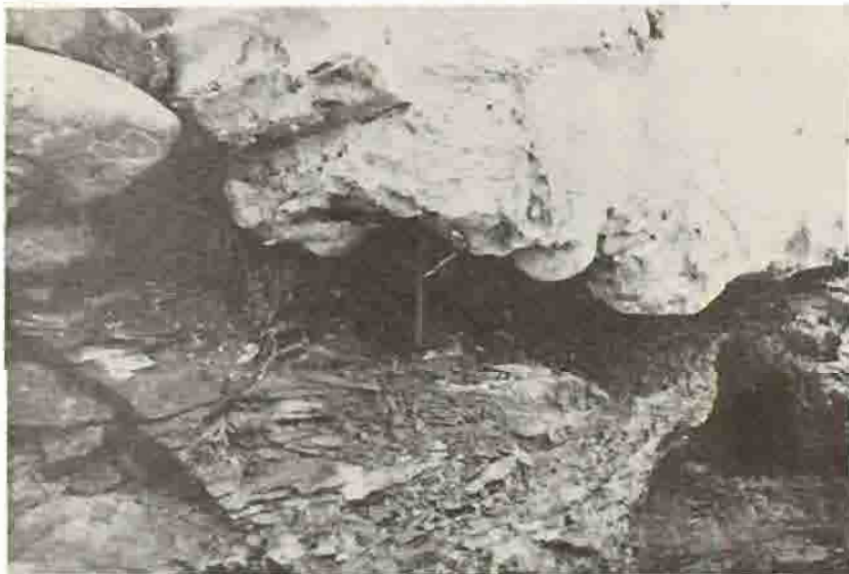
Illustration 32 Bottom of Retaining Wall, Anchored in Bedrock 1977
