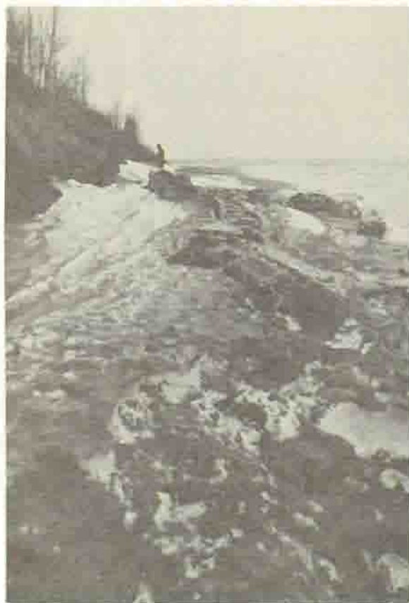
Illustration 30 Fallen Section of Retaining Wall 1977
