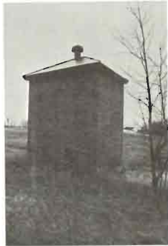
Illustration 21 Brick Oil House--Rear 1977
