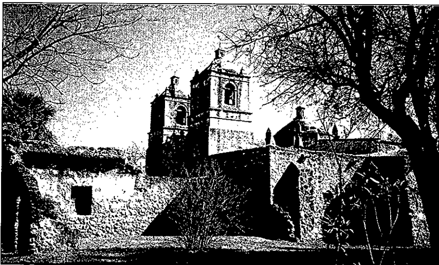
Figure 63. Mission Concepcion is one of five missions along the San Antonio River. The Mission is still actively used by the local community and is owned by the Catholic Archdiocese of San Antonio. Treatment and management decisions are made by the park in association with the Archdiocese based on a cooperative agreement. San Antonio Missions National Historical Park. (NPS, 1992)
