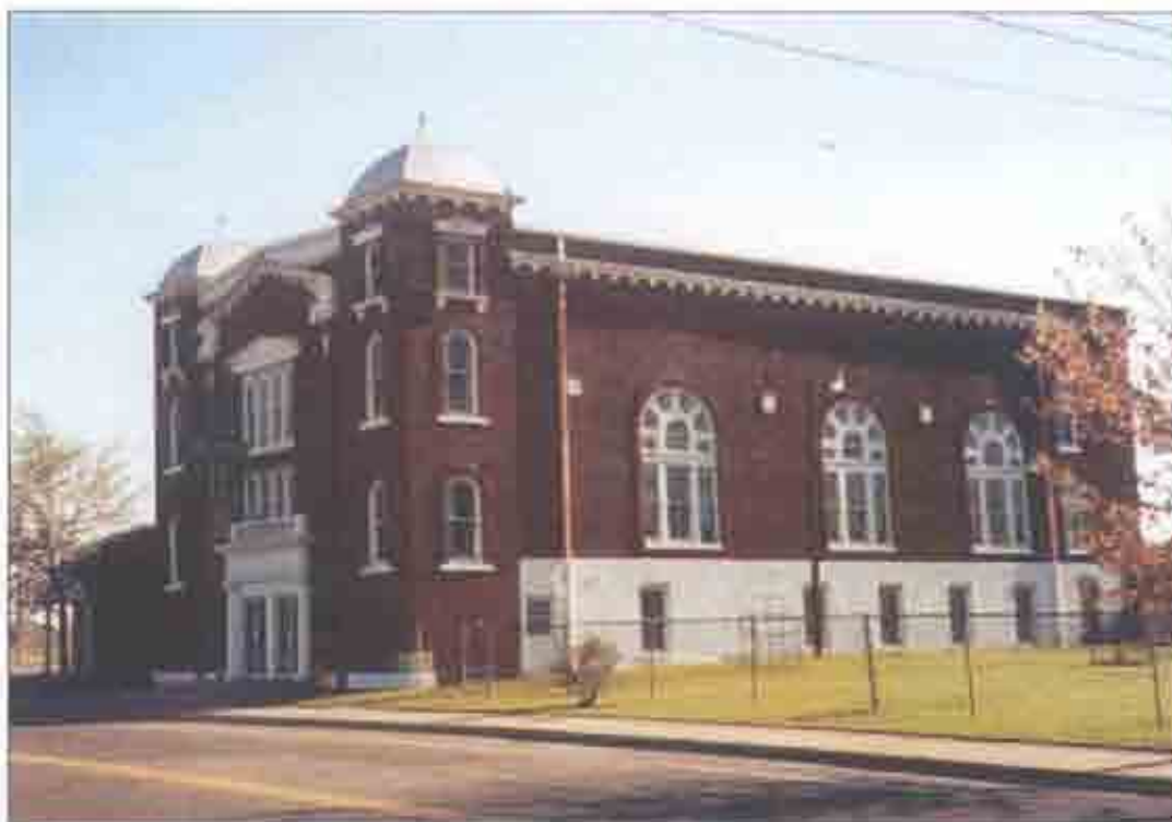
North and West (front) Facades.
