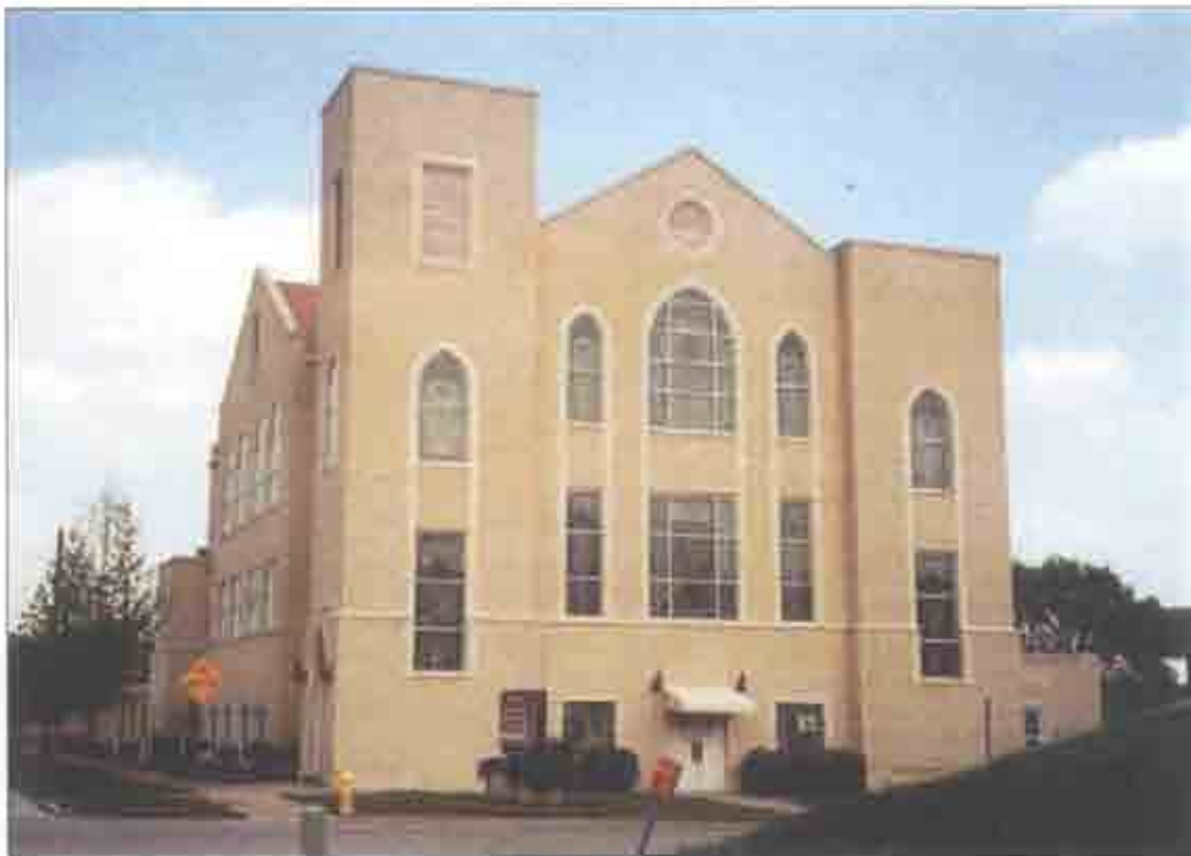
Southwest (Front) Façade.
