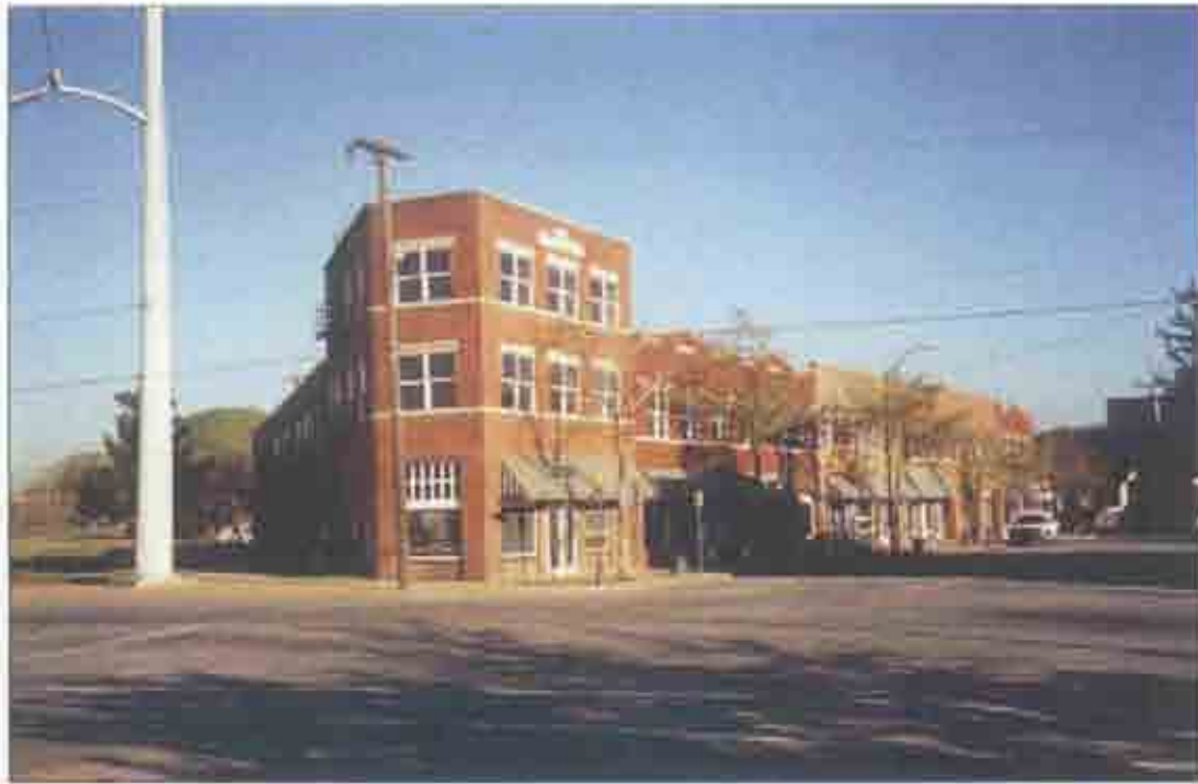
West Side of Greenwood Avenue looking north from Archer Street.
