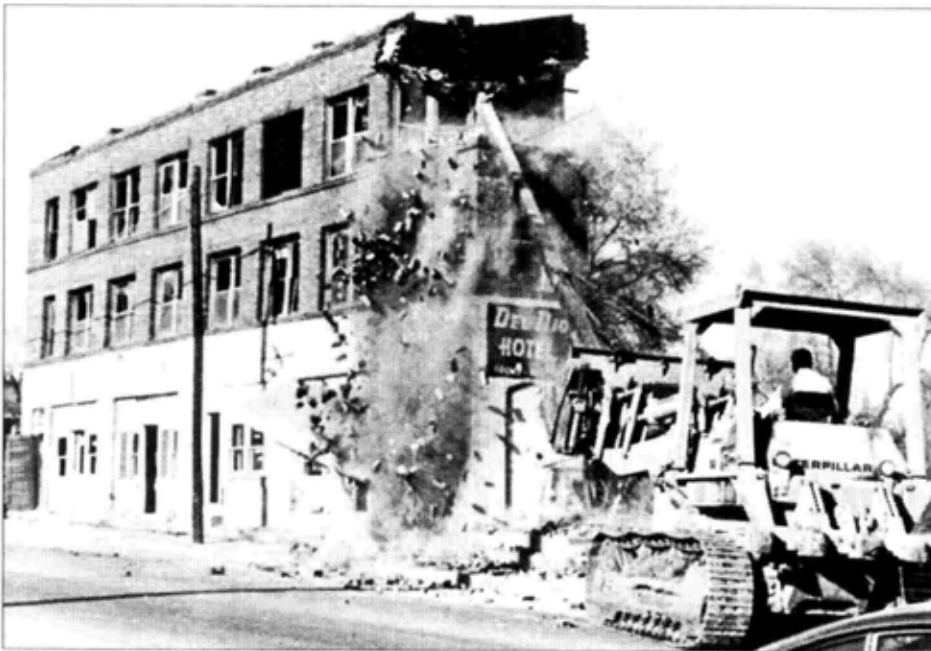
Urban renewal bulldozers demolishing Black Wall Street businesses during the 1960s - 1970s. Courtesy of the Greenwood Cultural Center.
