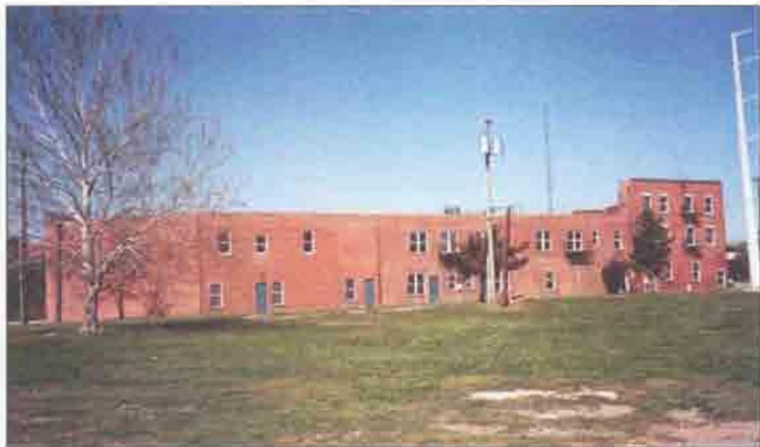
Rear of historic buildings on west side of Greenwood Avenue looking east from historic site of Royal Hotel on Archer Street.
