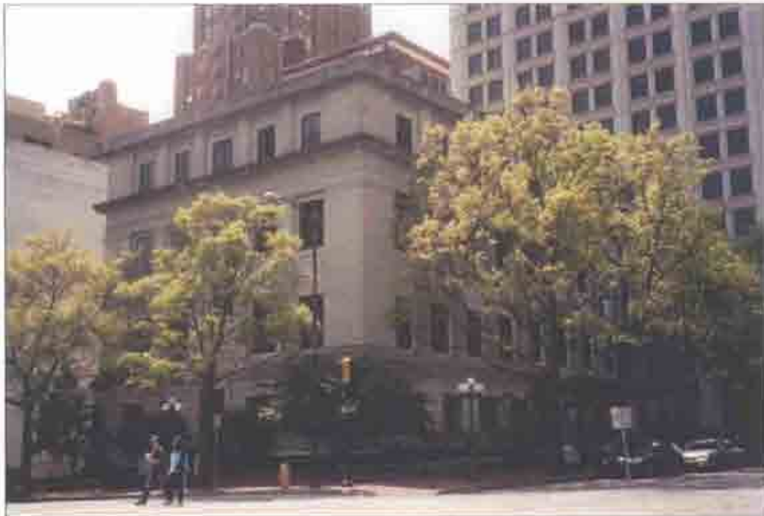
North and east facades of Tulsa Municipal Building.
