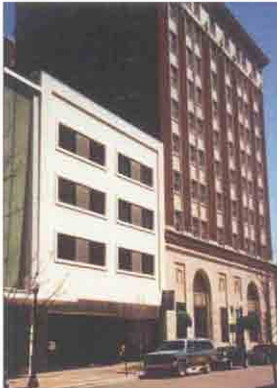
Front façade of Drexel Building.
