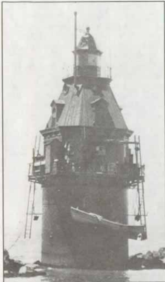
Figure 42. ShipJohn Light (pre-1876) is a Victorian caisson-type light in the Cohansey River. Undersail.
