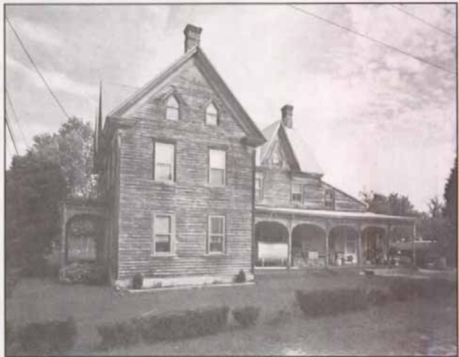
Figure 18. This Heislerville house (19th century) has fine Victorian elements in its pointed Gothic windows, gables, and spindlework trim; a store was in the rear.
