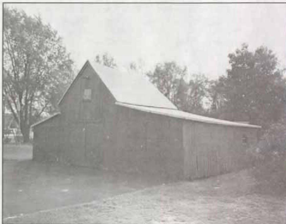
Figure 47. The drive-in corncrib form, here adapted for use as a garage, housed grain in the flanking compartments; the gable-end opening has been glazed.
