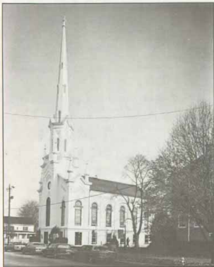
Figure 109. First Presbyterian Church (1856) facade has a projected entrance with a series of recessed facade and cornice lines, decorated steeple base and matching narthex-end walls.
