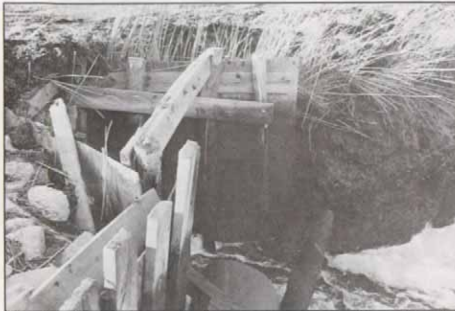
Figure 54. Sluice gates around a drain pipe let water escape from fields at low tide; as the tide rises, the gates press shut so as not to flood the fields. Sebold.
