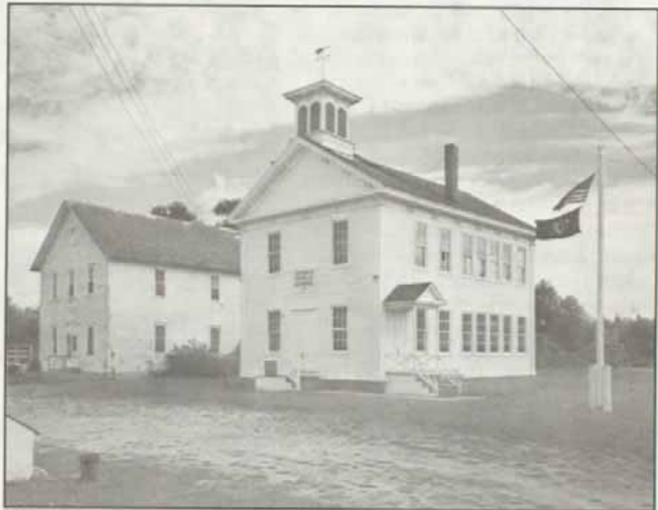
Figure 103. Goshen Public School (1872), with community building in background. Main gable-end entry and seven-bay side facades with banked windows offer improved light and ventilation.
