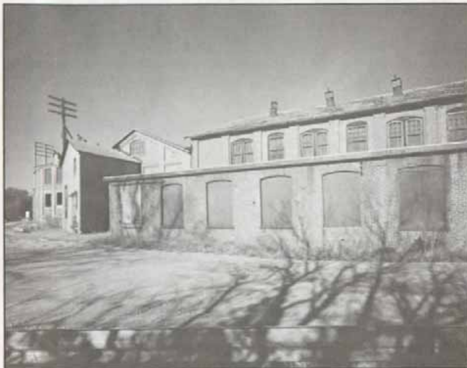
Figure 75. Now owned by Wheaton Industries, this complex of buildings includes the pump house once used by Millville Manufacturing Company.
