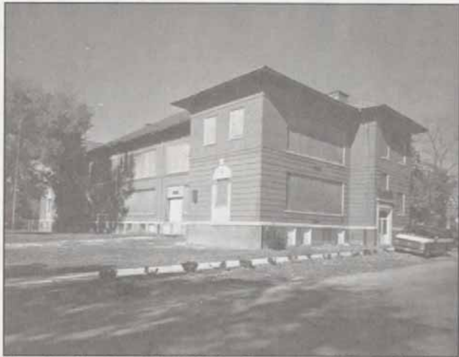
Figure 100. Vine Street School (1906). The two-story, H-plan building has a formal three-part brick facade with hipped roof and raised basement.
