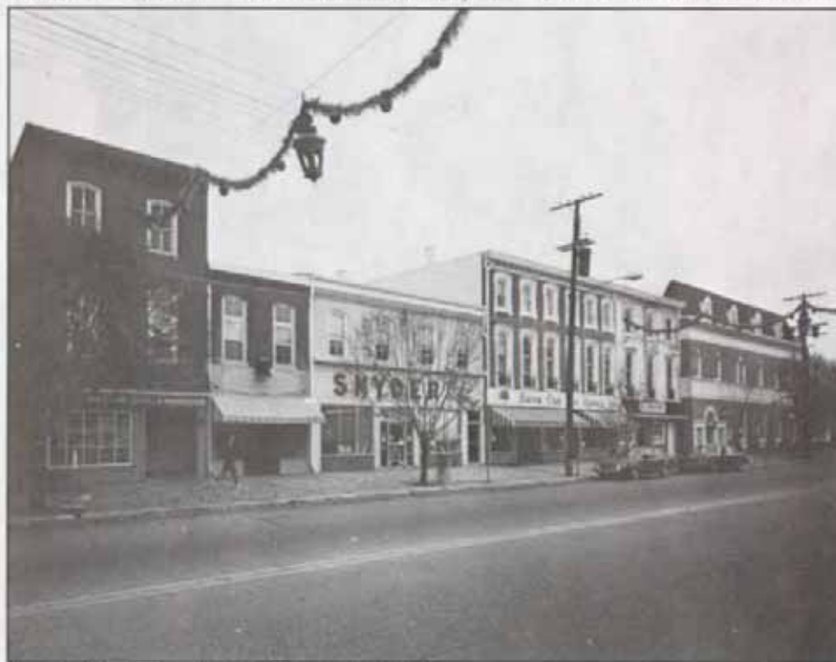
Figure 14. View of High Street, Millville.
