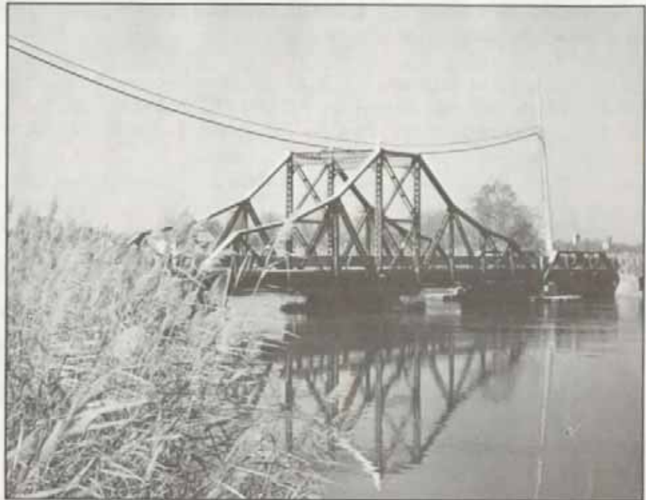
Figure 86. New Bridge Road Alloways Creek Bridge, built by the New Jersey Bridge Company of Manasquan (1905), is an unusual metal truss swing bridge with a Pratt pony-truss approach.
