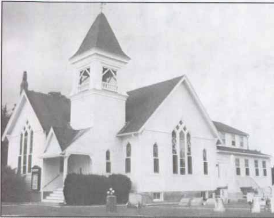
Figure 113. Goshen Methodist Church (ca. 1870). This church is an example of the irregular Victorian plan and abundant architectural texture. Leach.
