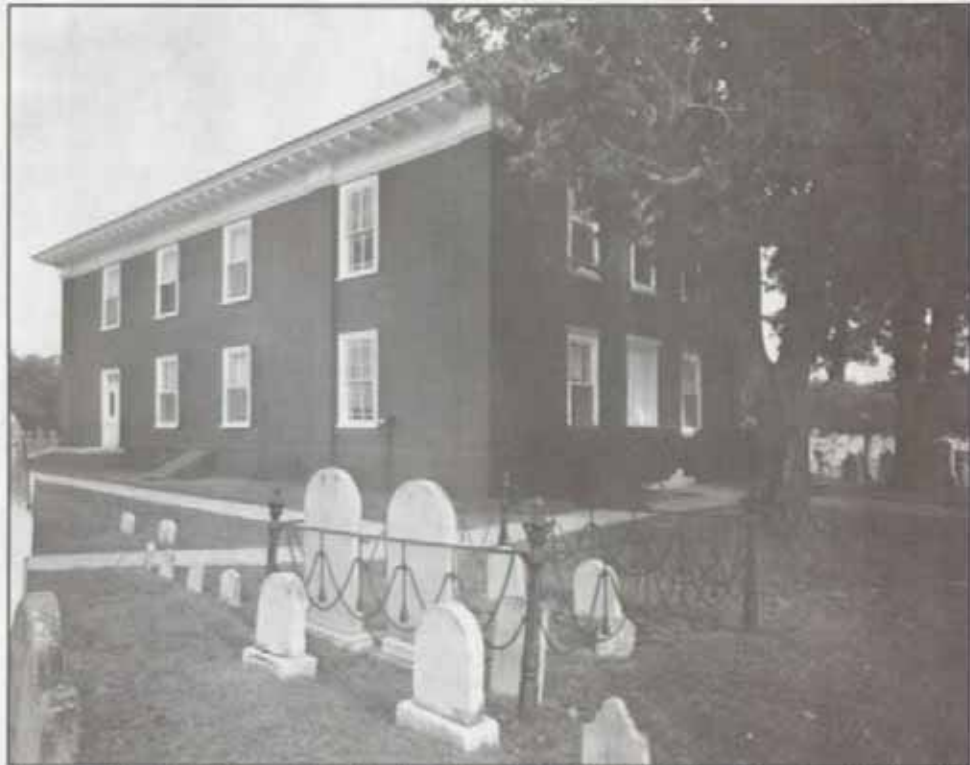
Figure 110. Cold Spring Presbyterian Church (1823, NJ-270). Two-story brick, with cornice and pediment with dentils. Three bays wide by four bays deep.
