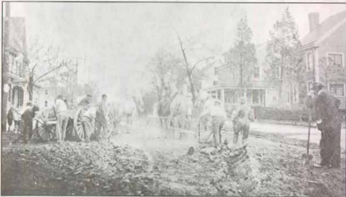
Figure 93. Working on the roadbed in Millville, Main Street/Route 49 at Fifth Street. Wettstein, 1915.
