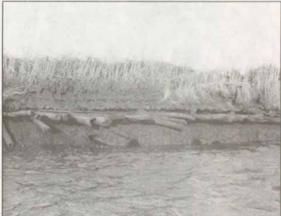
Figure 83. Corduroy road remains, such as these along Dennis Creek, are found preserved but buried in layers of mud throughout the tidal marshes. Sebold.
