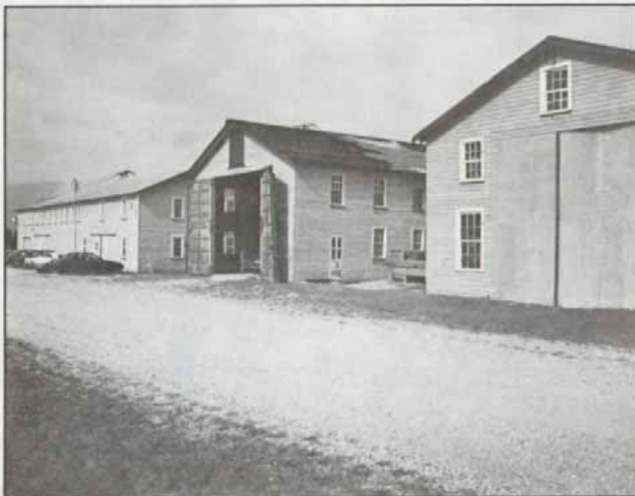
Figure 26. Del Bay Shipyard, located in Leesburg, repaired and built schooners as well as other vessels, including World War II mine sweepers.
