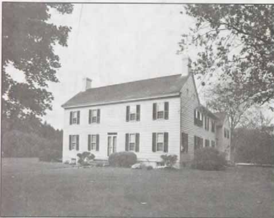
Figure 45. Christopher Ludlam House (1776), though plain, is an ordered, Georgian five-bay block with gable-end chimneys, center door, and rear additions.
