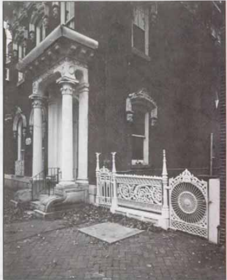
Figure 9. William Sharp House (1862), on Market Street, has 19th-century cast-iron fencing found throughout Salem.
