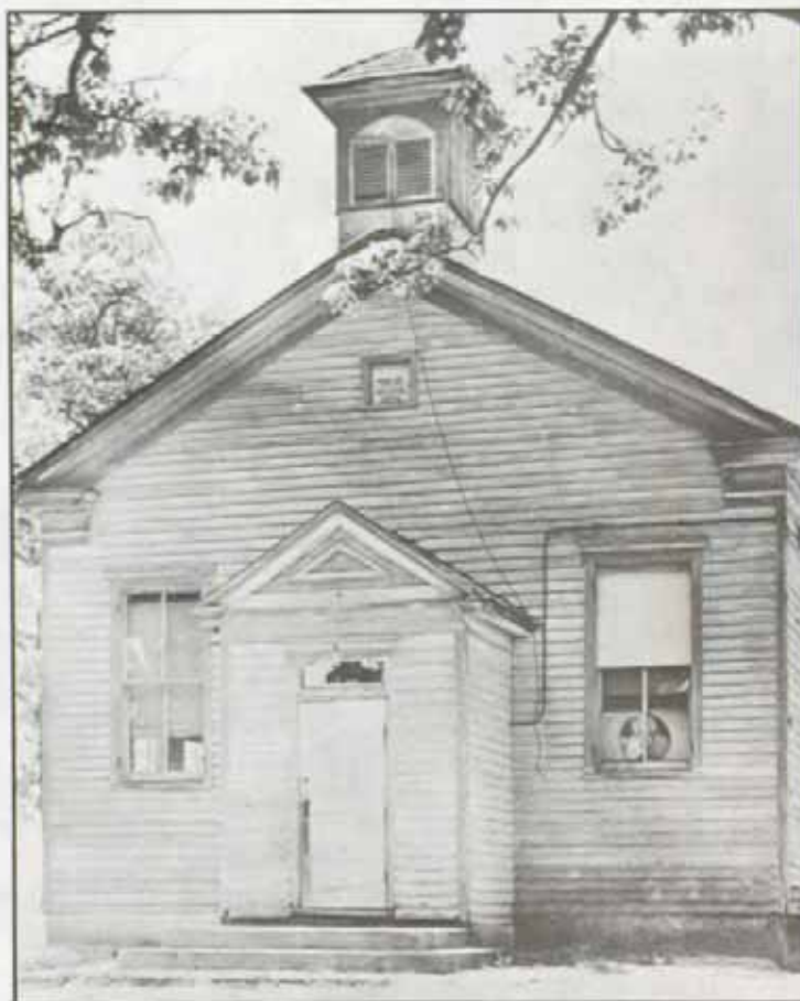
Figure 104. Buckshutem Public School (1875). The traditional gable front with returning cornice is topped by a cupola. Rutgers University, early 20th century.
