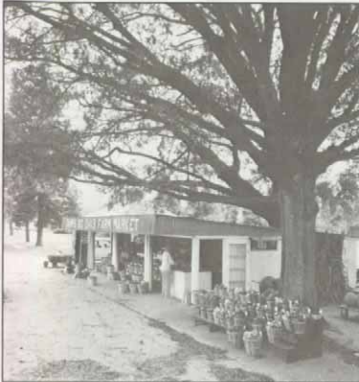
Figure 58. Camp's Big Oaks Market, near Port Elizabeth, is a partially enclosed utilitarian structure with a shed roof.
