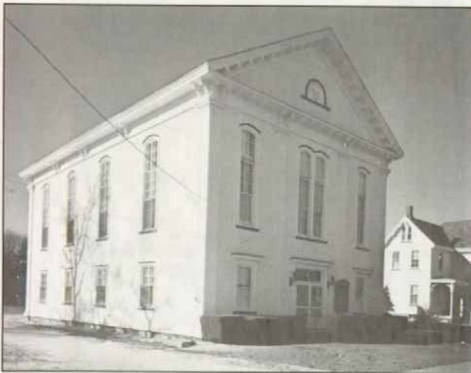
Figure 112 Cedarville Methodist Church. The two-story gable-front frame block is three bays by four bays, with a deep pediment and decorative cornerboard pilasters.
