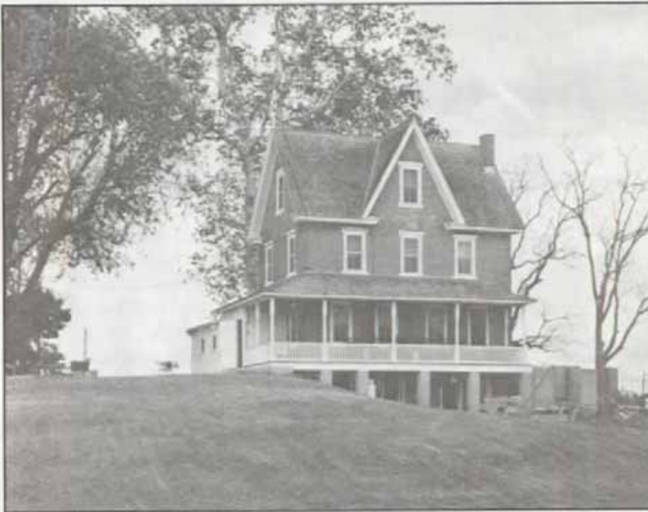
Figure 46. The Burcham Farm House (ca. 1870) is a vernacular Gothic Revival block, indicated by the center gable; the bricks were fired on the property.
