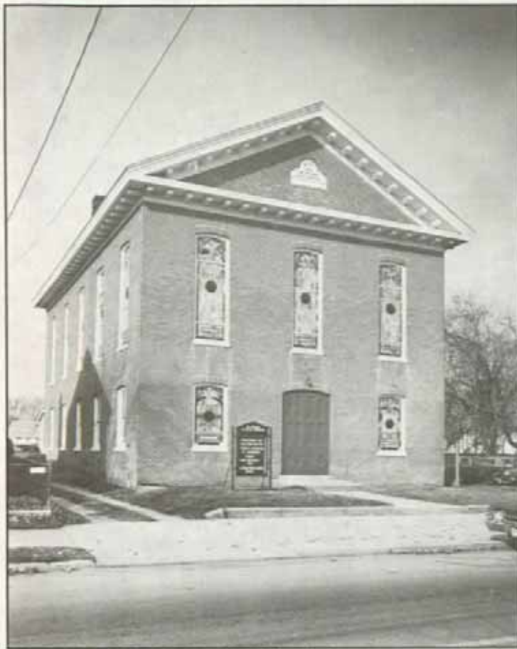
Figure 114. Mt. Pisgah AME Church is a two-story, three-bay brick block with a gable-front, deep pediment, and stained-glass windows.
