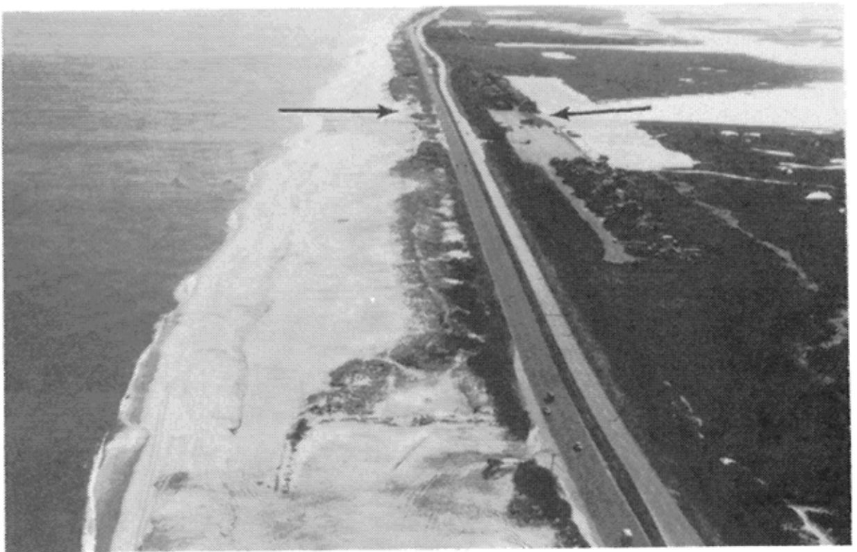
Figure 12. Gilgo State Park after removal of pavilion and riprap; remains of foundation visible in foreground. Note narrowing of barrier island at arrows due to oceanfront erosion and bayside boat channel dredged (in part) through salt marshes-likely site of a new inlet. Photo taken June 1978.
