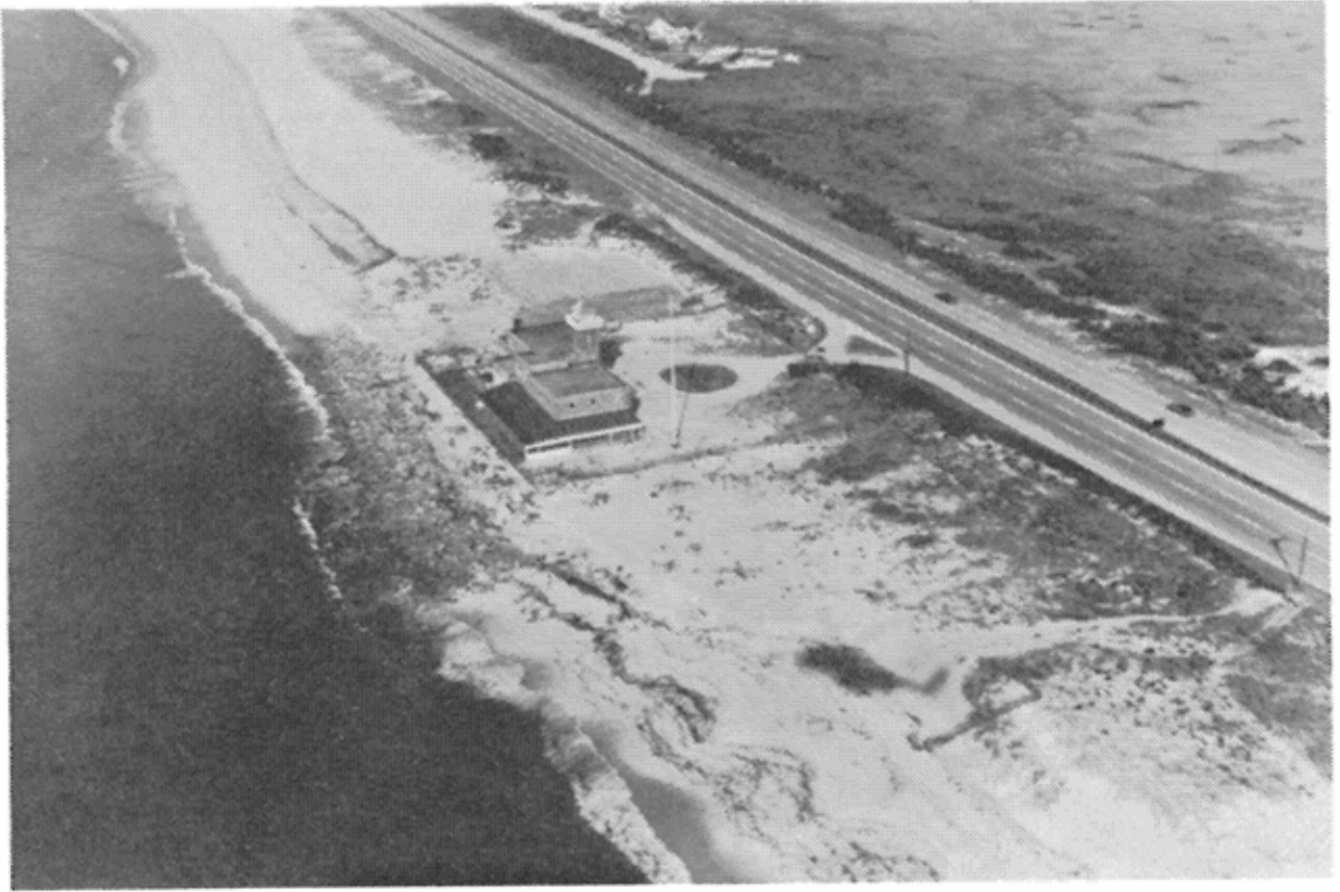
Figure 11. Gilgo Pavilion looking west August 1971. This photo taken when sediment loss had reached its maximum, only 17 months after emplacement (cf. Figures 10, 12). Note rubble riprap immediately in front of structure. Photo courtesy New York District, U.S. Army Corps of Engineers.
