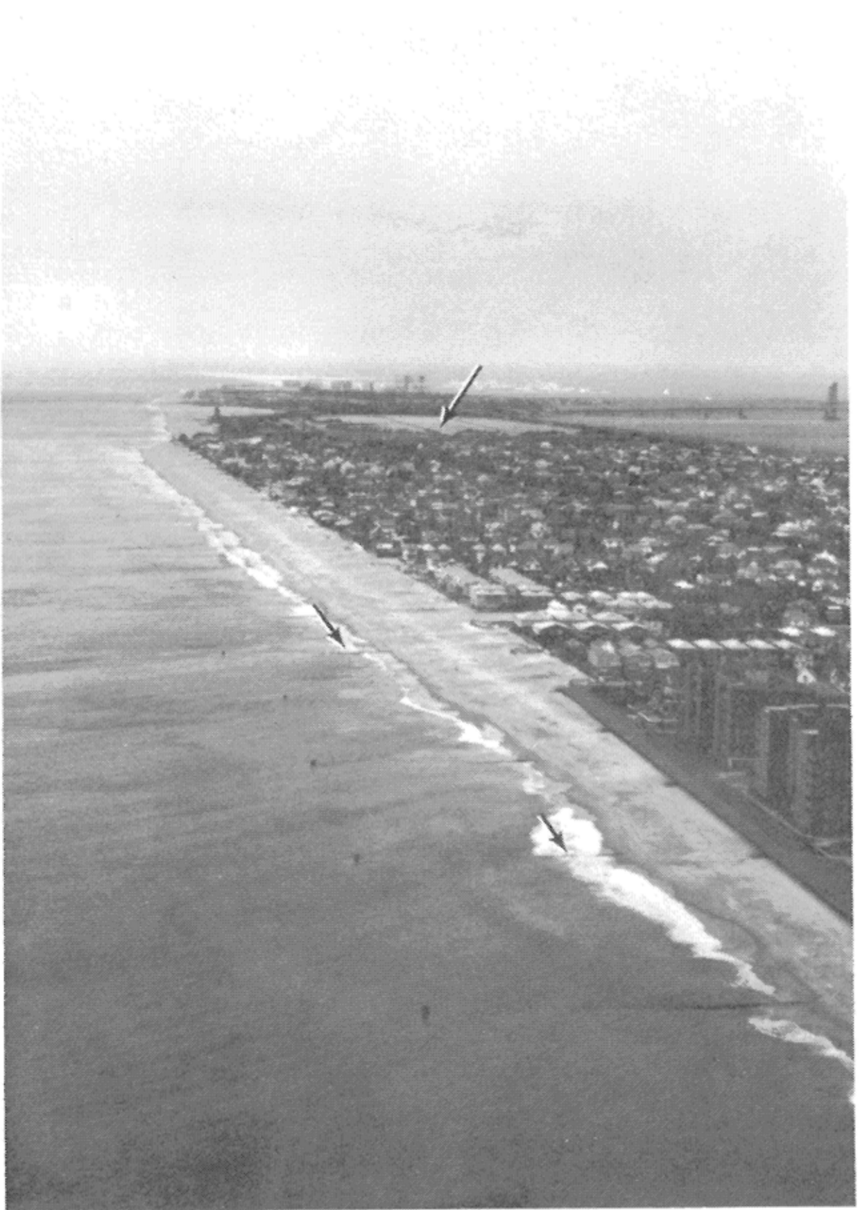
Figure 4. Rockaway Beach, Queens County, New York City, looking westwards towards Jacob Riis Park (far arrow). Photo taken February 1975, not long after beach nourishment covered most groins (near arrows).
