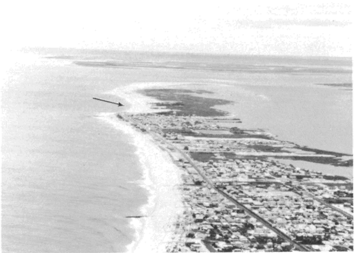
Figure 1. Long Beach Island, New Jersey, looking south towards Holgate Wilderness portion of Brigantine National Wildlife Refuge. Note westerly offset to barrier beach past groin field (arrow). Photo taken May 1977.
