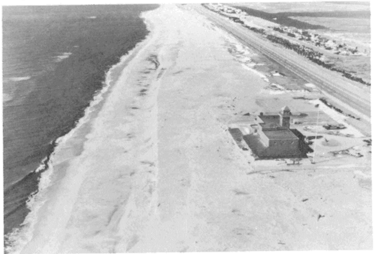
Figure 10. Gilgo State Park Pavilion, Jones Beach, Long Island, New York, looking west March 1969, after extensive beach replenishment with sand bypassed from Democrat Point, Fire Island, across Fire Island Inlet. Photo courtesy New York District, U.S. Army Corps of Engineers.
