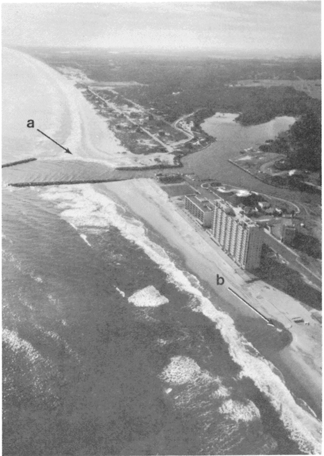
Figure 5. Rudee Inlet jetties, Virginia Beach, Virginia, looking south December 1979. Longshore transport is south to north, sediment dropping into the weir-jetty basin (arrow at "a") is then transported across the inlet by pipe and released downdrift (arrow at "b").
