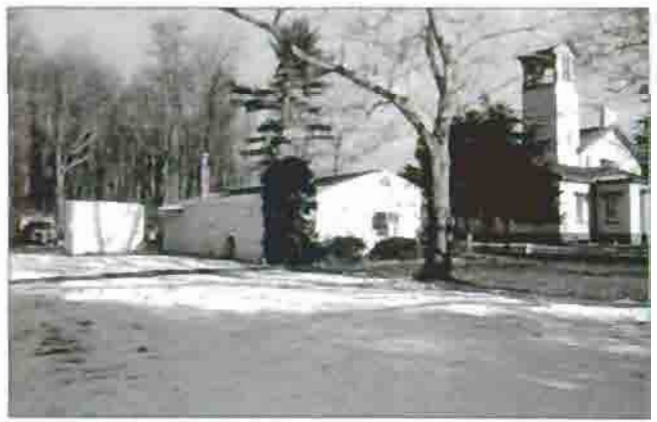
Figure 86: Maintenance building and chemical storage shed behind mansion.
