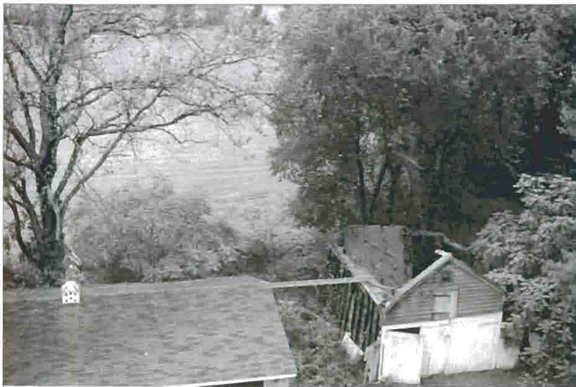
Figure 64: Garage on right built by Dr. Birney, partially collapsed, circa 1969. Campbells garage on left later used as NPS maintenance building. A portion of the upper terrace agricultural field under cultivation by Meyer is visible behind the two buildings. (Photo CLR - 429, MVB NHS).
