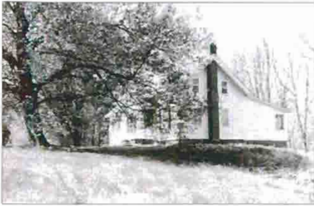
Figure 81: View south of the farm cottage.
