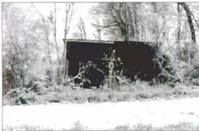
Figure 83: Open-fronted storage shed on the north side of the road between the upper and lower terrace.
