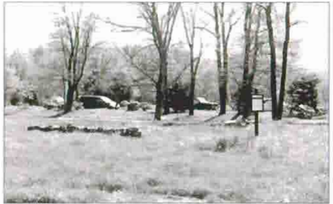
Figure 85: View east of the north gatehouse site, Old Post Road section and NPS parking lot.
