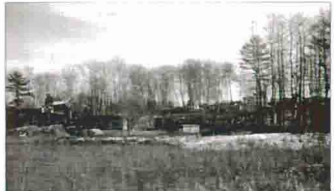
Figure 97: View southeast of eroding slope on property adjacent to site.
