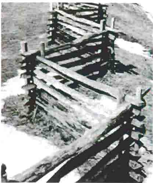
Fig. 7-6 Rail fence, with upright supports providing additional stability (Near Sharpsburg, Maryland, 1979)
