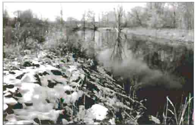
Figure 73: View west of Kinderhook Creek with shale and concrete slabs lining the southern bank.
