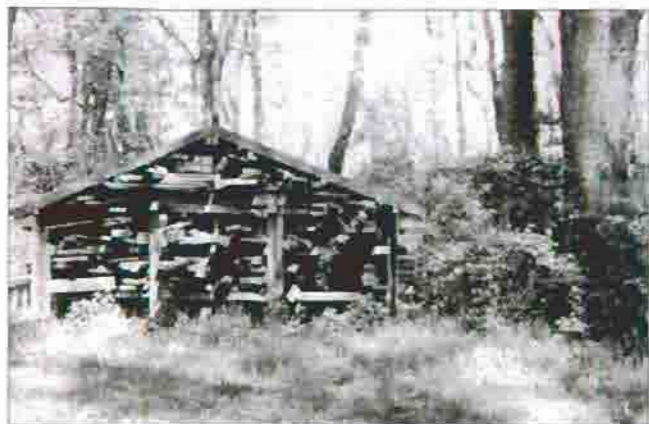
Figure 87: Lumber storage building in the north woods.
