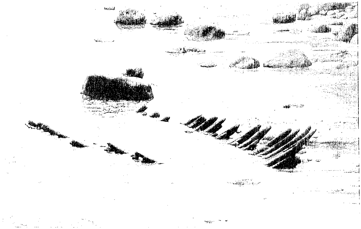
Figure 6.1. A hull section partially exposed near the pier, Becher's Bay, Santa Rosa Island, in the general area where the Ella G wrecked. NPS photo by Don Morris.
