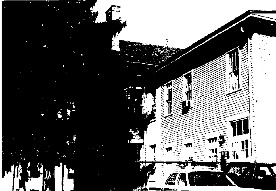
Figure 81. Ell: South Elevation, Looking Southeast.
