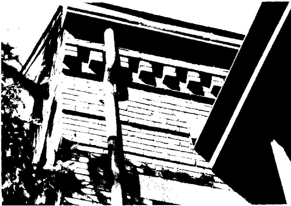
Figure 83. Main Block, East Elevation: South End, Cornice and Eaves at Junction of South-Unit Stair Tower.
