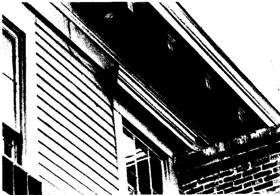
Figure 82. Ell, North (Rear-Yard) Elevation: Window W224 with Cornice Hood (circa 1859-1878).
