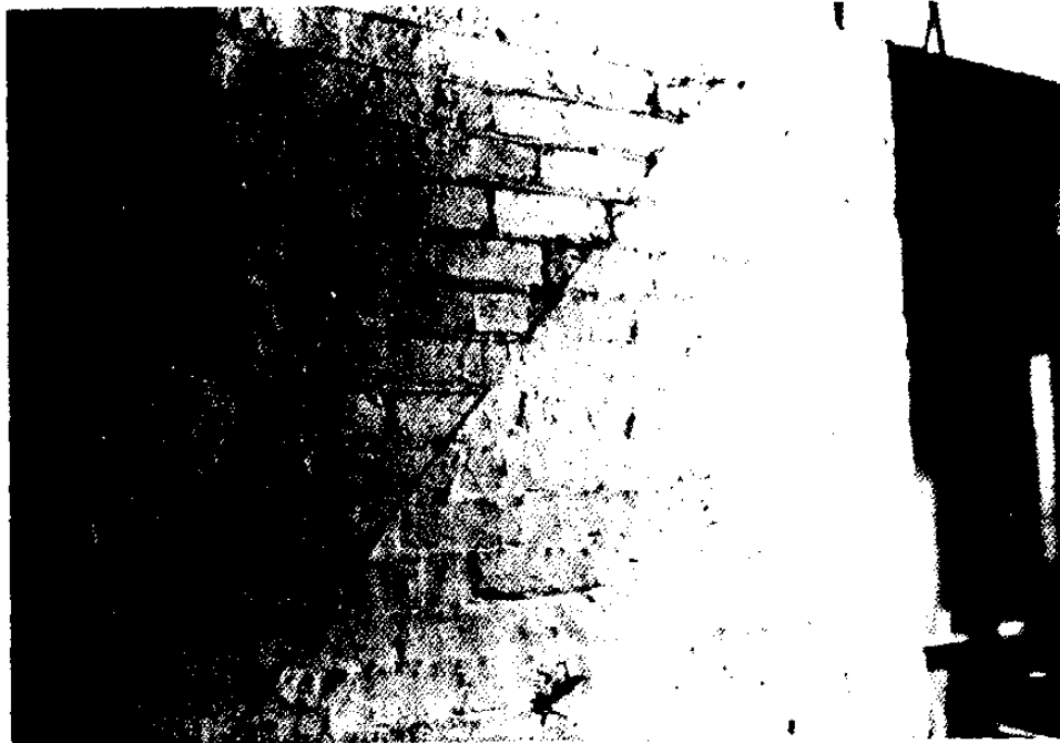
Figure 32. Room N002 (Cellar of North-Unit Stair Tower), West Wall: Paint Evidence of Former Staircase.
