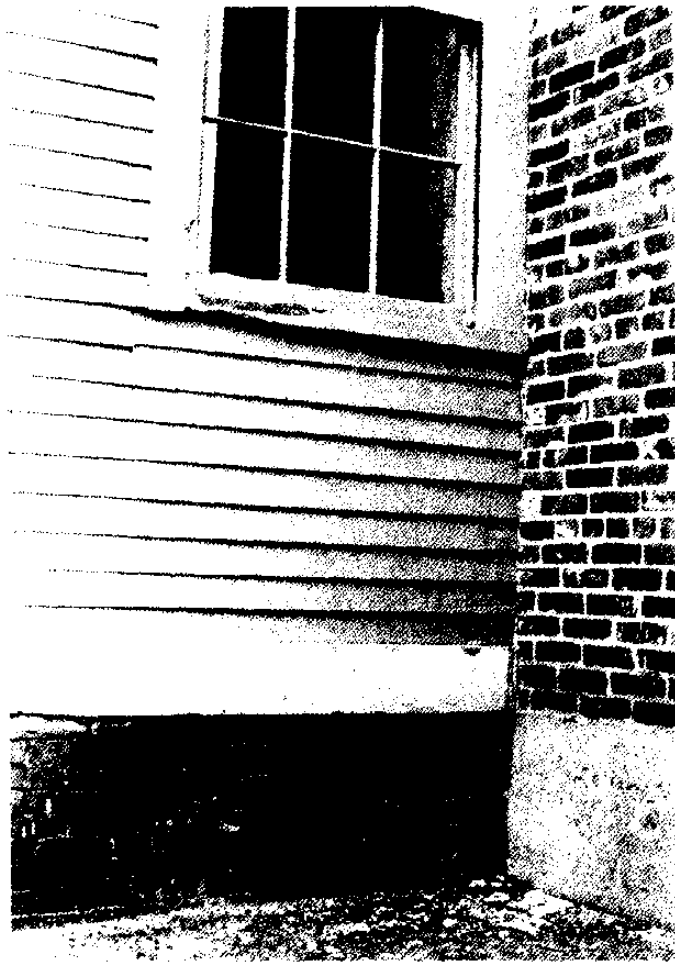
Figure 75. Ell, North (Rear-Yard Elevation): Foundation and Water Table.
