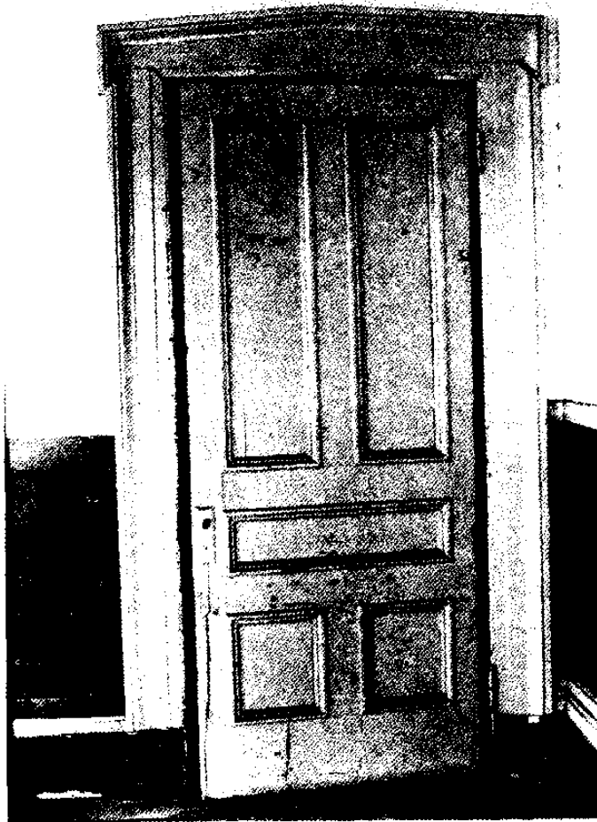
Figure 54. Room N101, East (Dining Room) Portion: 1890's Five-Panel Door.
