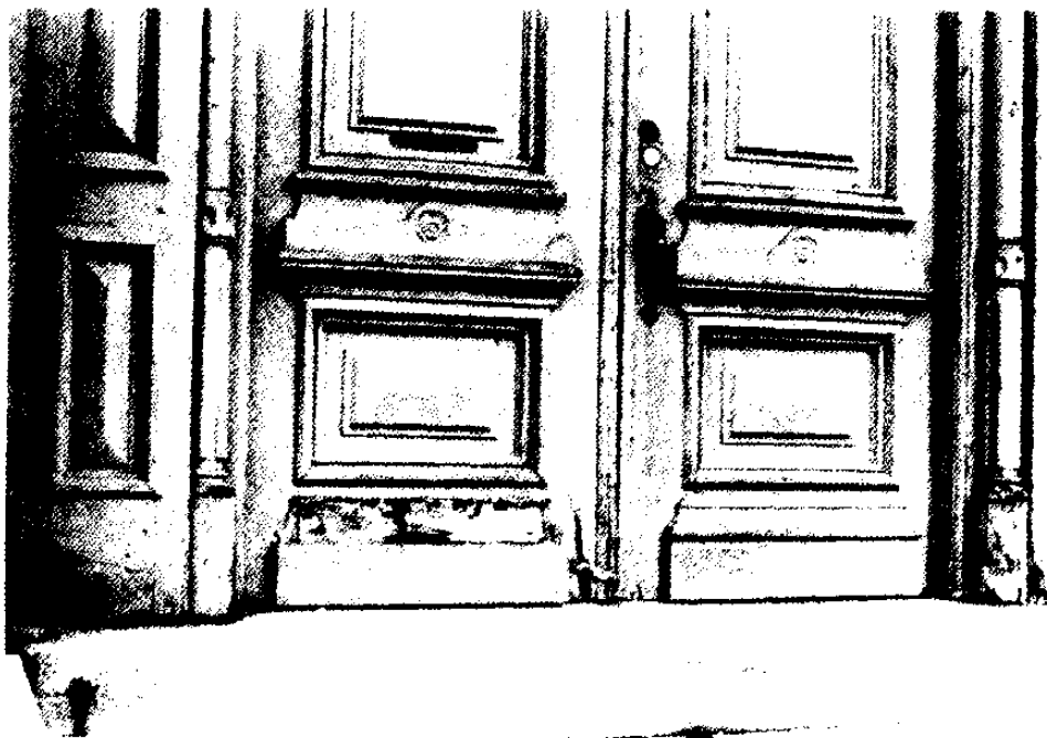
Figure 78. Main Block, West Elevation: Detail of Deteriorated South-Unit Entrance Door.
