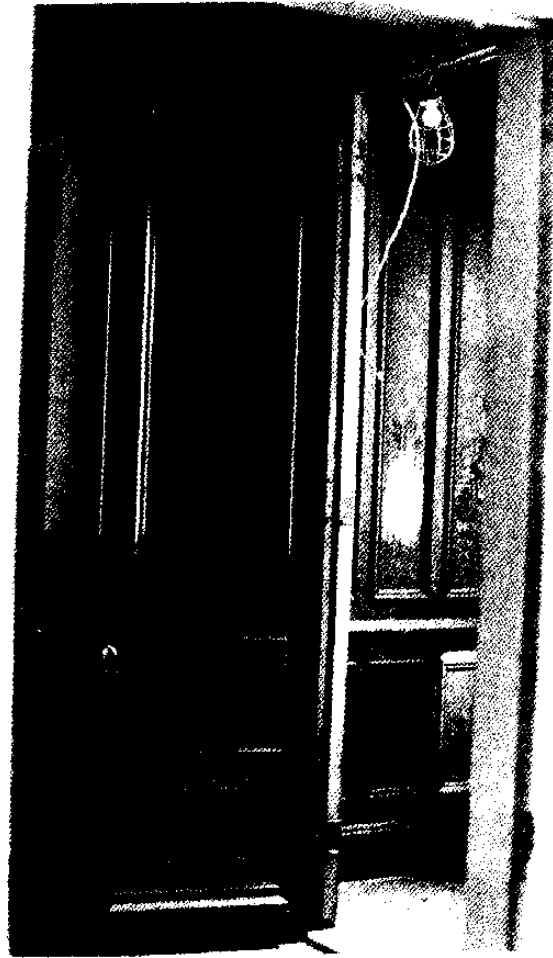
Figure 53. Room N106: Vestibule Door and Paneling.
