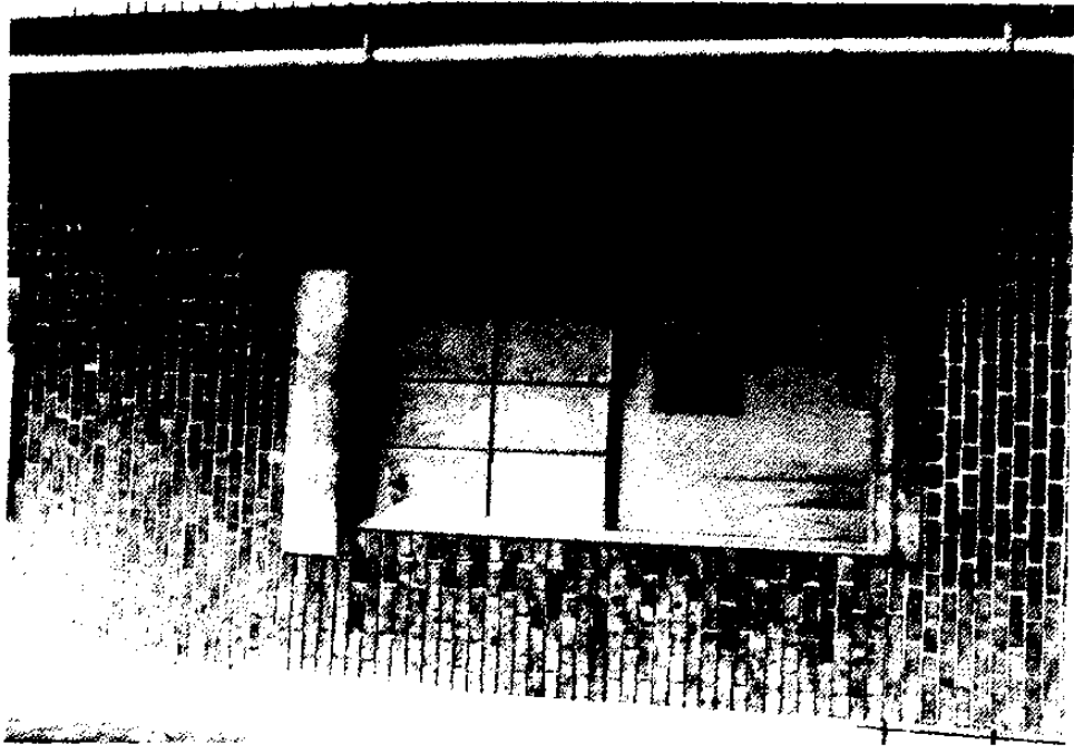
Figure 74. North-Unit Stair Tower, North Elevation: Window W124.
