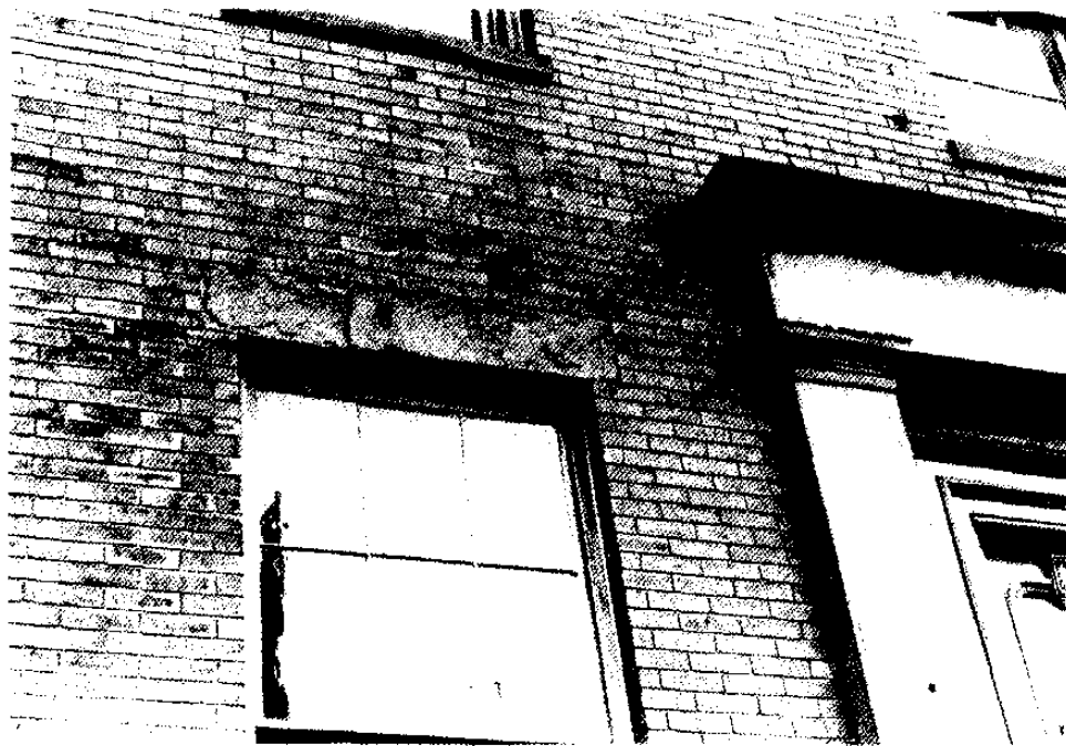
Figure 80. Main Block, West Elevation: Deteriorated Lintel over Window W106.
