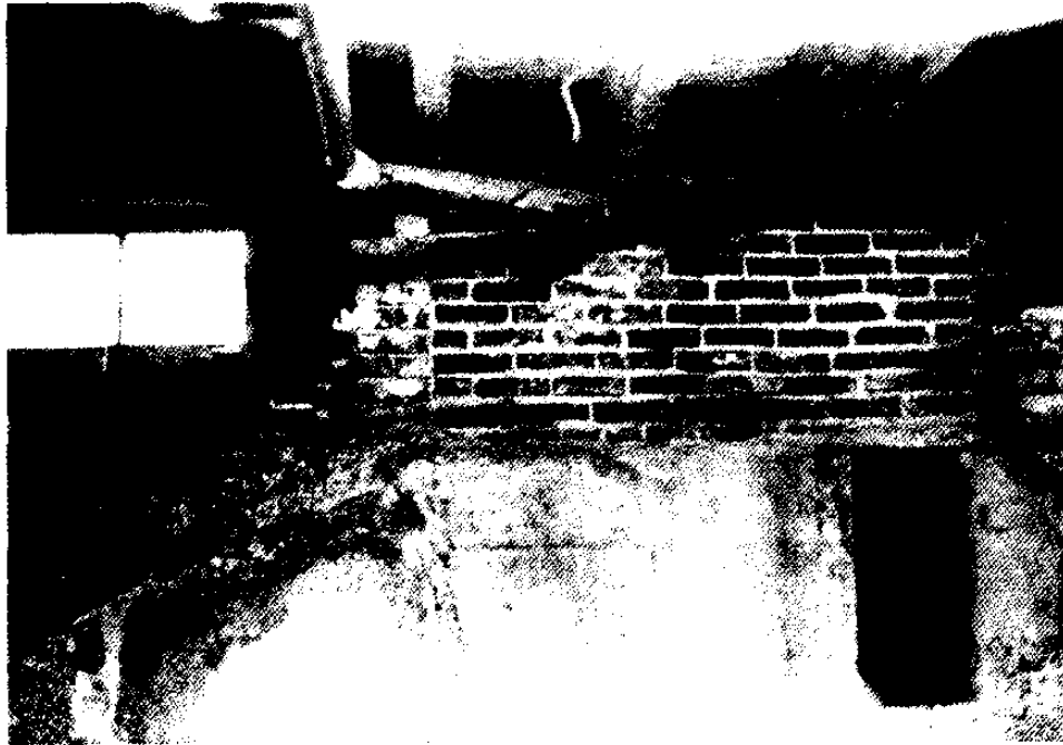
Figure 88. Room E001 (Ell Cellar), East Wall: Blocked 1847 Bulkhead Opening.
