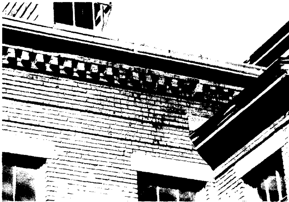
Figure 76. Main Block, East Elevation: Cornice and Eaves at Stair Tower.
