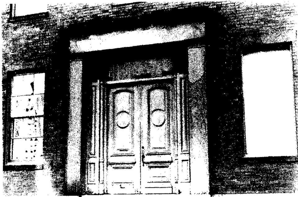
Figure 47. Main Block, West Elevation: South-Unit Entrance.
