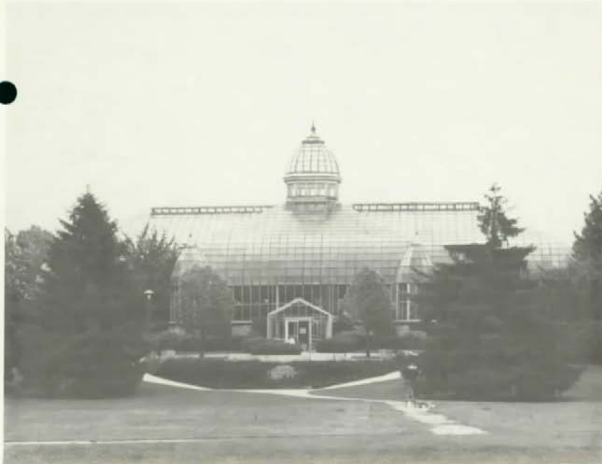
Franklin Park Conservatory, Columbus, Ohio Photo, NPS files
