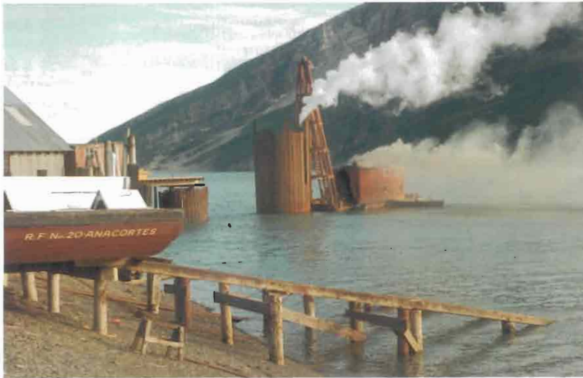
"Building the permanent dock," courtesy of Dorothy Fribrock, private collection.
