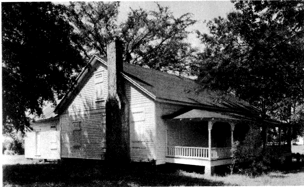
Photograph 9. Kolb house in 1961 prior to rehabilitation
