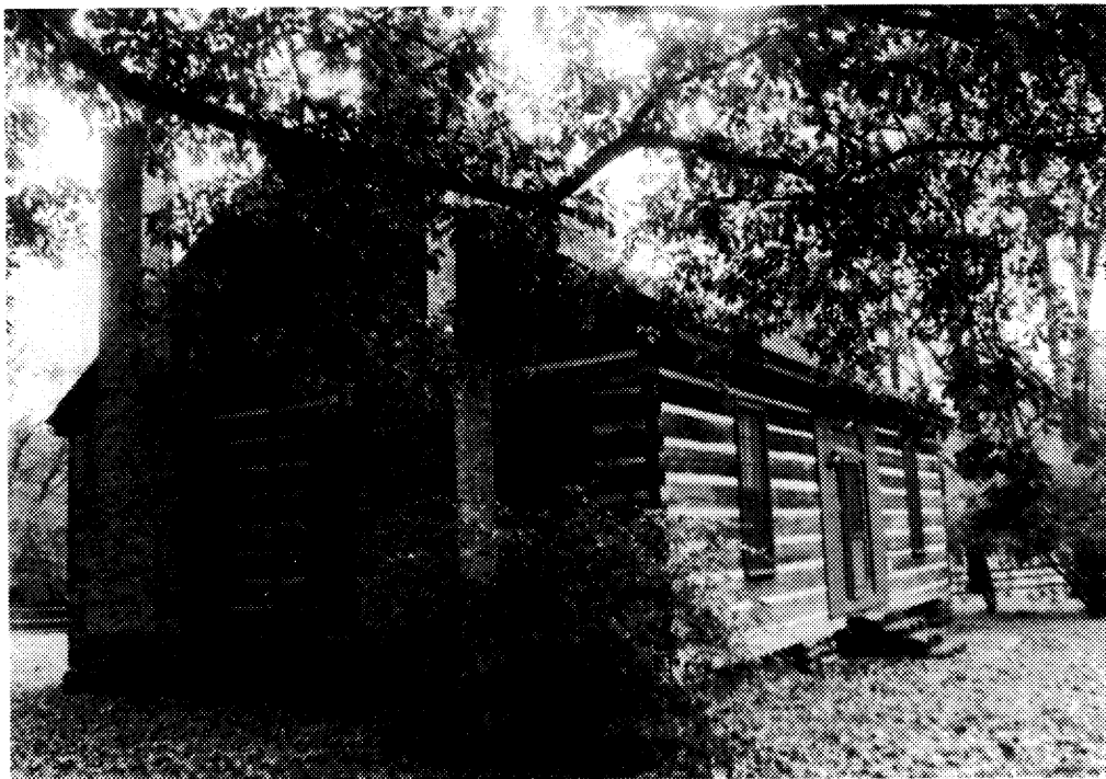
Photograph 10. Kolb house in 1992
