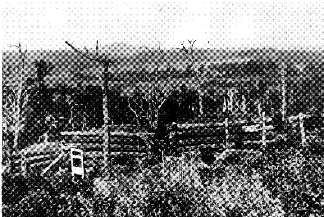
Photograph 4. View from behind Confederate earthworks on Pigeon Hill, showing log revetments (U.S. Signal Corps photograph, National Archives)
