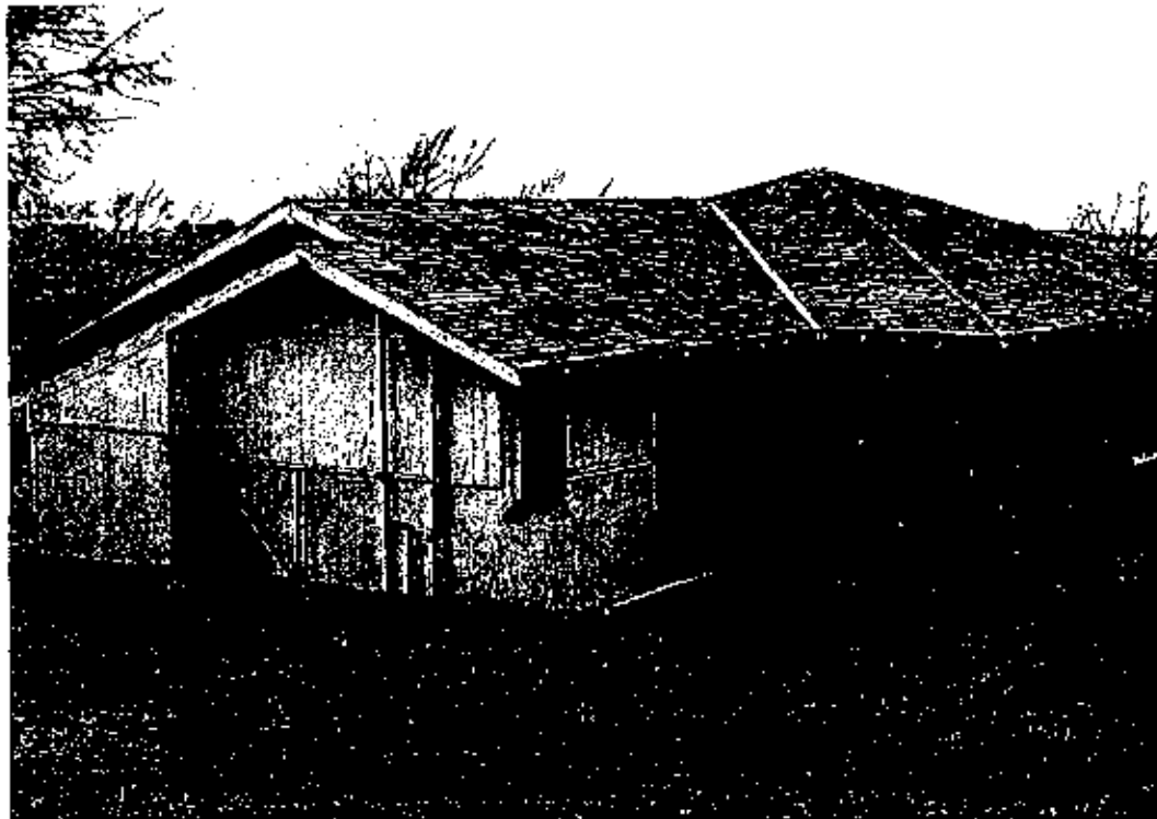
Figure 40. Stone, Principal Keeper's Residence (Feature 7), from east/northeast, September, 1999. Photograph: William Chapman.
