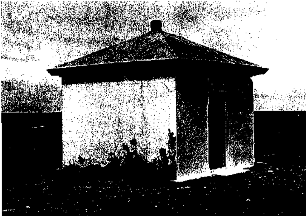
Figure 48. Oil-storage building (Feature 11), view from south, September, 1999. Photograph: William Chapman.
