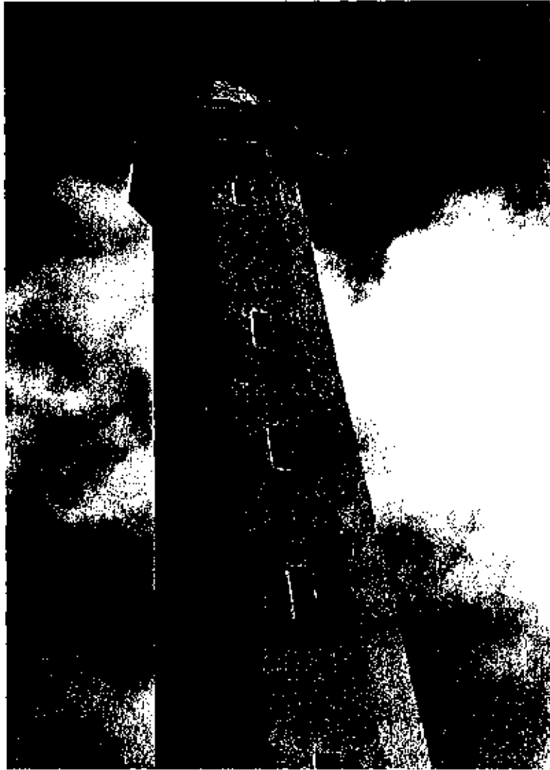
Figure 27. Lighthouse tower (Feature 1), view from west, September, 1999. Photograph: William Chapman.
