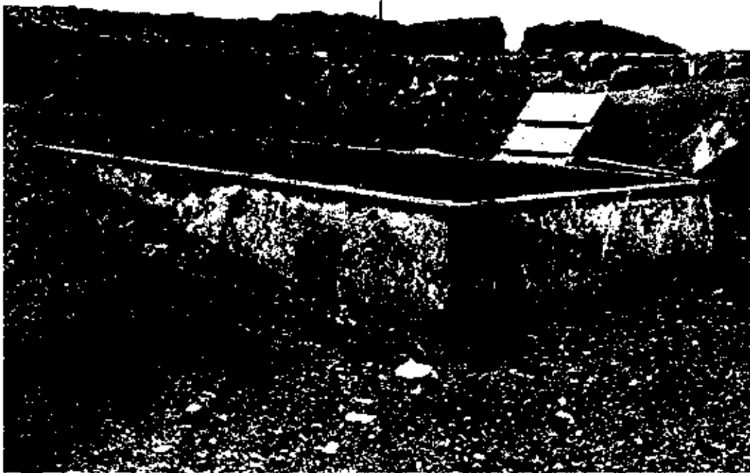
Figure 29. Reinforced-concrete base of former oil-storage tank (Feature 2), from east, September, 1999. Photograph: William Chapman.
