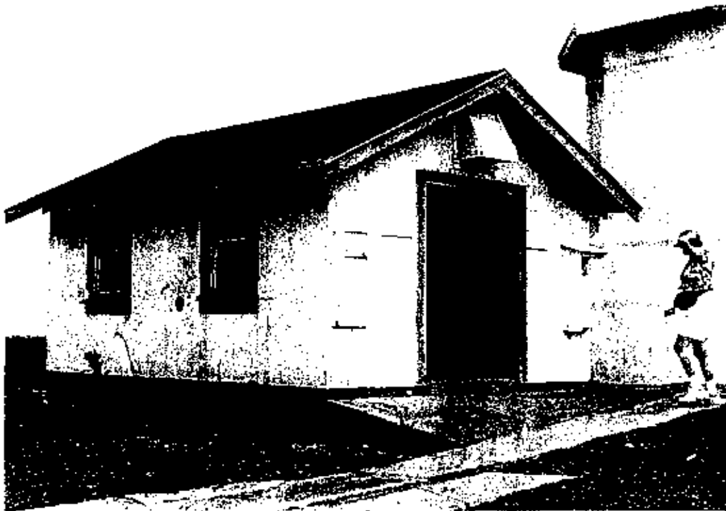
Figure 34. Wood-frame powerhouse (Feature 4), view from west, September, 1999. Photograph: William Chapman.
