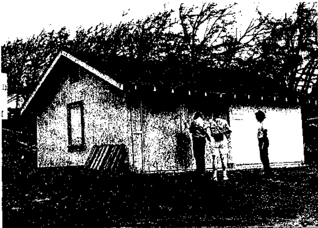
Figure 46. Wood-frame garage (Feature 10), from northwest, September, 1999. Photograph: William Chapman.
