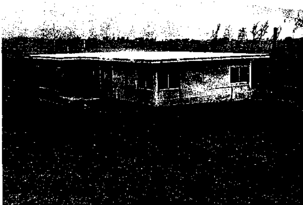
Figure 42. First Assistant Keeper's Residence, later Keeper's Residence (Feature 8), view from northeast, September, 1999. Photograph: William Chapman.
