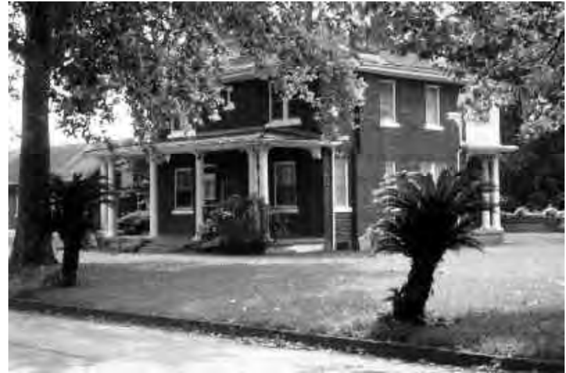
Figure 51. Cemetery lodge/park administrative headquarters viewed from northeast. Note foundation plantings and sago palms along drive [foreground].
