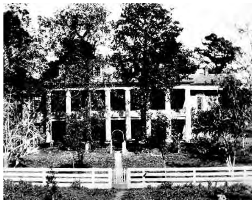
Figure 8 Malus-Beauregard House, riverfront facade and fenced yard with ornamental tree plantings, c. 1900. (#40-20-027)
