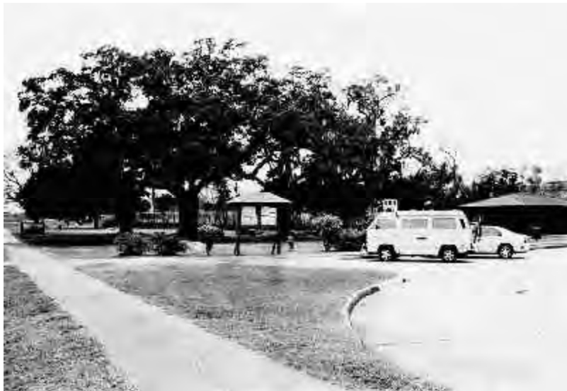
Figure 36. Comfort station and visitor parking area, showing wayside bulletin board, pedestrian paths, and ornamental shrub plantings.
