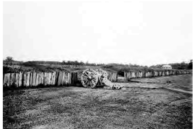
Figure 32. American rampart showing battery position at interpretive wayside.
