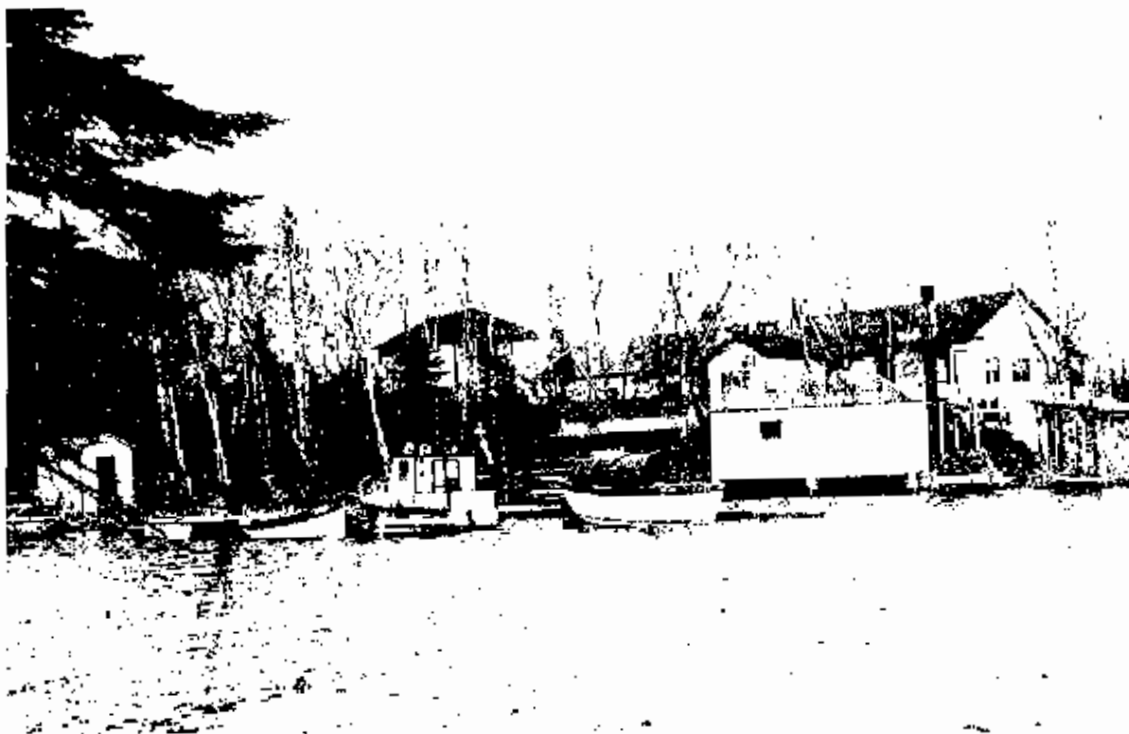
Fig. 6.49. View of the ledge and other service buildings looking southwest. Several small boats are tied up at the service dock. NPS photo by Donald Walbrink, 937.
