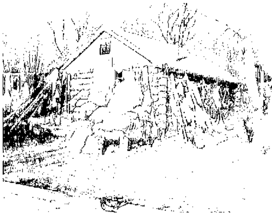
Fig. 6.19. The net house is constructed using simple and expedient saddle-notched logs, rather than elaborate corner notching techniques that typify traditional Scandinavian building. The use of logs, rather than milled lumber, is typical of first generation Swedish-Americans on the northshore. NPS photo by C. R. Humberger, 1949.
