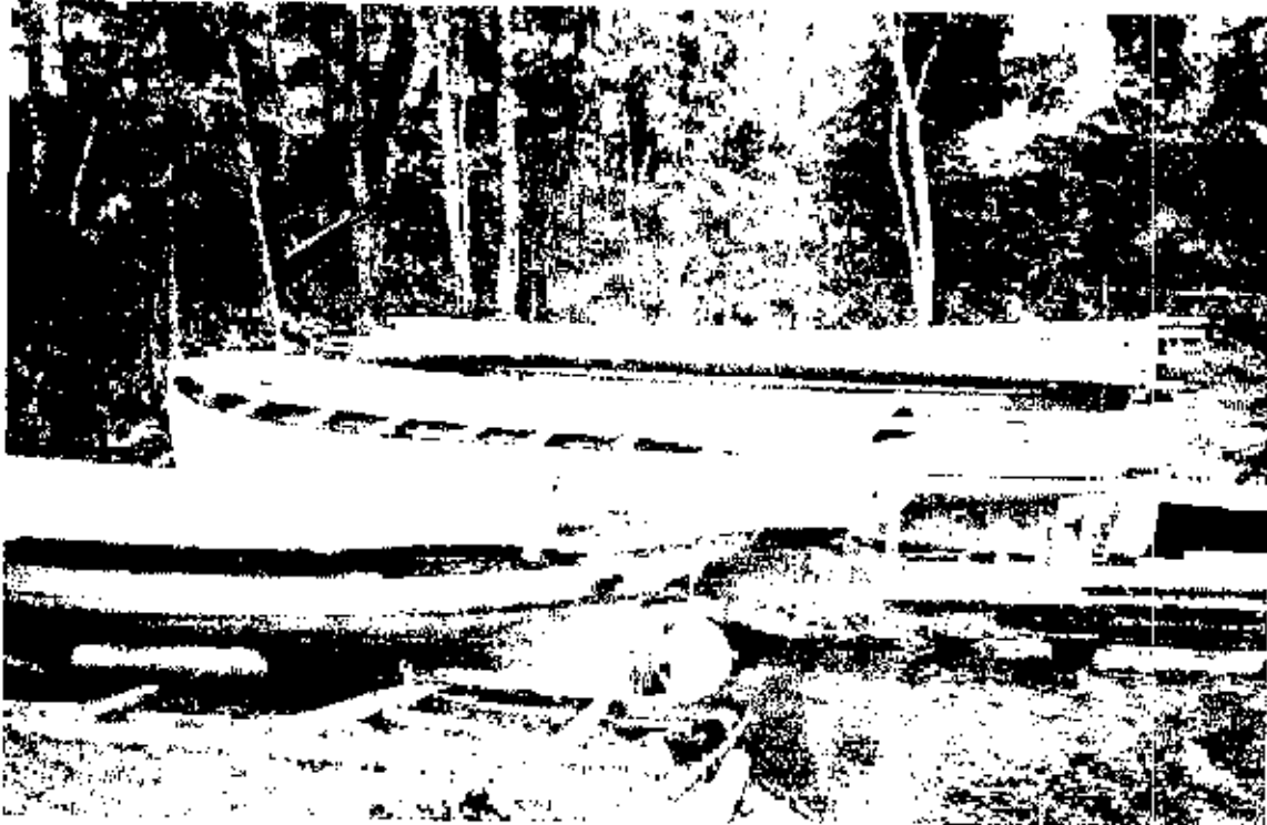
Fig. 6.72. By the 1930s the stern on both the launch and the gas boat took one of three forms, a fantail, a raked square stern, and a cut-away stern. The fantail and raked square stern were also seen on the larger fish tugs, the latter being the most common. NPS photo.
