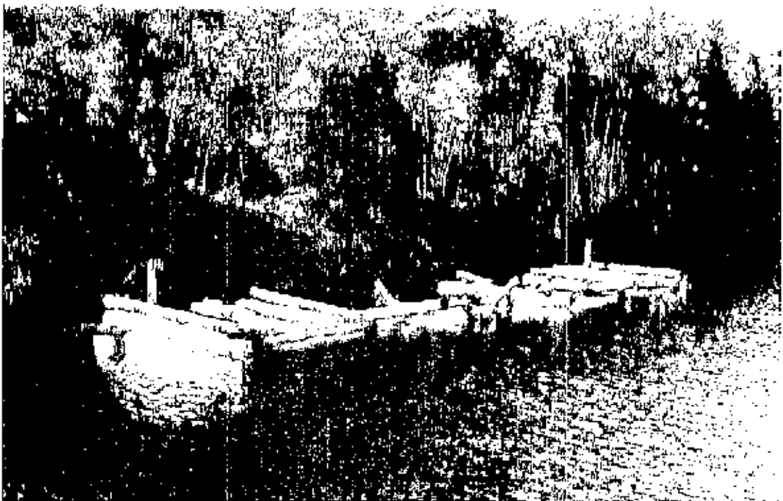
Fig. 6.30. The cribs associated with the wharf were still protruding above the water in the 1950s. NPS photo.
