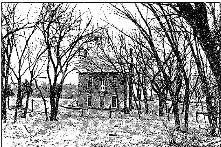
Figure 7. North elevation of Freeman's Brick House, early 1900's. [HNMA]
