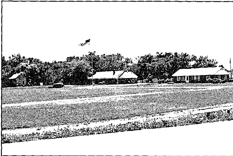
Figure 37. HNMA Headquarters area, 1957. [HNMA]
