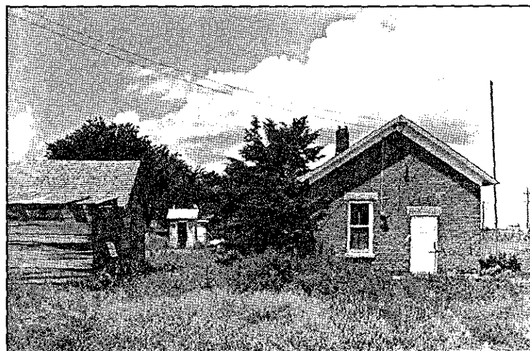
Figure 45. South elevation of Freeman Schoolhouse and outbuildings, 1958. [HNMA]
