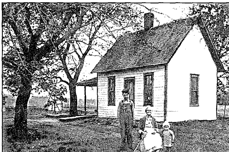
Figure 18. North and east elevations of Agnes Suiter Freeman Cabin, ca. 1925. [HNMA]
