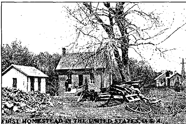
Figure 11. Freeman Brick House with Daniel Freeman in foreground, ca. 1903-1904. [HNMA]
