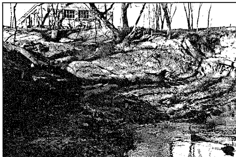
Figure 35. Cub Creek erosion south of utility building, 1951. [HNMA]
