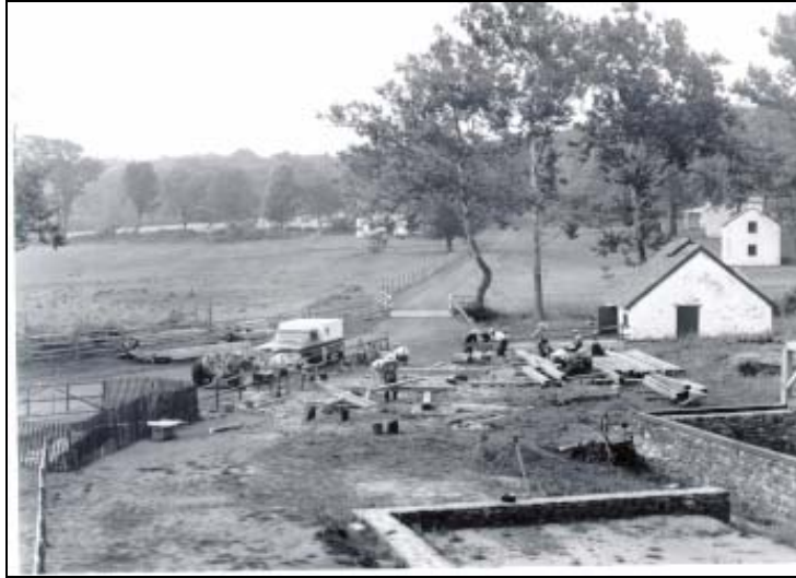
5.13 General View of Amish Workers Preparing Beams Prior to the Cast House Reconstruction, 1964. HOFU Photographic Archives.
