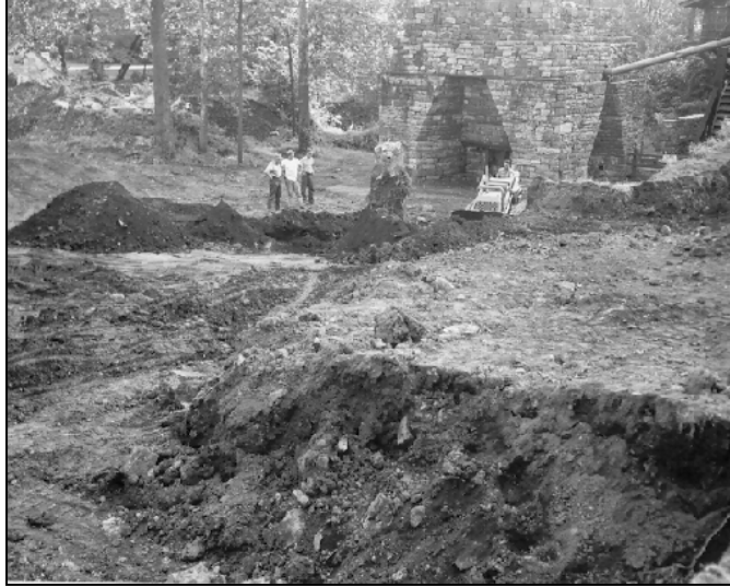
5.5 Excavating with a Front End Loader near the Furnace, 1955, HOFU Photographic Archives.
