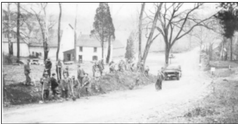
3.2 General View, North, CCC Grading Road Slopes, 1935. HOFU Photographic Archives.
