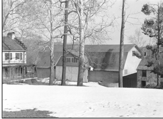
5.8 North View of Dairy Barn, Photo by Bob Ronsheim, 1958. HOFU Photographic Archives.
