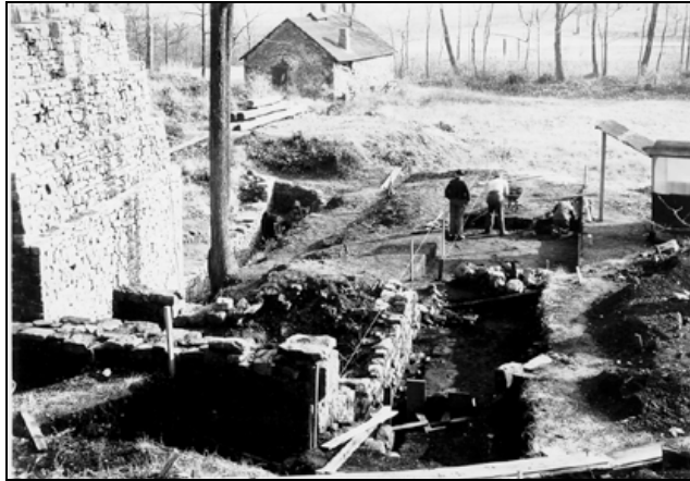
4.1 General View of the Wheel Pit Excavations from Furnace Bank, 1941. HOFU Photographic Archives.
