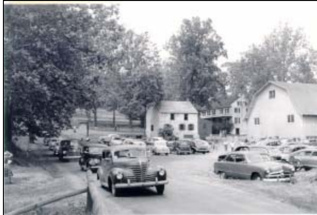
5.2 Cars and People in Village for Dedication of Waterwheel Ceremony, 1952, HOFU Photographic Archives.
