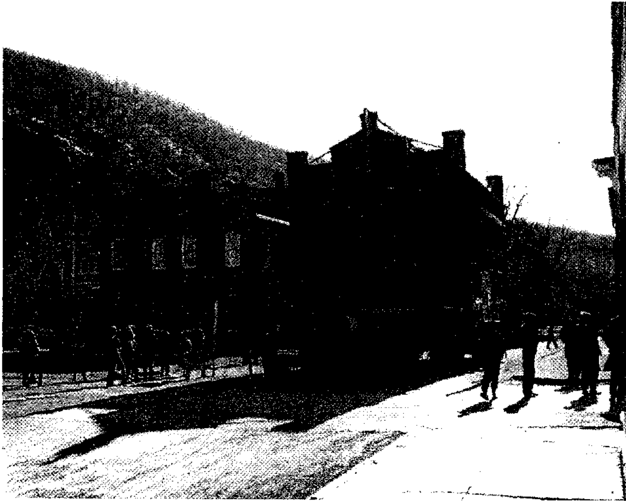
Fig. 19: John Brown Fort crossing intersection in Lower Town, 1968 (NHF-3152, Harpers Ferry NHP).
