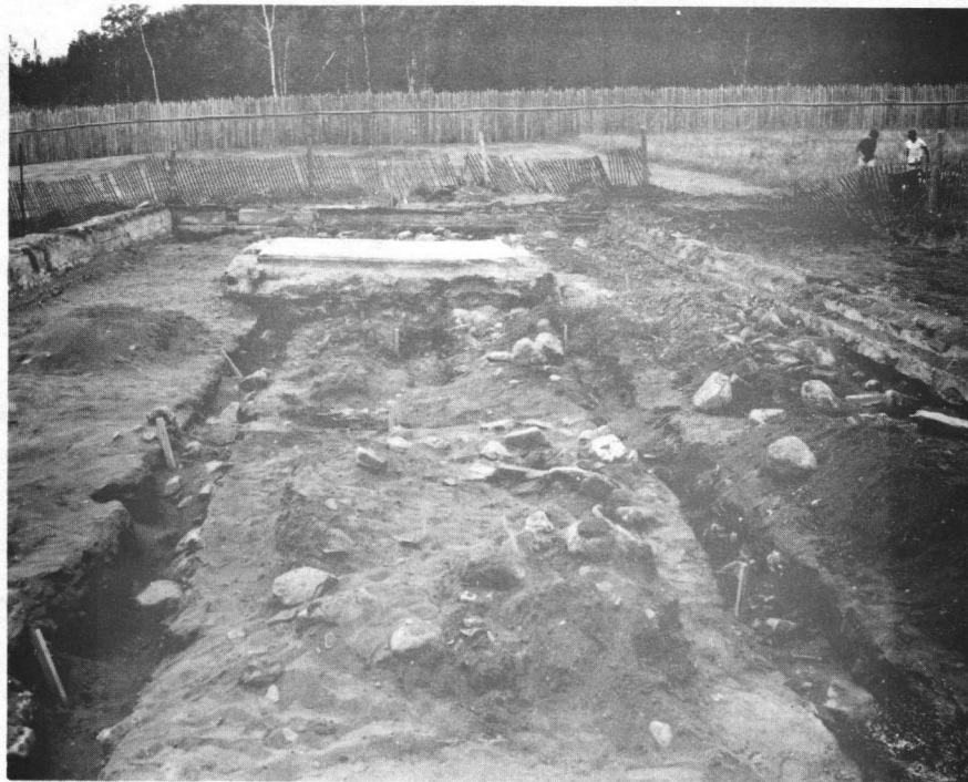
Figure 2: Exploratory trenches on the interior of the Great Hall Foundations. View is West.
