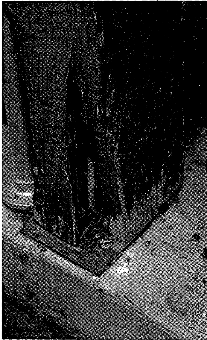
Figure 24. Tapered column at north elevation, shifted off steel base plate, a large split at bottom and exposure of the vertical steel dowel within the column. Damage caused by car. ARG Photo, dated May, 2000.
