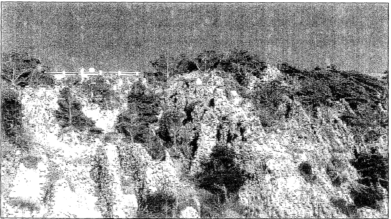
Figure 22: Cultural resource management at Golden Gate faces challenges not seen at other national parks. One of the park's responsibilities is maintaining Sutro Height's artificial rocks, built more than fifty years ago to hide walls that stabilize the cliff.
