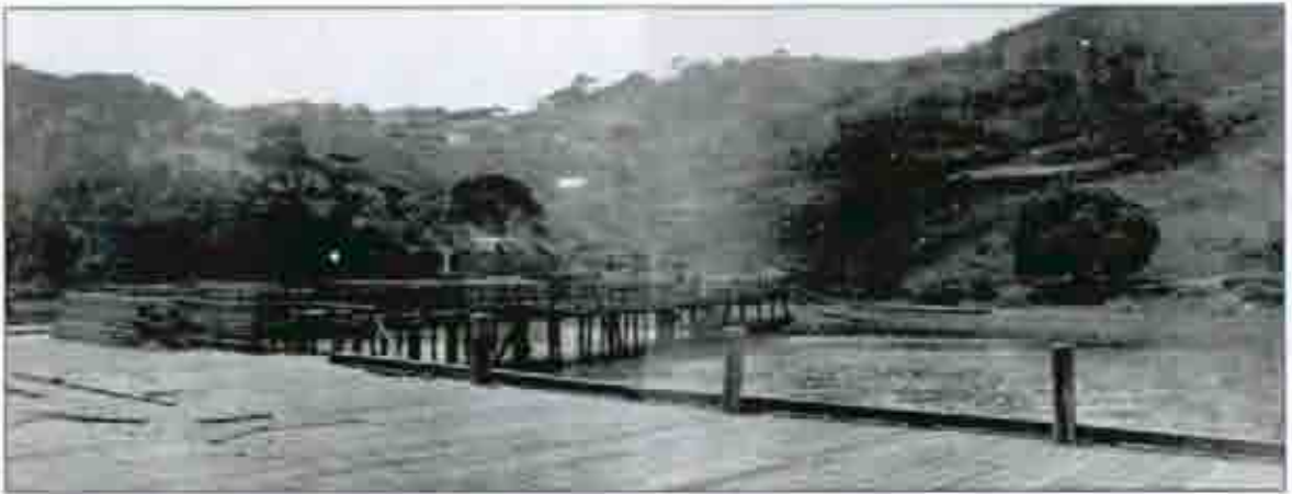
Figure 23. Damaged wharf, 1906 (CDPR Archives).
