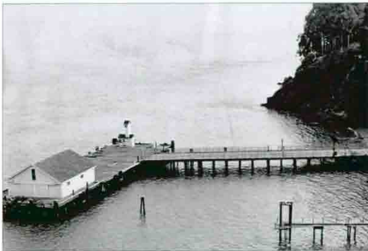
Figure 5.1. The wharf, 1950 (CDPR Archives).
