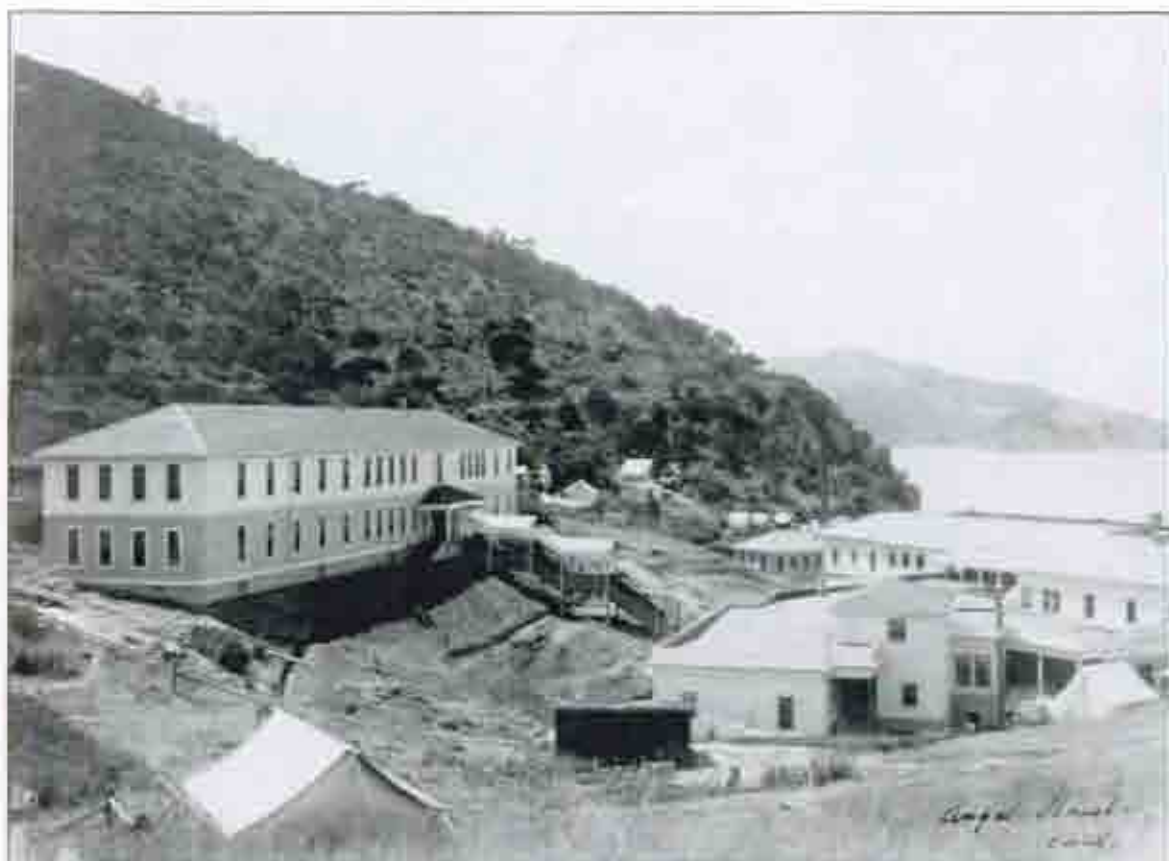
Figure 2.9. Newly constructed Detention Barracks and Administration Building, c.1908 (CDPR Archives).
