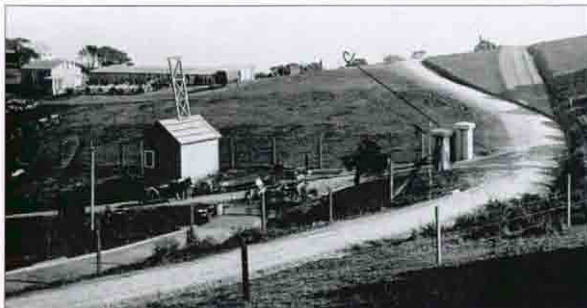
Figure 2.14. Entrance to Immigration Station from Perimeter Road, c.1910 (NARA/DC).
