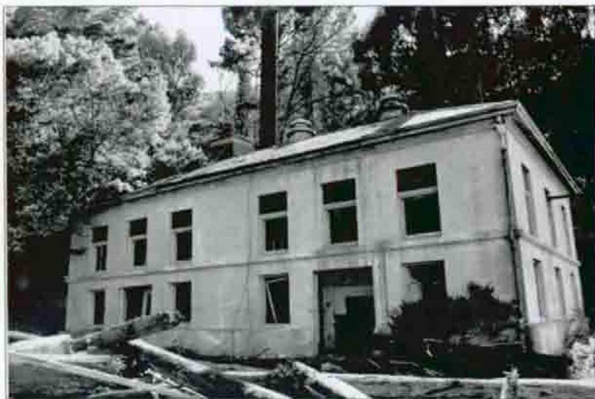
Figure 4.6. Neglected Power House, 1976 (CDPR Archives).
