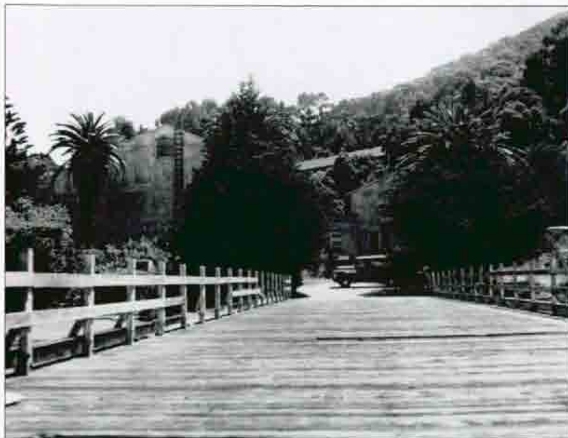
Figure 5.6. View of consolidated mess hall from the wharf, 1958 (CDPR Archives).
