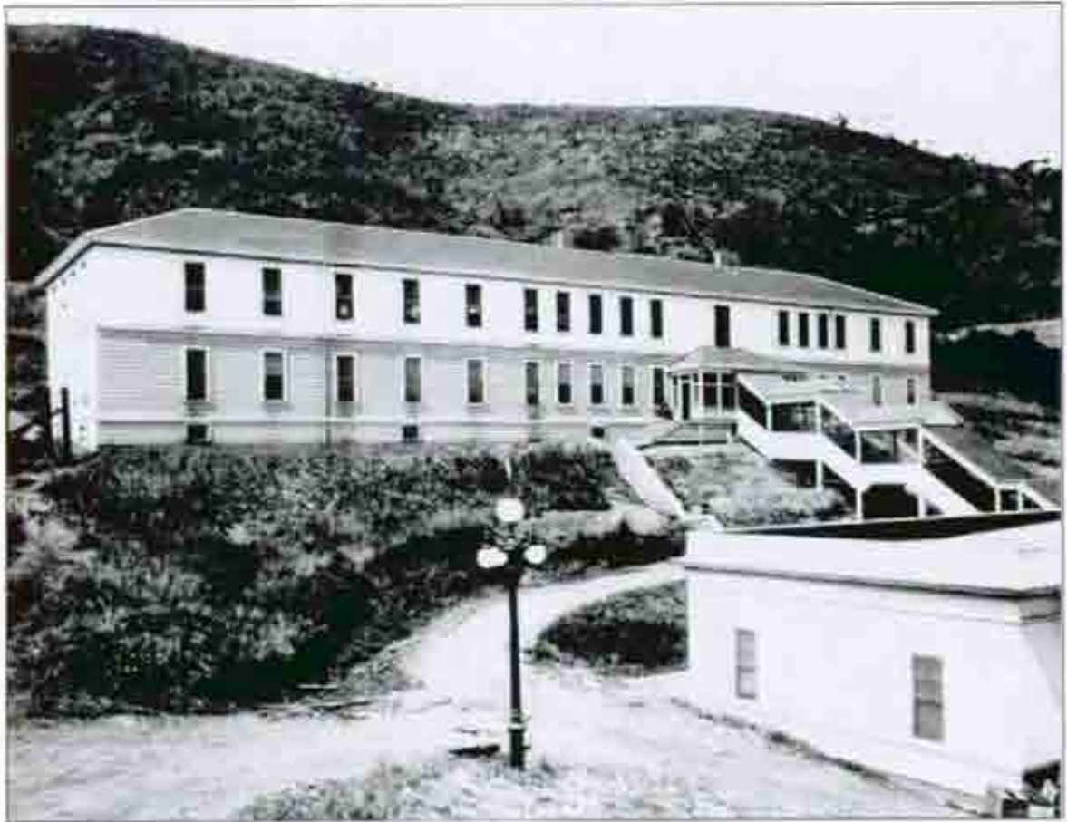
Figure 2.10. Completion of Detection Barracks and installation of lighting, c.1909 (CDPR Archives).
