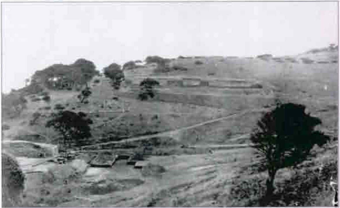
Figure 2.5. Excavation of foundations for Administration Building and Hospital, c.1907 (CDPR Archives).
