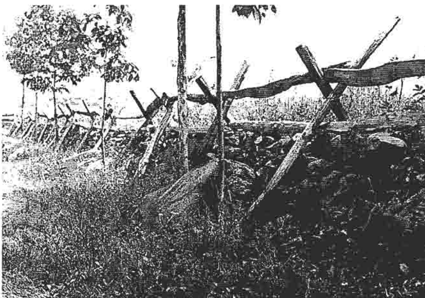
Figure 2-33 Stone and Rider fence. Normally, the rails forming the cross-braces were the same length and material as the rails that were used as the riders. (GNMP #23S-0006)
