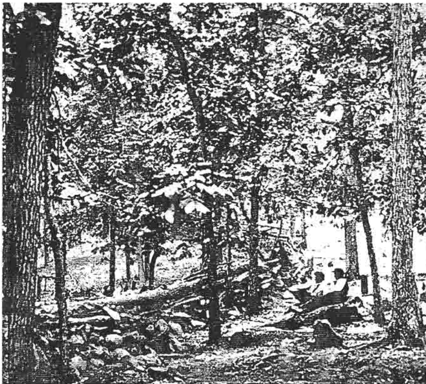
Figure 4-5 Union defense works on Culp's Hill (Mathew Brady, July 1863). These defense works were constructed by the Union 12 th Corps on the morning of July 2, 1863. Earth works defenses varied greatly in design and construction as soldiers used whatever materials and tools that were readily available. This section of works consists mostly of rocks and logs. Other Union defense works on Culp's Hill were made by felling trees and then digging a small trench along the inside, the dirt being thrown toward the front. Some even had head logs placed several inches above the main work, thus providing its defenders almost complete protection. (GNMP #2B-2115)
