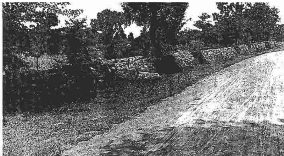
Figure 2-31 (below) shows a stone wall along Sedgwick Avenue (Wm. Tipton, ca. 1900-10). Although this wall was rebuilt by the War Department using contemporary standards, this photograph does provide a good example of the construction techniques used in 1863. These include tightly fitted stones, a wide solid foundation using larger stones and the top finished with capping stones. (GNMP#21P-2176)
