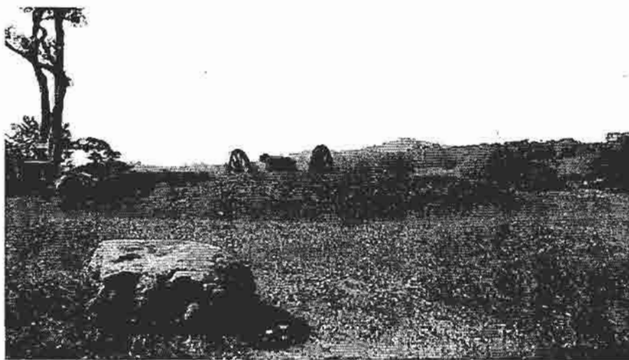
Figure 1-4 "Looking to Round-Top from Stevens' Battery," ca. 1898. View south/southwest from McKnight's Hill clearly reveals the excellent Observation and views from this location. Nearly the entire Union line, including the Round Tops (seen to the right of the cannon) could be seen from this location. (GNMP, Tipton #4272)
