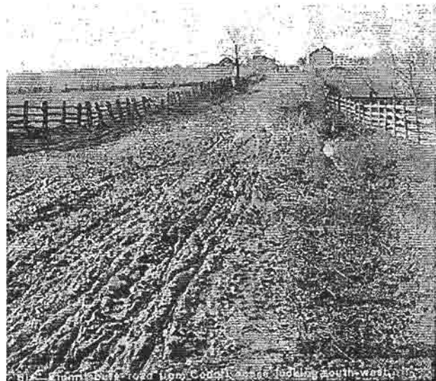
Figure 2-3 “Emmitsburg road from Codori house looking south-west,” (William Tipton, ca. 1888-1895). The poor condition of the Emmitsburg Road illustrates the result of the initial construction and lack of maintenance of county roads. This was especially true, as seen here, during times of inclement weather or heavy use. (GNMP, Tipton #1886)
