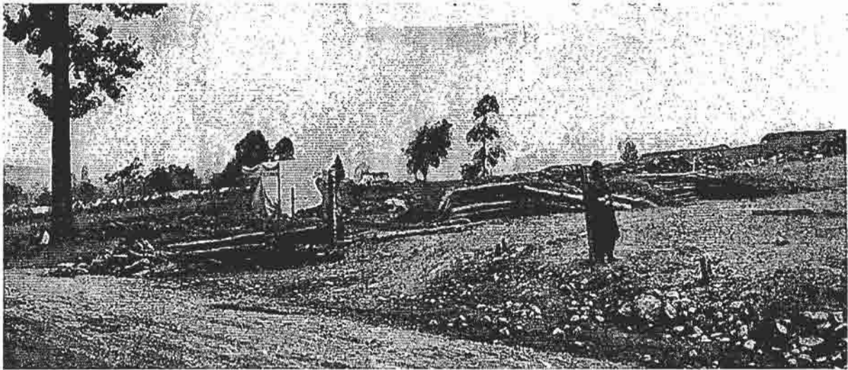
Figure 4-6 Union artillery lunettes on East Cemetery Hill, view north (Frederick Gutekunst, July 1863). These lunettes were constructed on the night of July 1, 1863 and protected the guns belonging to Lt. James Stewart's Battery B, 4 th U. S. Artillery. Note the use of rails from a dismantled fence on the inside of the lunettes. (GNMP #2B-2031)
