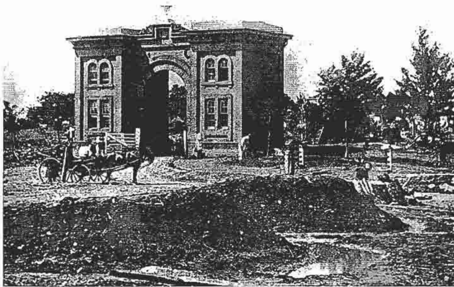
Figure 4-7 Evergreen Cemetery Gatehouse (Timothy O'Sullivan, July 1863). The artillery lunettes in foreground are the same as those shown in the previous photograph as seen from the front. (GNMP #2B-2027)
