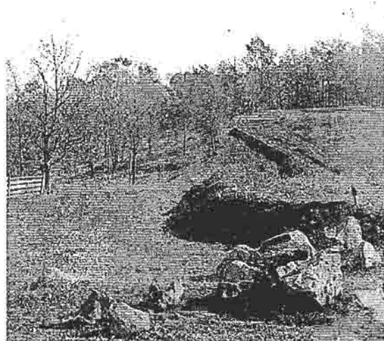
Figure 4-8 "Earthworks from Steven's Knoll to Culp's Hill (William Tipton, ca. 1888-1889). This view shows some of the earthworks on McKnight's Hill (Steven's Knoll) and Culp's Hill that had recently been reconstructed by the Gettysburg Battlefield Memorial Association. (GNMP, Tipton #1846)
