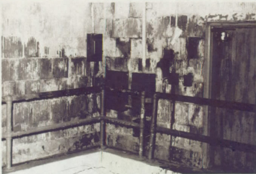
Northeast corner - typical wall and railing condition. June 1979
