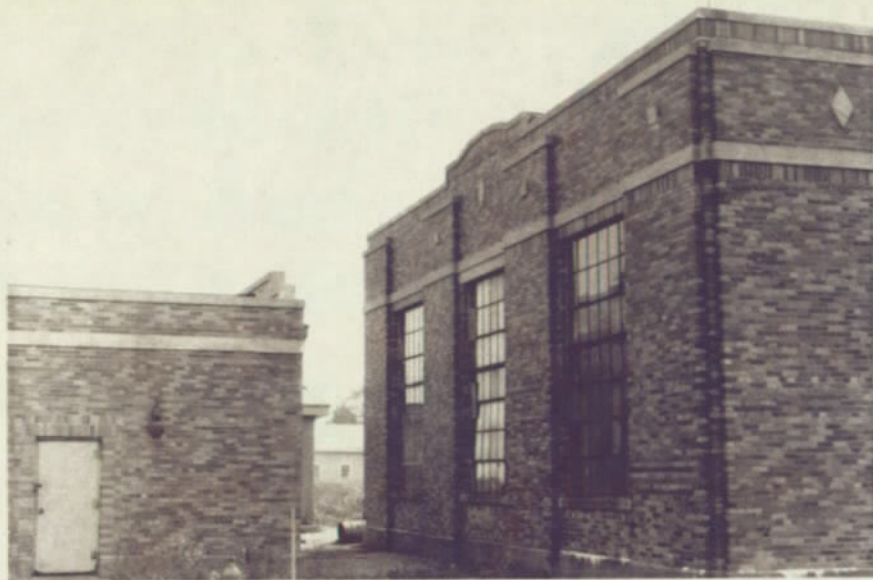
East Elevation - Note Pump House 30 to the left. October 1978
