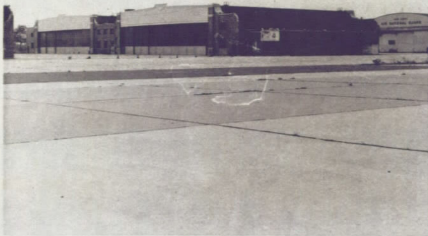
South Elevation - Hangar Complex 6 June 1979
