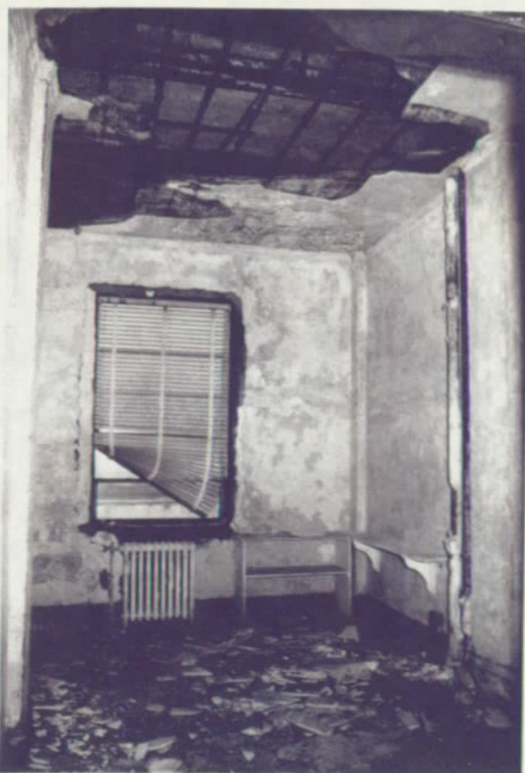
First-floor room at east side of building.
