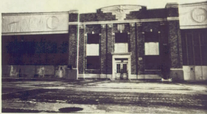
Decorative facade of infill's north elevation - note art deco cast stone panels and propellor January 1979
