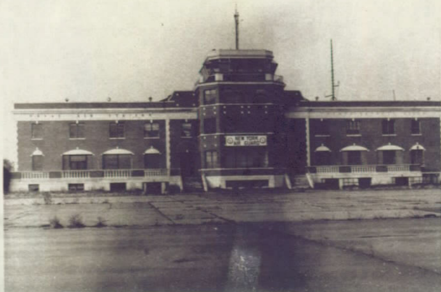
Administration Building - East Elevation, 1979 Note half circle ghosts above entry doors at either side of the tower where leaded glass canopies were attached.
