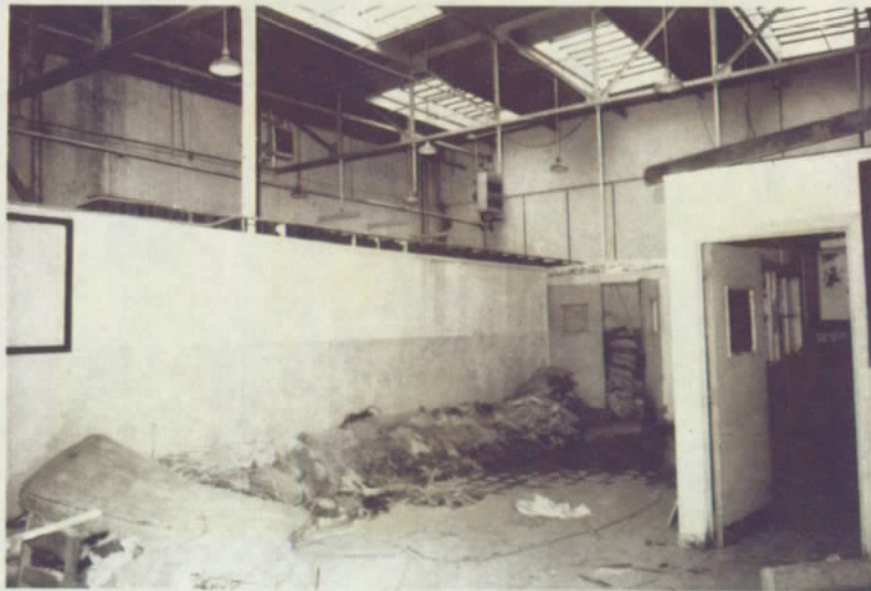
Interior WPA infill
