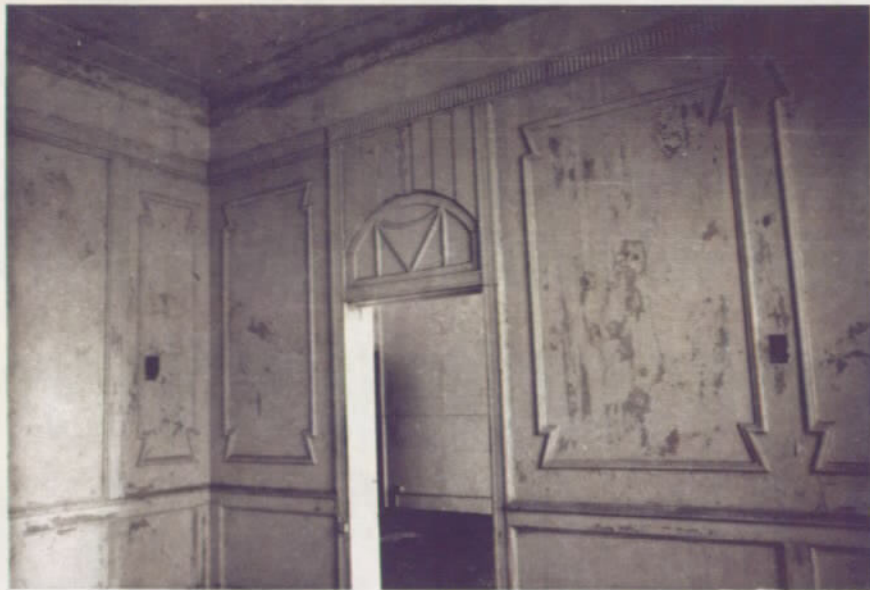
Interior of Women's Rest Room on First Floor. January 1979.
