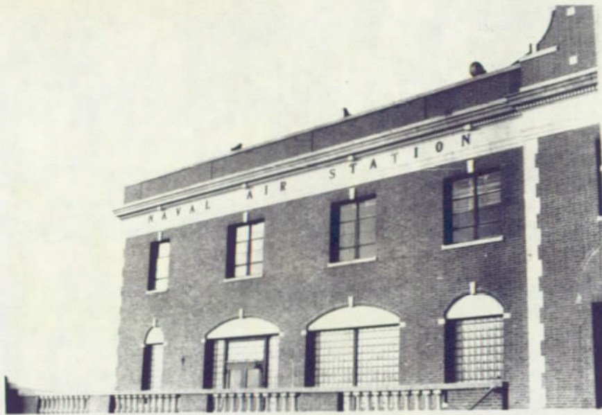
East Elevation at South End - Note later copper letters ("Naval Air Station") and glass block windows (Compare with Sheet 1 of Contract 2000 following). October 1978.
