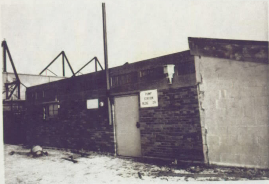
North Elevation. January 1979
