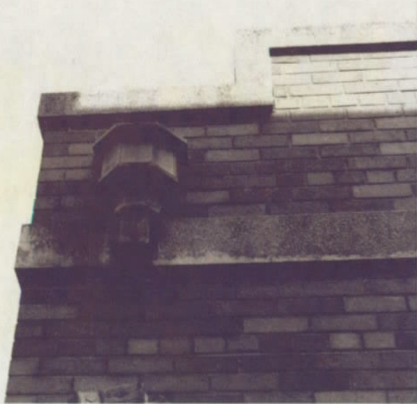
Northwest - scupper detail. October 1978
