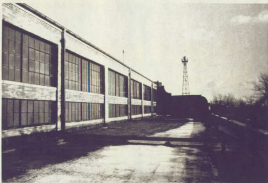
Roof of Hangar Complex 5, West Hangar Lean-to January 1979
