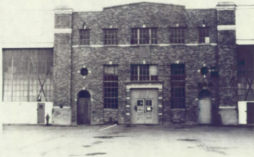
Hangar Complex 3 - WPA infill - North elevation October 1978.
