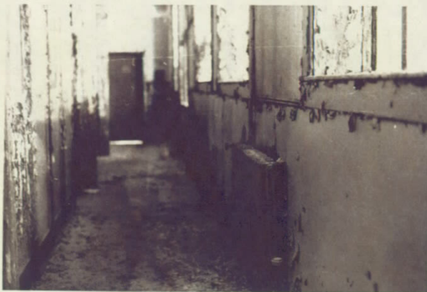
Typical condition at second story of East Hangar Lean-To January 1979
