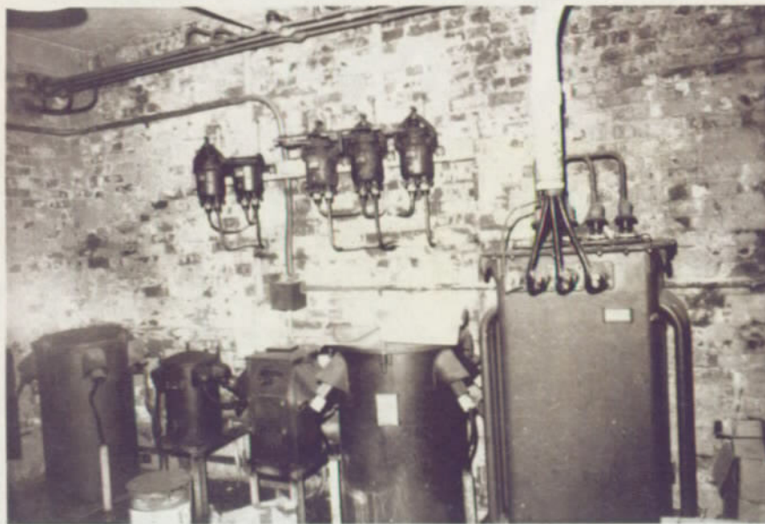
Typical interior wall - inside original wing.
