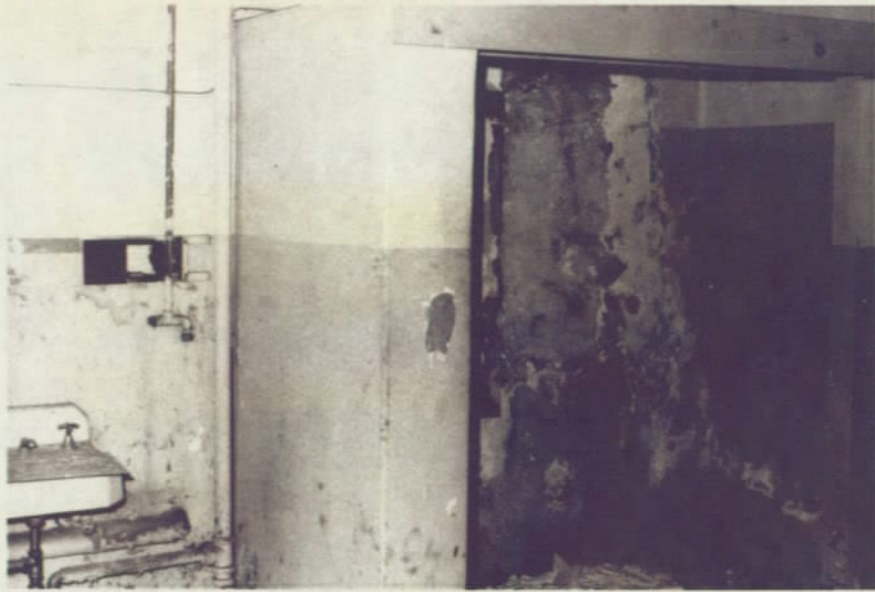
Hangar Complex 6 - Lean-to June 1979
