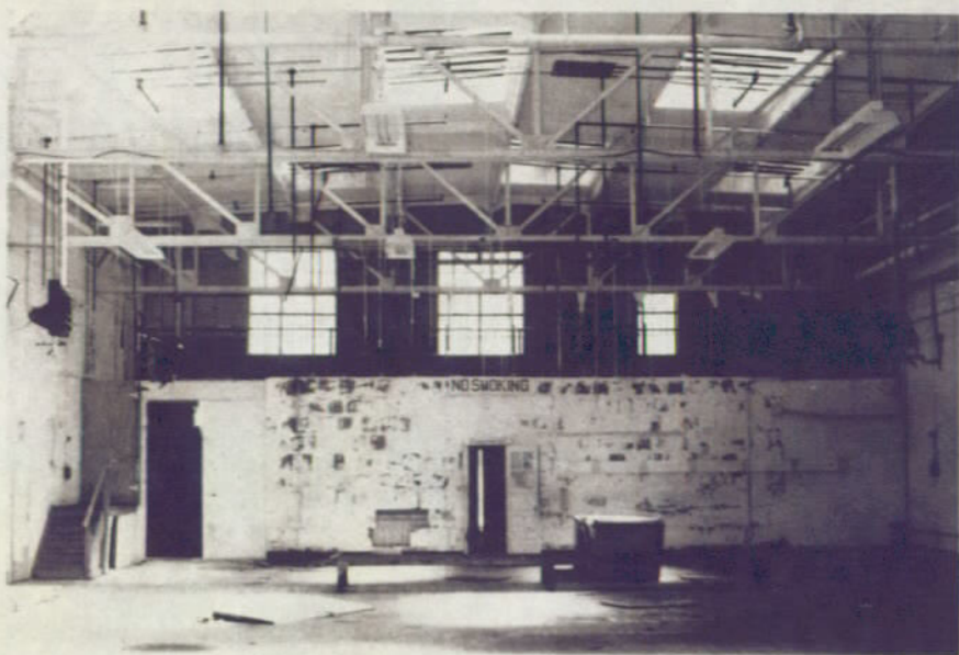
Interior WPA Infill, Hangar Complex 5 June 1979
