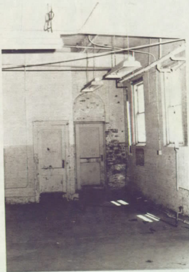
Hangar Complex 6 - Lean-to June 1979
