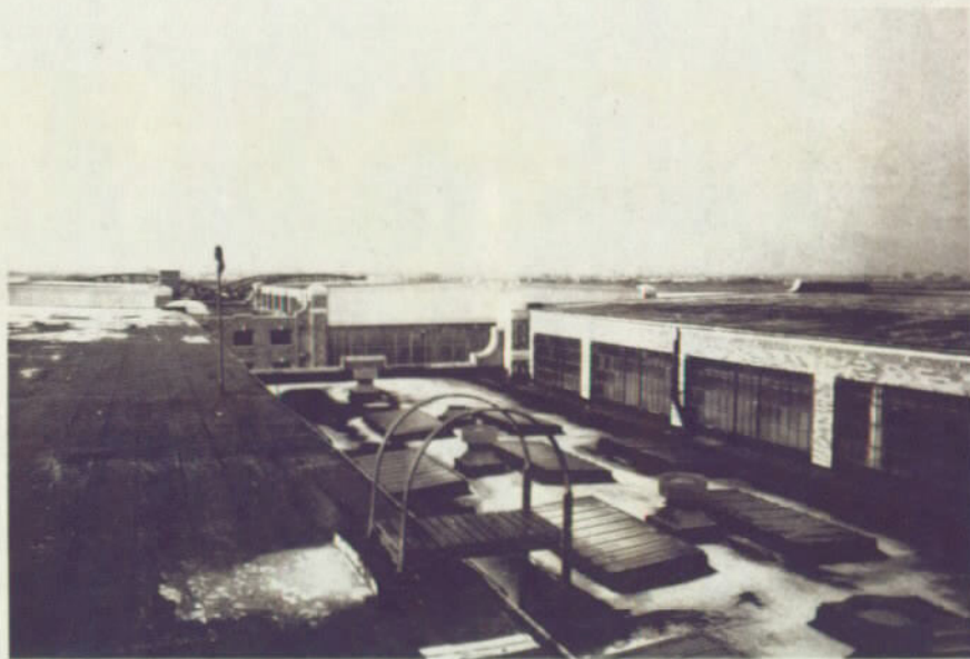
Roof of Hangar Complex 5, WPA Infill January 1979
