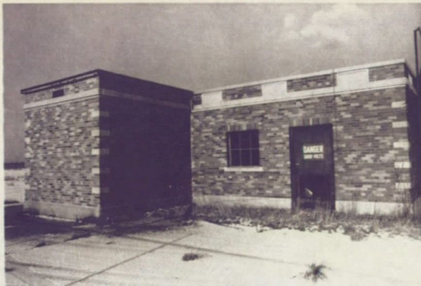
Southwest Elevation - Original wing at right and later wing at left. Note decorative cast stone panels at parapet of original wing. Quoins at the north end of this wing were obscured by the abutment of the south wall of the later wing. January 1979
