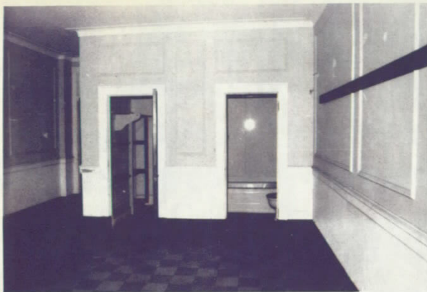
Second Floor - Typical bedroom
