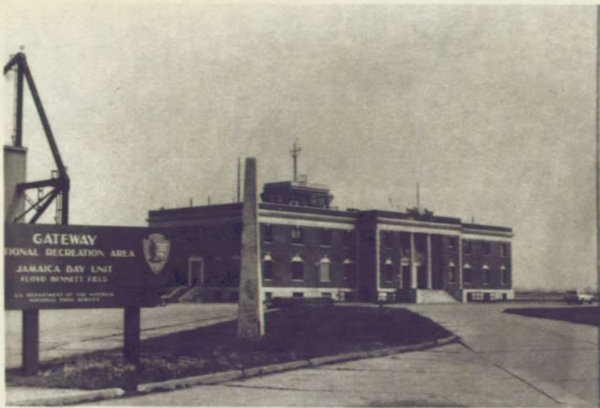
Administration Building - West Elevation, 1979
