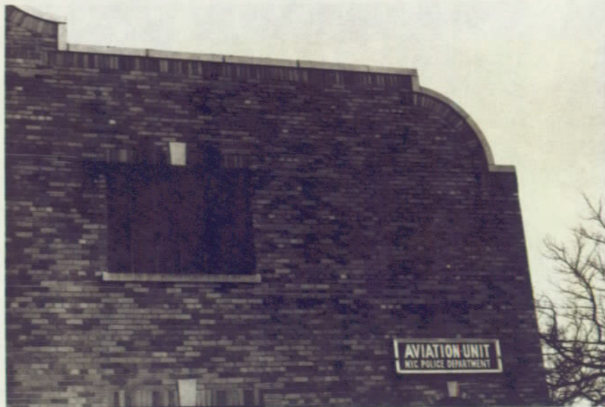
Northwest corner parapet - typical parapet condition. April 1979
