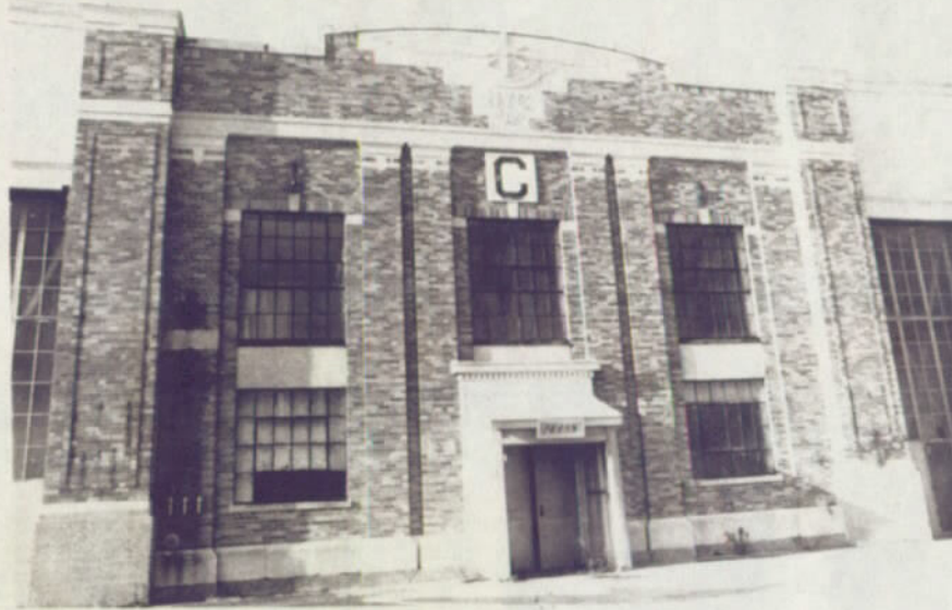
WPA Infill - South Elevation January 1979
