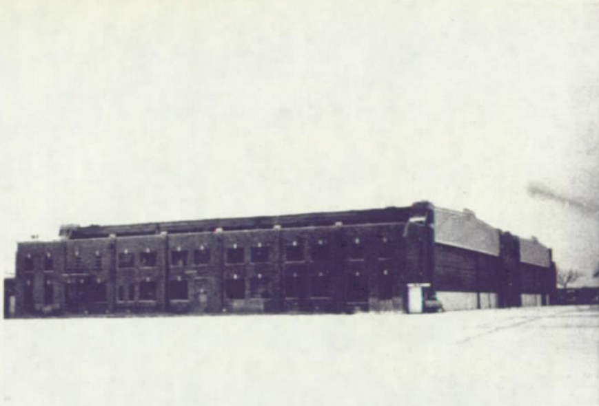
Hangar Complex 3 - Northeast elevation January 1979.
