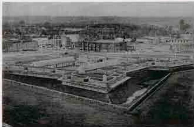
Fig. 17 This aerial view of the fort shows the Northern Bastion with sentry boxes and gun platforms. Inside the parade ground, the Park Service converted the West Barracks into two audio-visual rooms and a visitor contact hall; while the East Barracks provided space for living-history demonstrations. A museum in the East Casemate displays a series of the archaeological finds of the dig. The smaller brick house contained public restrooms. Courtesy of the National Park Service Historic Photograph Collection, Harpers Ferry Center, Maryland.
